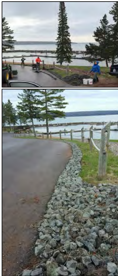
Initial riprap installed on April 25, 2017
