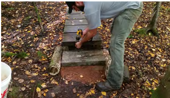
Figure 1: Replacing steps on a foot bridge
