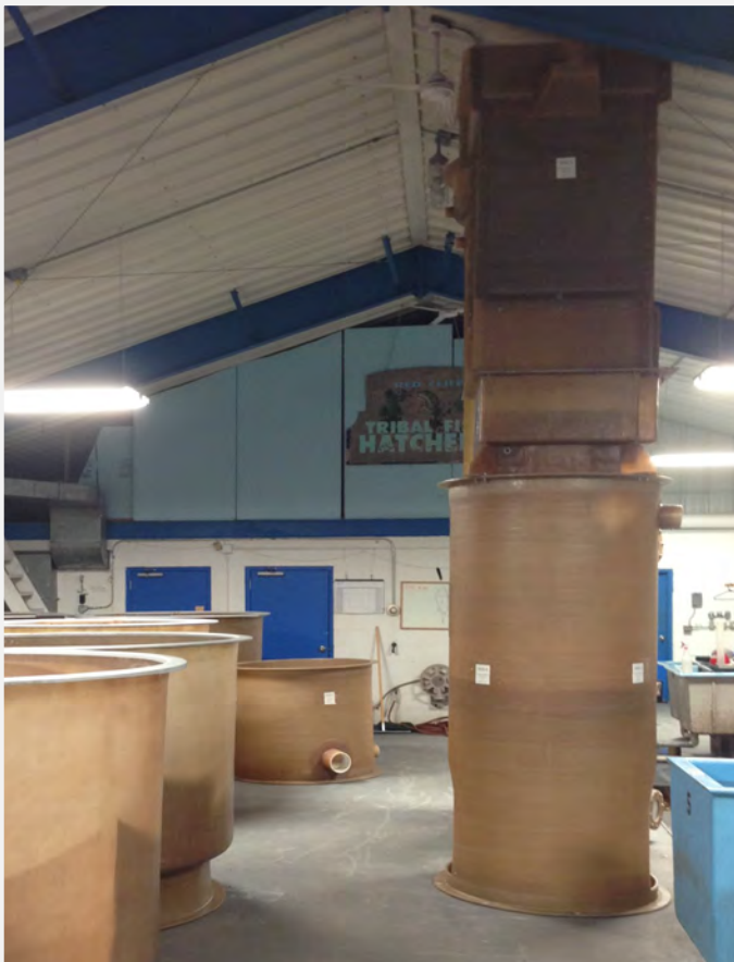
Pictured above: New tanks on left. On right is a 16 feet tall gas management tower and 16 feet tall sand bio-filter.
