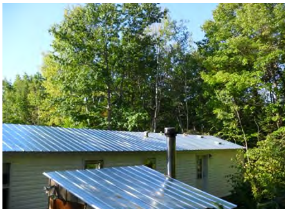
This trailer's roof and windows leaked. The owner has installed a metal roof with a 6-inch overhang to keep water out and away from home. Also note: the wood heater has been located outside to keep smoke, ash, and wood out of house for better indoor air quality. Check insurance considerations and build safely.
