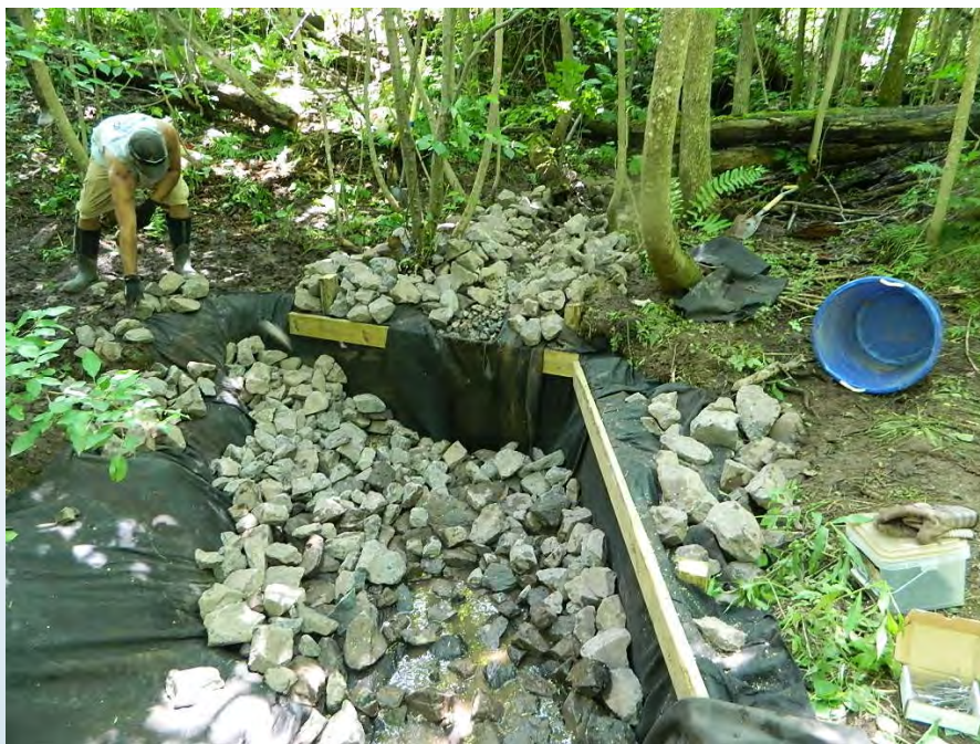
Below Photo: Restoration mid-project – the crew constructed what is called a toewall to stop the headcut.
