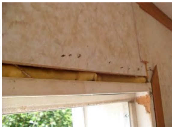
The gap around the door frame has been foam insulated by owner. Manufacturers often neglect to insulate windows, doors and hot water access.
