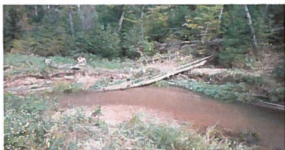
Brush bundle and log structure for bank stabilization.
