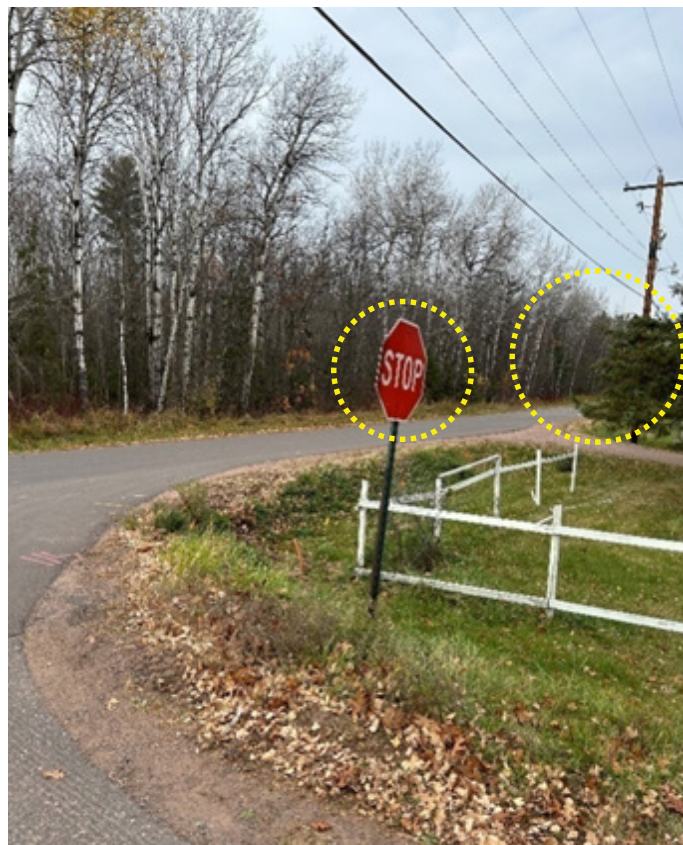
Figure 13 | | Example of Obstructions in the Line of Sight at Blueberry Road and Bishop Lane (Widseth)
