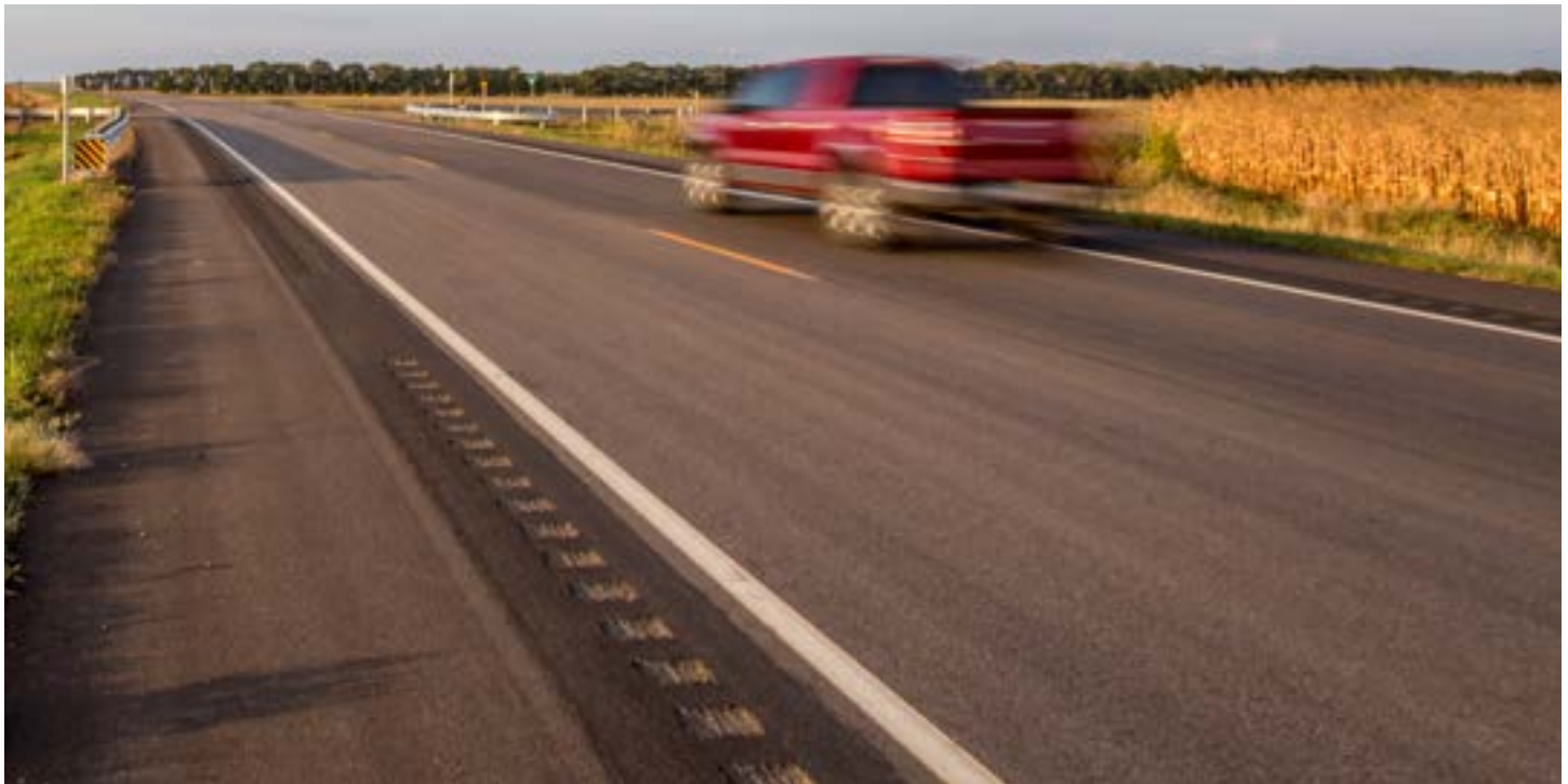
Figure 26 | Rumble strips along Highway 75 near Halstad, MN (Widseth)
