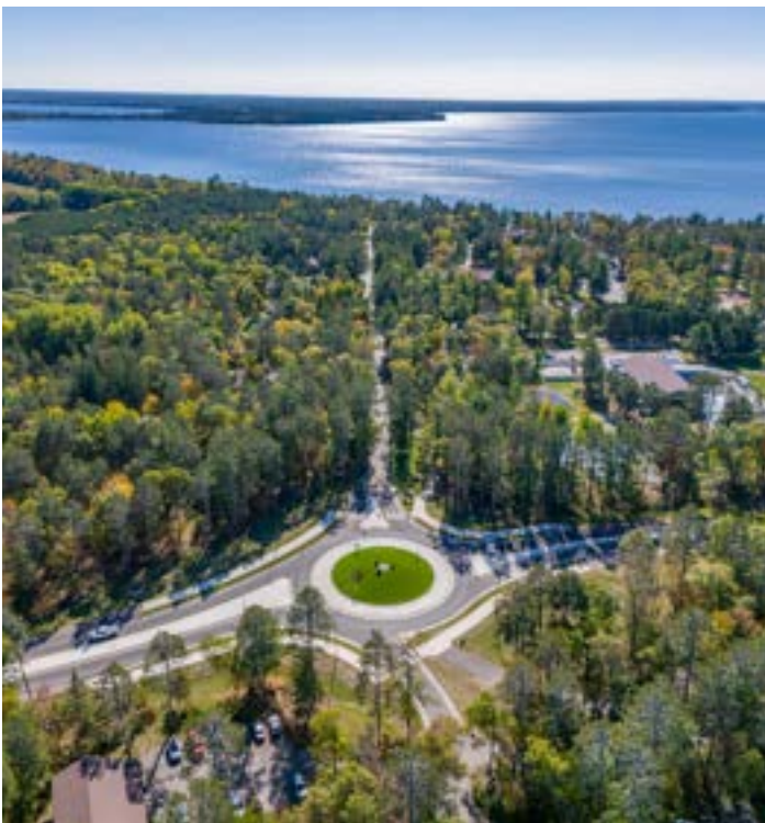
Figure 29 | Aerial view of County Highway 77 Roundabout, Nisswa, MN (Widseth)
