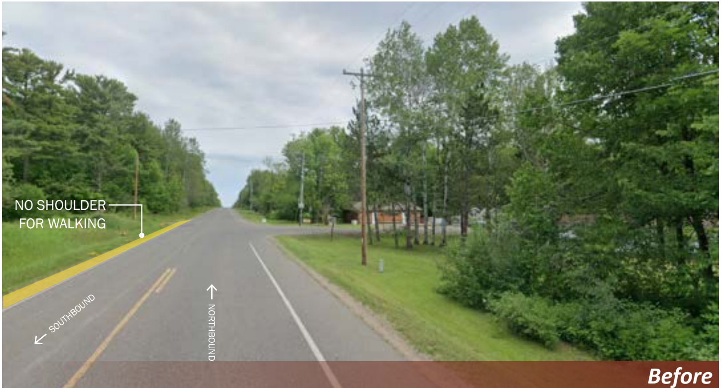
Figure 52 | Blueberry Road currently has narrow shoulders bordered by steep, vegetated slopes on both sides. As a result, pedestrians and cyclists are forced to share the roadway with fast-moving vehicles, creating a hazardous situation. (Terra Soma)
