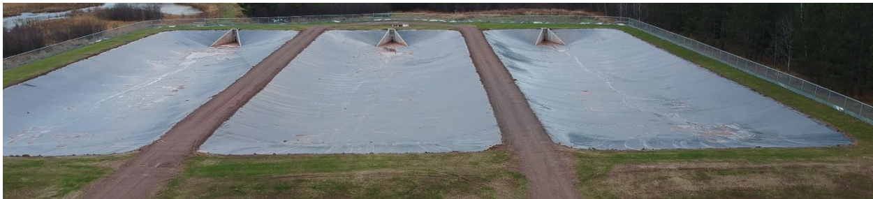
Three newly constructed walleye rearing ponds. Construction completed in 2018.
