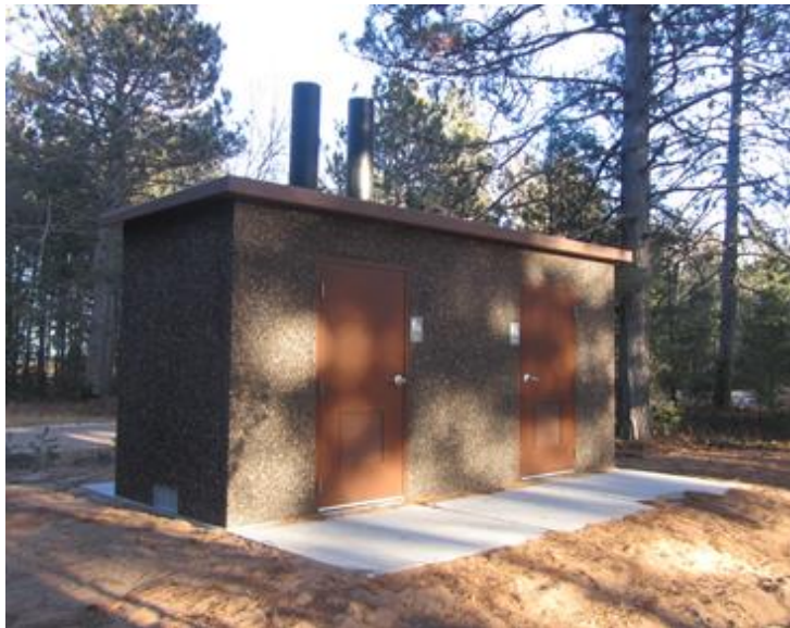
Latrine installed at Raspberry Bay Tribal Campground.
