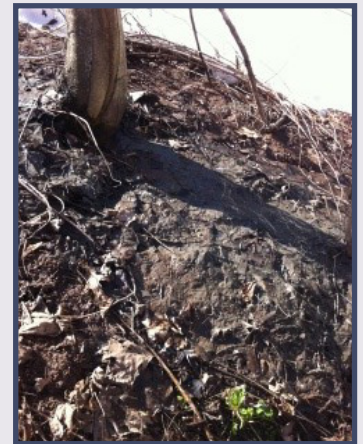
Septic system leakage
