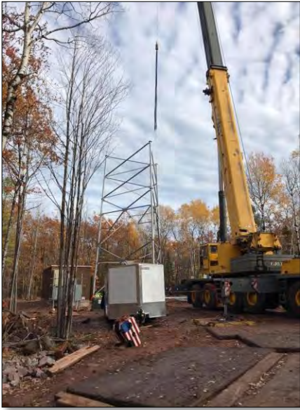
Wireless Cellular Tower Installation, October 2019
