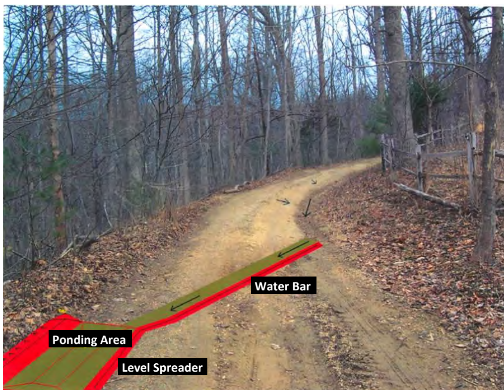
Possible Solution: Re-grade the roadbed with a crown, apply proper roadbed materials (gravel base), and install side ditches or rock check dams.
