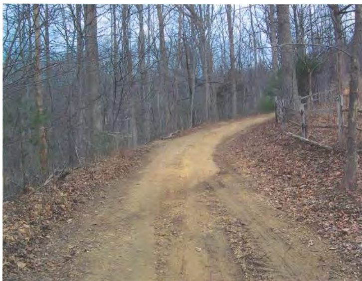
A poorly shaped road section that allows runoff to flow down the road bed.
