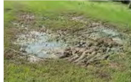
Sewage overflow due to failed septic system.
