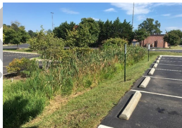
Figure 5-7. Bioswale to catch runoff from parking lot, Marshall, Virginia (September 2016).
