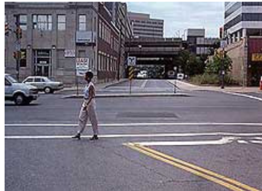
Median Barrier in Montgomery County, MD: barrier allows left turns out of the side street by use of a short barrier.
