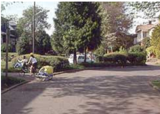
Diagonal Diverter in Boulder, CO: uses a wide landscaped closure with raised contour and paved pedestrian/bicycle walkway to connect both sides.
