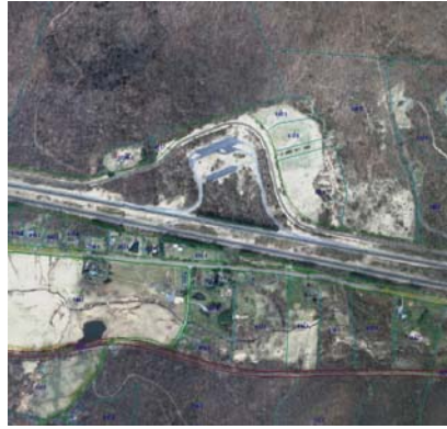
Markham Truck Rest Area
