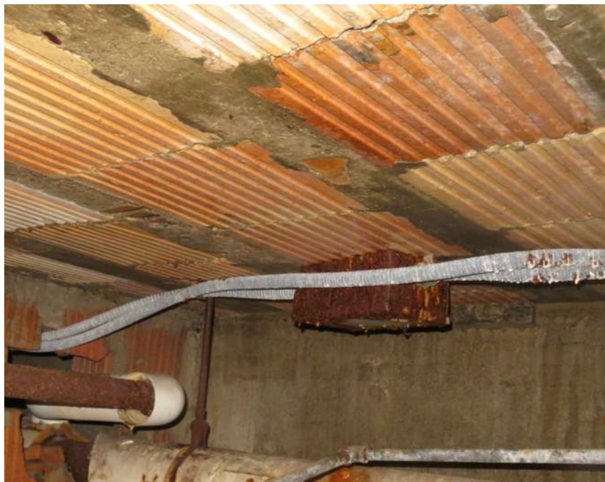
Photo 16: First Floor One-Way Clay Tile Framing in Main Wing
