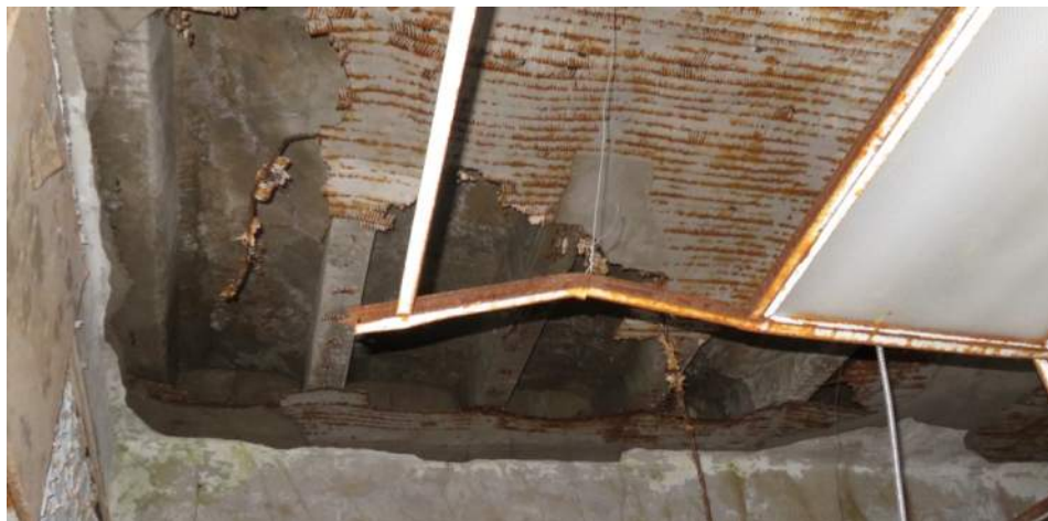
Photo 17: Second Floor Ribbed Slab Construction
