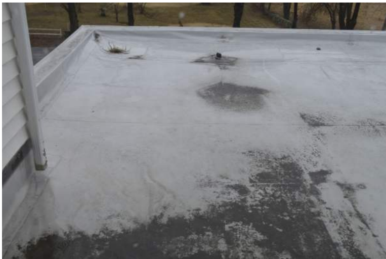
Photo 30: Ponding water exerts unintended forces on the roof structure, promotes growth of algae and plant materials which harm the integrity of the membrane, and infiltrates compromised flashing joints.
