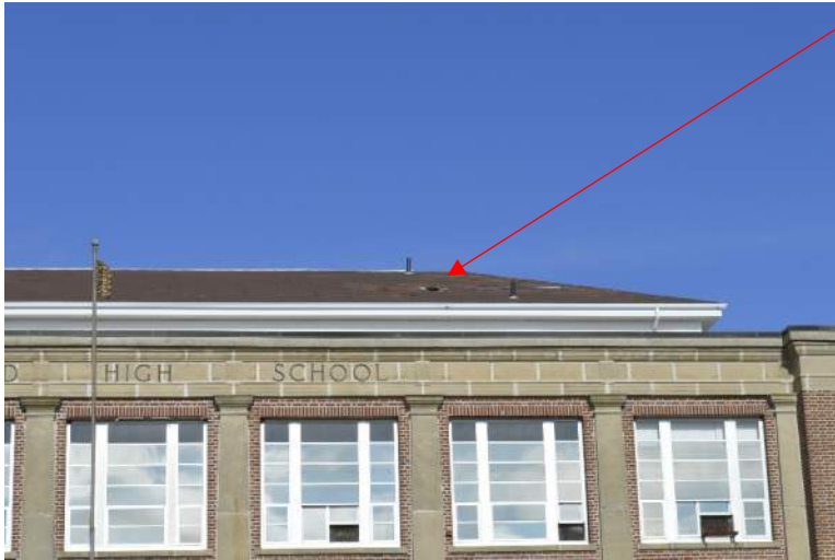
Photo 29: The asphalt shingles on the hipped roof third floor have served beyond their useful life.
