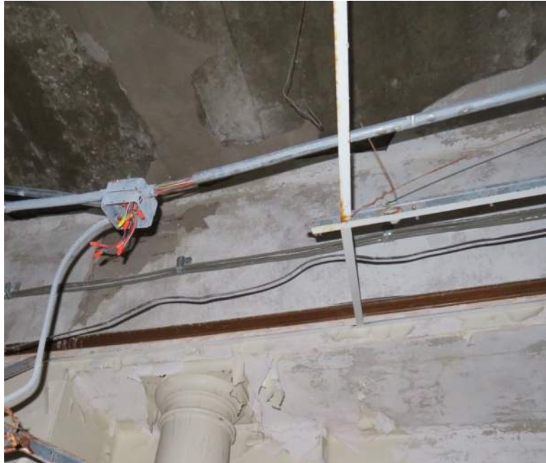
Photo 18: Second Floor Concrete One-Way Slab Construction in Corridor
