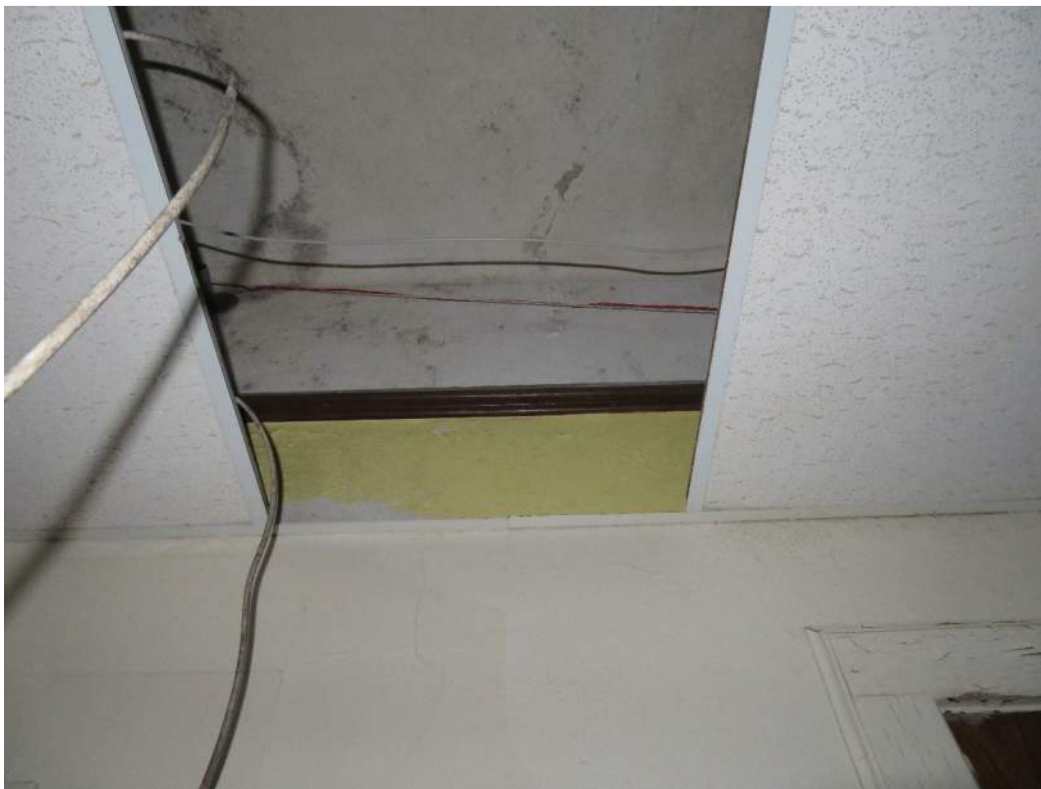
Photo 15: Picture rail molding has been concealed above the dropped ceiling. The height of the original ceiling in the hallway once provided a sense of the monumental building. This wood trim is one of few interior details in the old school.
