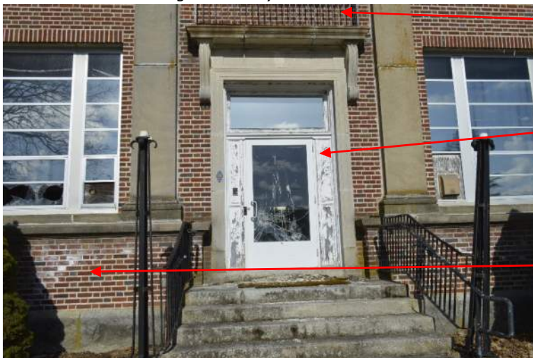
Photo 28: Originally the front entrance consisted of a pair of French doors filling the entire opening below the transom. Given building code requirements, a single wider door was added, flanked by side panels.
