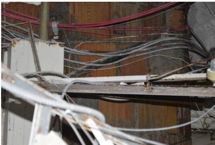
Photo 34: All power, life safety and lighting systems should be removed and replaced.
