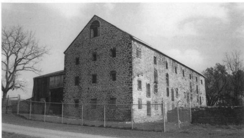
Figure 24. Once mothballed, a property must still be monitored and maintained. The openings in this historic barn has been modified with a combination of wood louvers and metal mesh panels which require little maintenance. The grounds are regularly mowed, even inside the chain link security fence. Photo: Williamsport Preservation Training Center, NPS.
