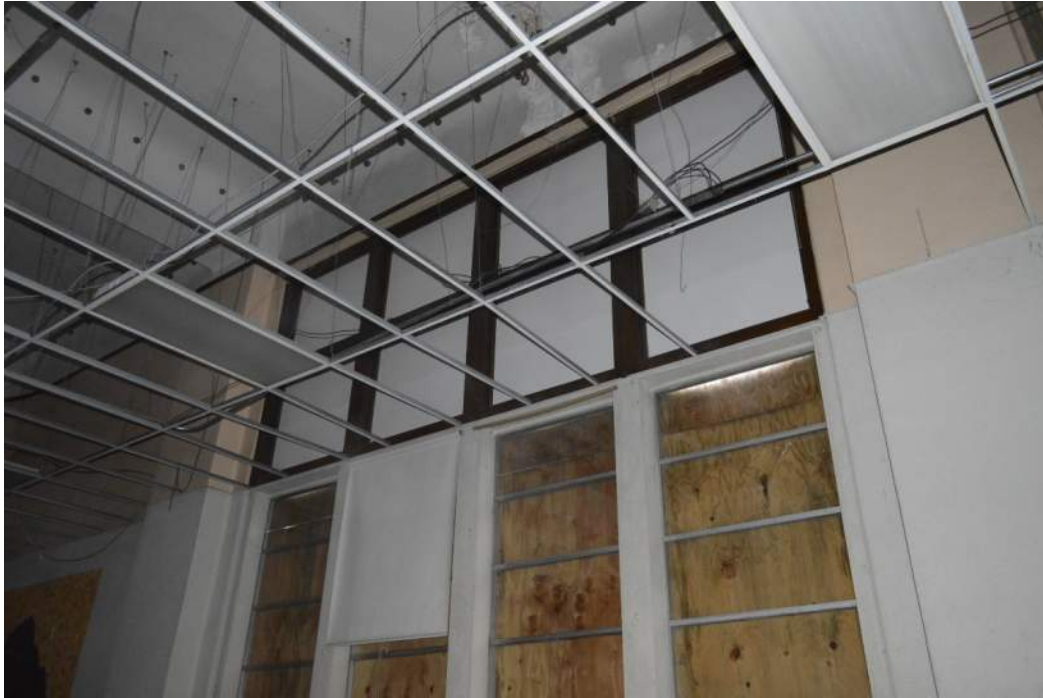
Photo 10: The two-story Auditorium features a coffered ceiling with rows of electric lights around each coffer. Transom windows above the first-floor windows retain the original stained wood finish. The height of the space, the special ceiling treatment and the windows should be retained as they provide unique character to this space. Partitioned spaces within the room should be removed.
