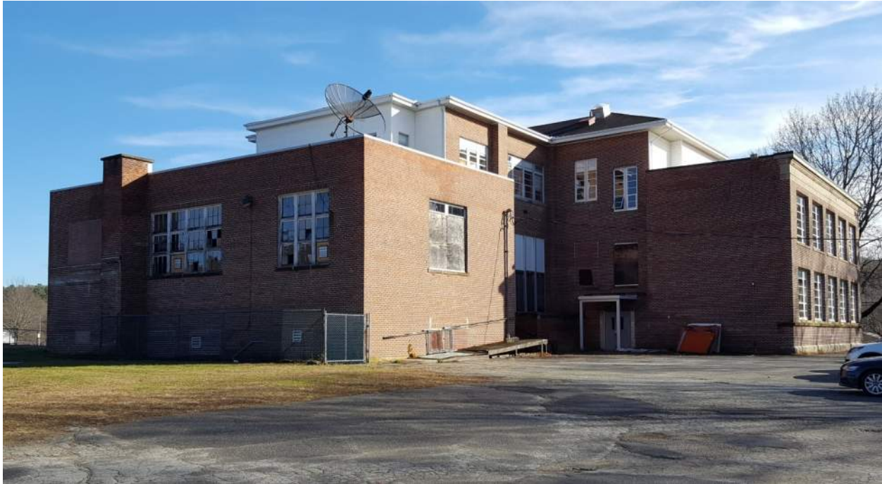
Photo 6: A view of the rear of the building looking northeast at the former gymnasium block on the left.
