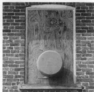
c. The exhaust fan has tamper-proof housing.
