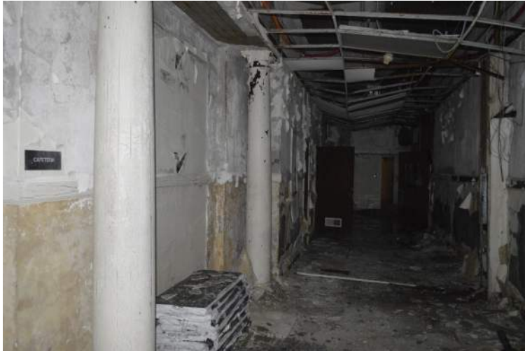
Photo 32: Floor, wall and ceiling finishes will need to be replaced.
