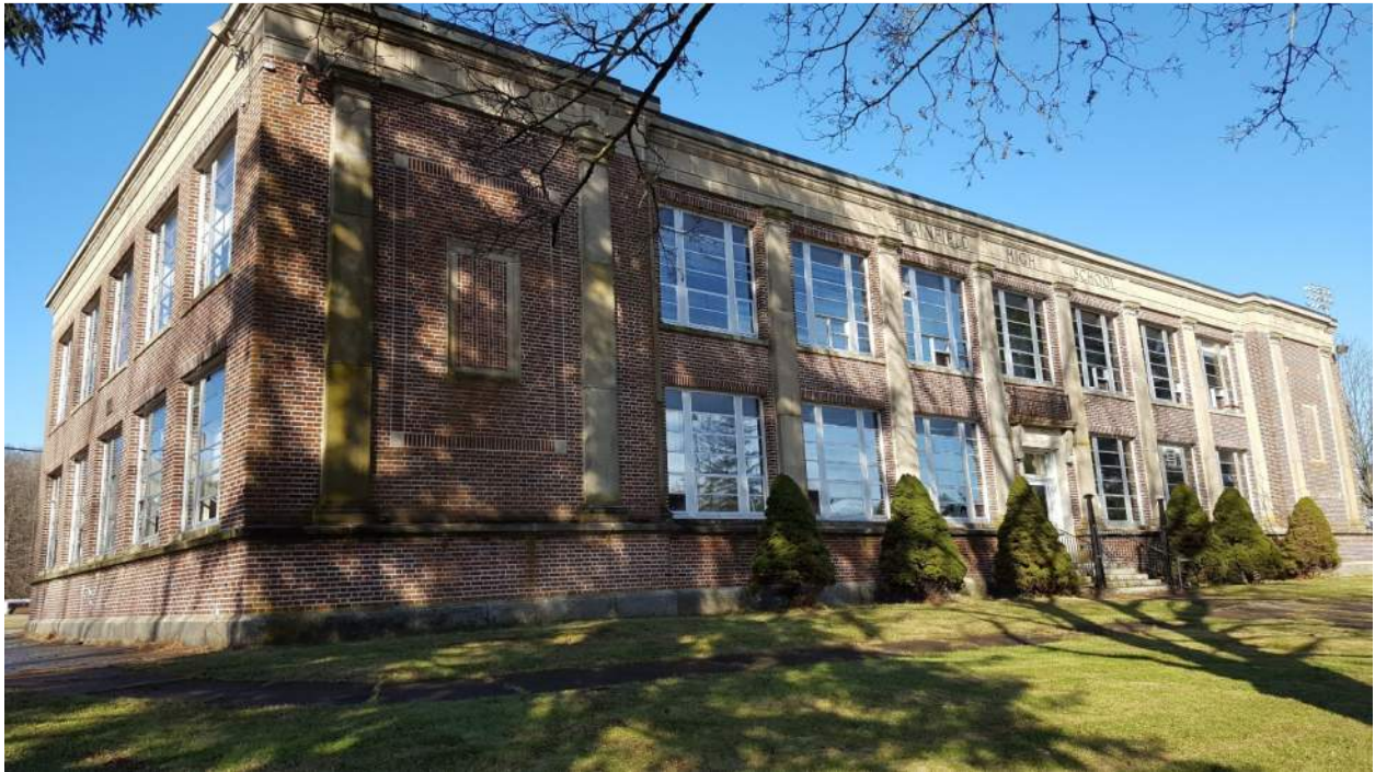
Photo 5: The east facing front façade in 2018.
