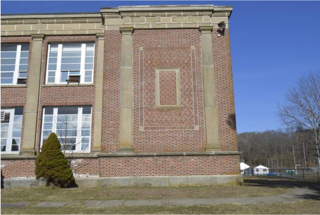
Photo 8: Character defining features of the façade include the red brick laid in Flemish Bond, decorative brick panels in the end pavilions, cast concrete two-story pilasters, cast concrete frieze and plinth base, granite foundation blocks and large window openings.
