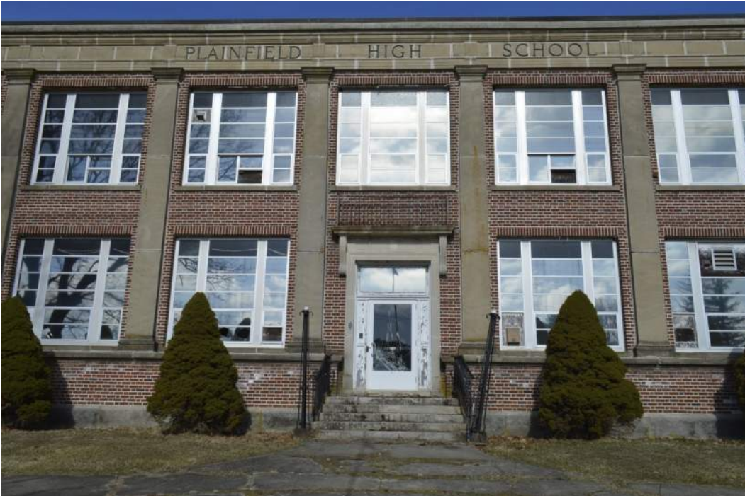
Photo 9: The main entrance approach, steps, railings, lamps, door surround, bracketed canopy with cast iron railing, and Plainfield High School bronze signage are all character defining features that should be retained.
