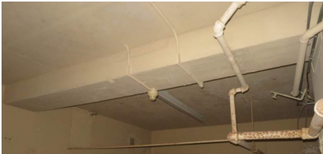
Photo 19: First Floor Ribbed Slab and Beam Construction with Finishes below Gym/Stage
