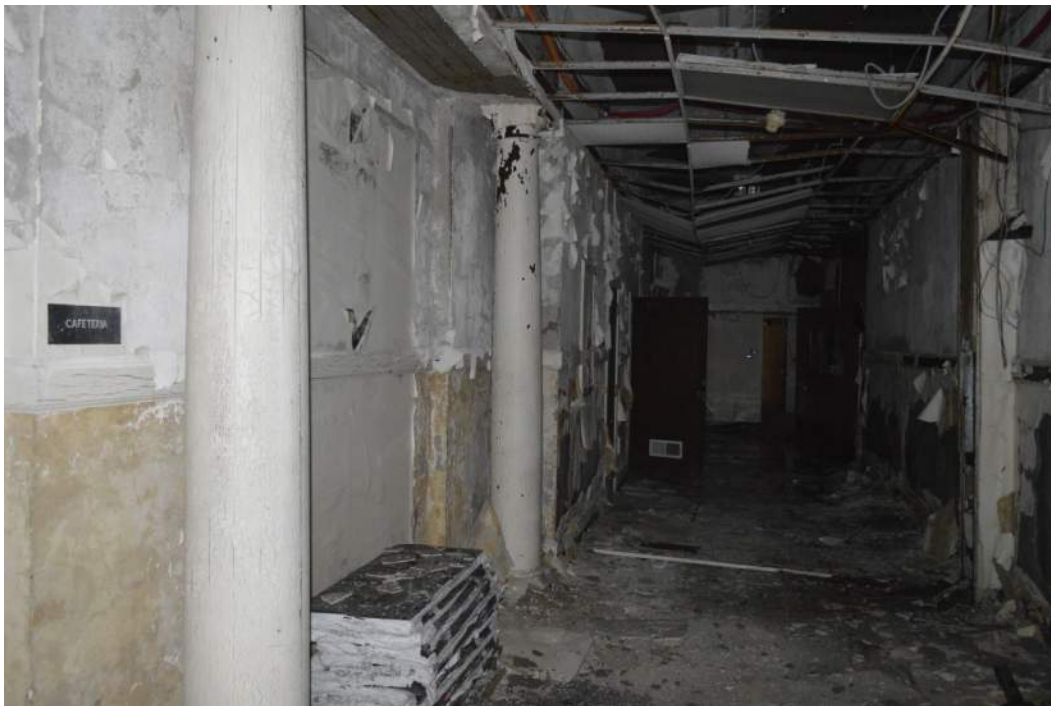
Photo 11: The staved wood columns outside of the Auditorium in the main corridor should be salvaged and refinished. Originally three double door openings provided entrance to the Auditorium. The entrance between the columns in this photograph has been blocked off, interrupting the symmetry.
