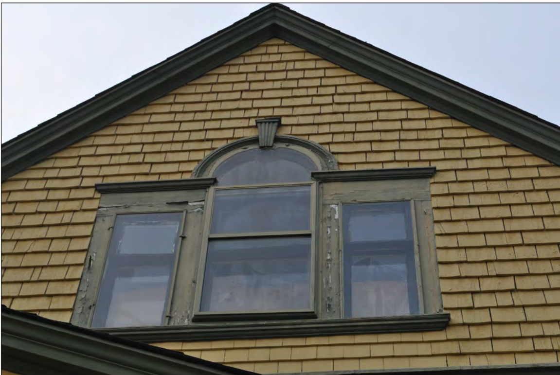
13. South elevation, camera facing up and north. Note missing trim on window surround.
