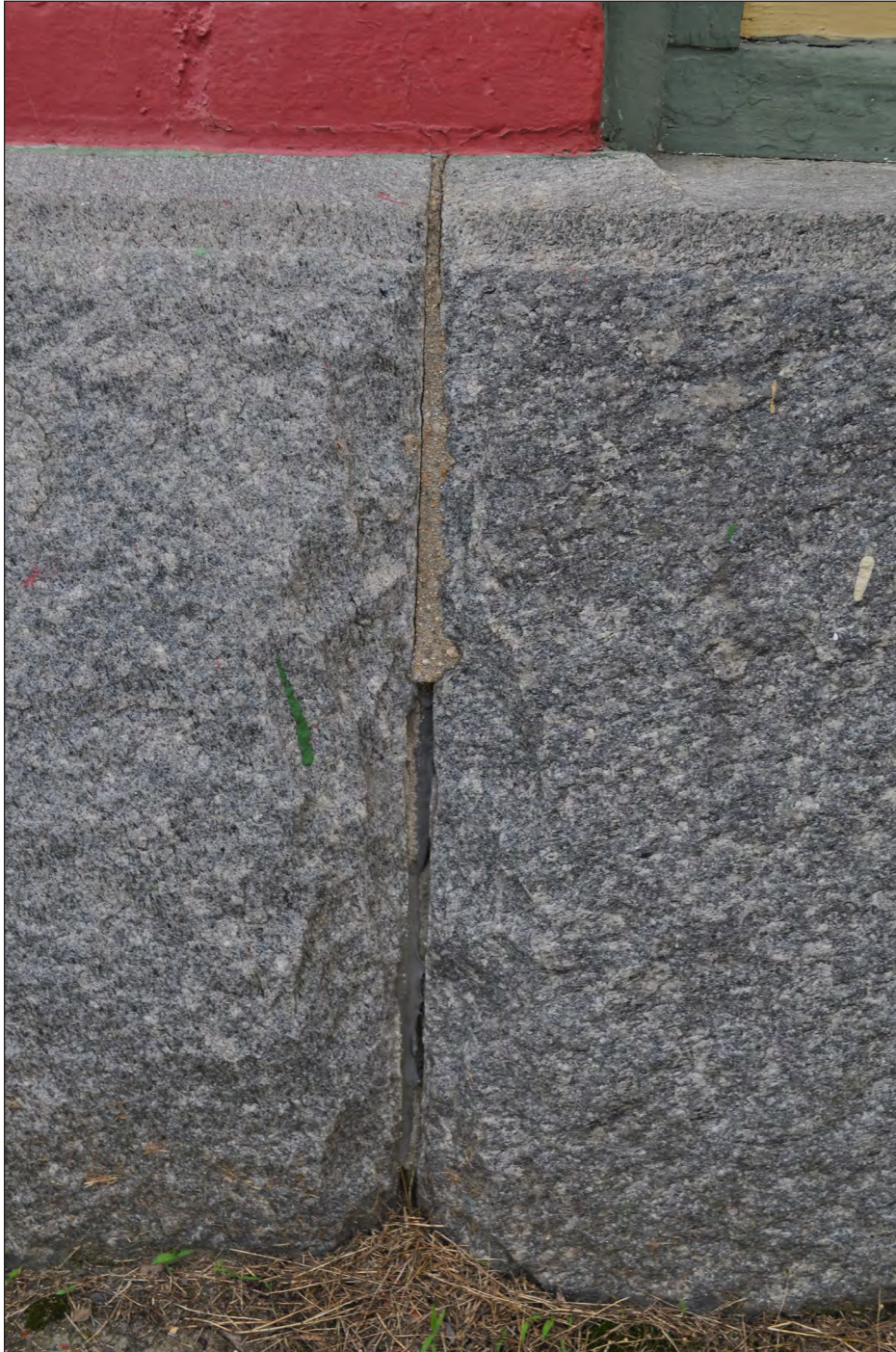
43. East elevation, missing mortar joint, camera facing down and west.
