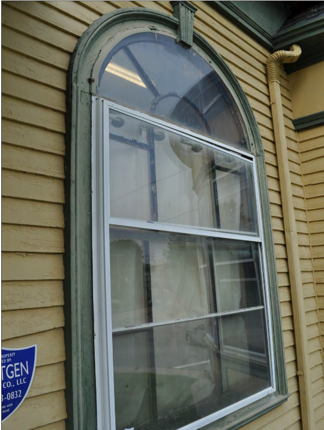
8. South elevation, close-up of window with exterior storm.
