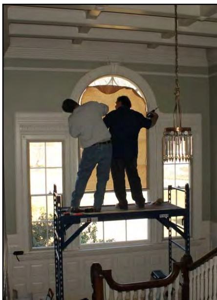
Installation of Palladian storm window
