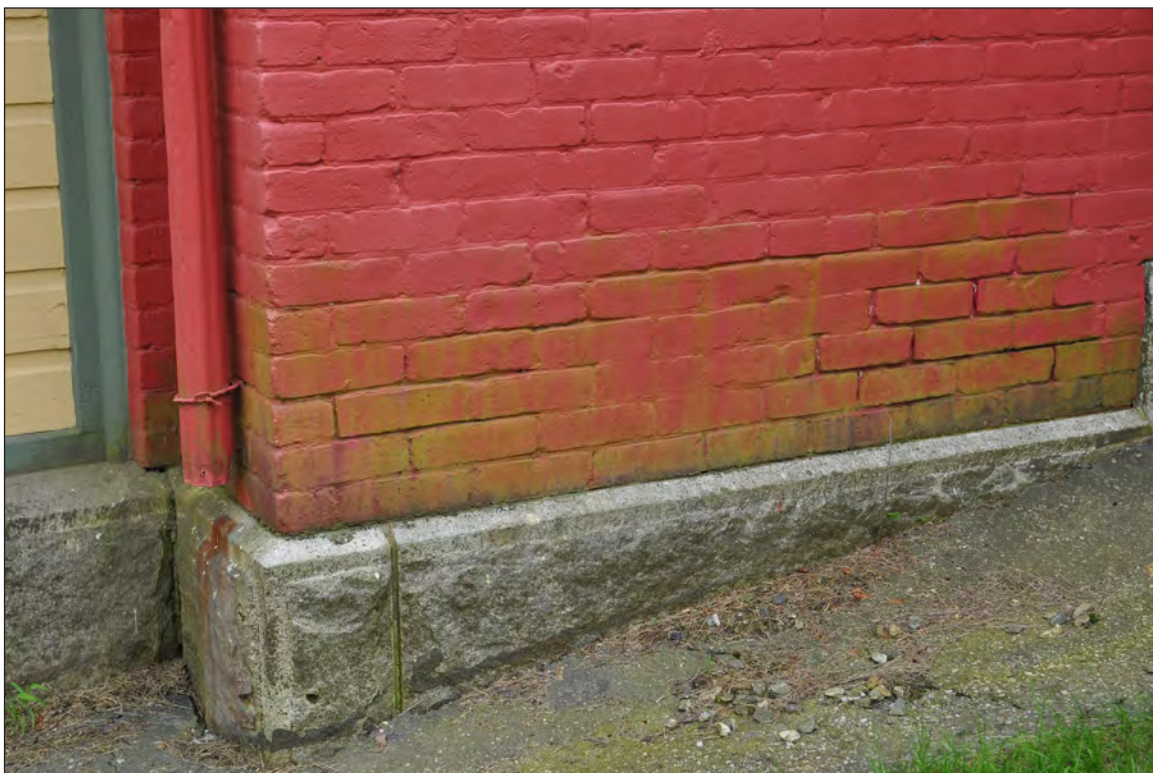
48. North elevation, camera facing down and southwest. Note bio growth and missing mortar.
