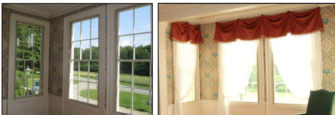
Interior storm windows installed
