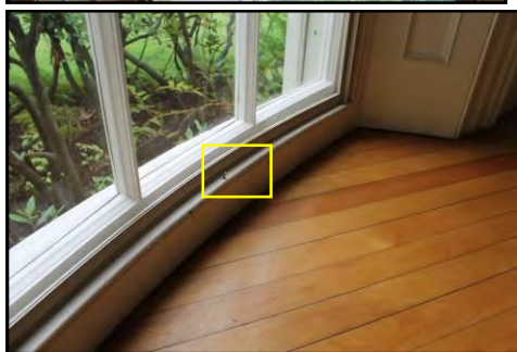
Above: additional rivet pin at bottom to hold curve of storm window
