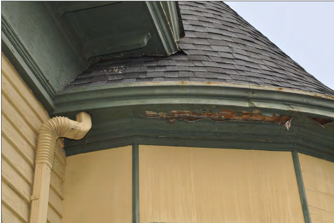
9. South elevation, west elevation of tower, camera facing up and northeast. Note deterioration of soffit boards.
