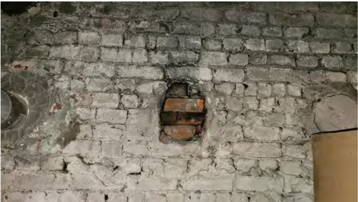
2. East wall of Furnace Room. Hole into inactive chimney should be properly sealed with brick.
