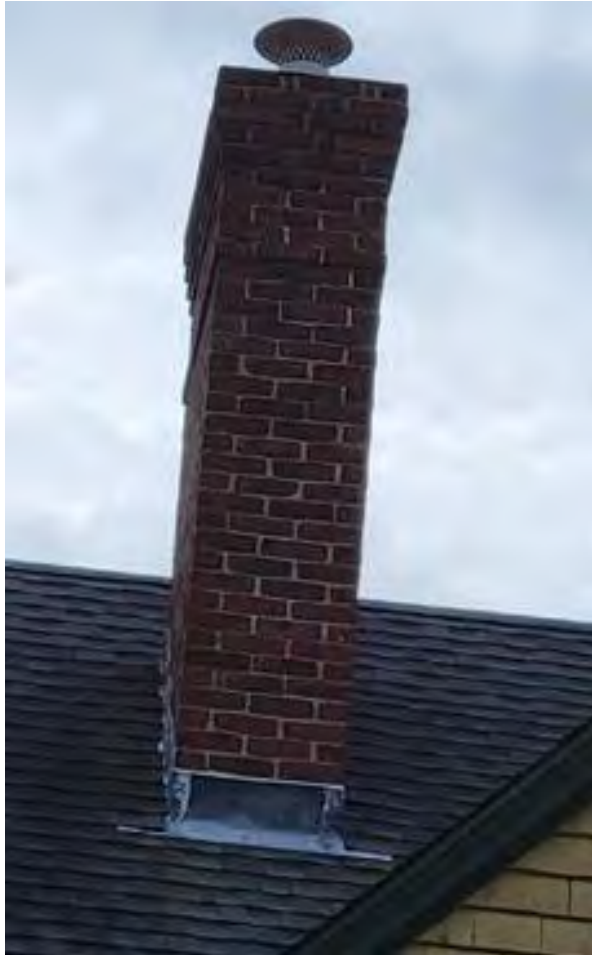
15. North chimney in good condition but needs repointing at top.
