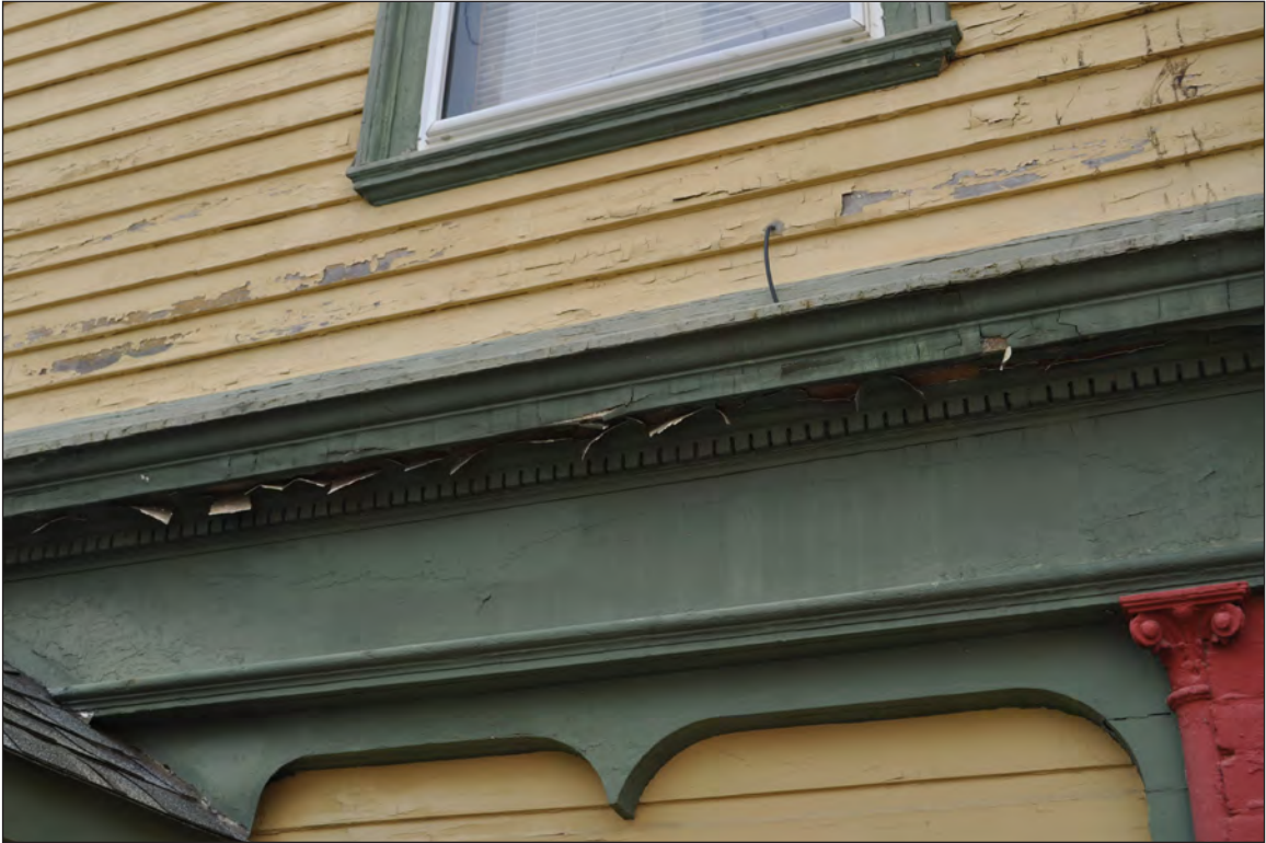
37. East elevation, camera facing southwest. Note conditions of clapboards and cornice components.
