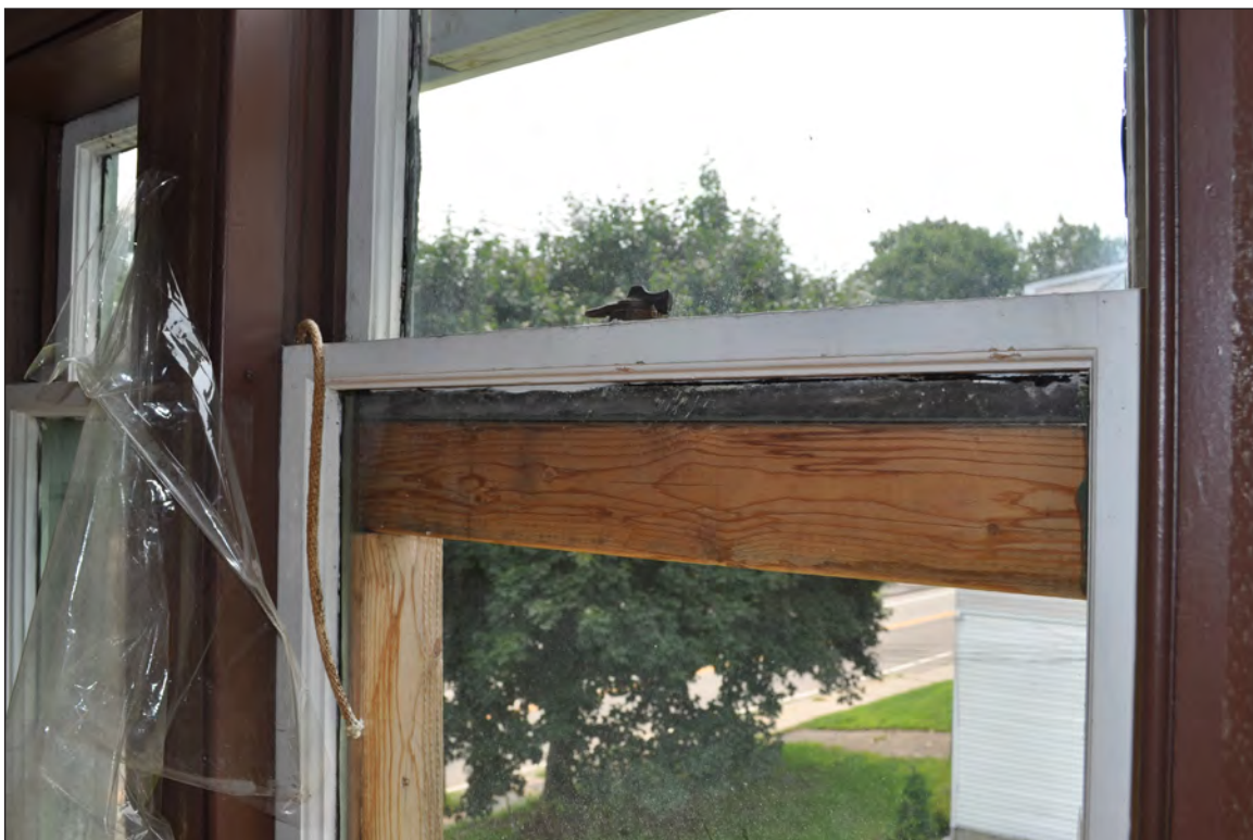
140. Second-floor, window in stair, camera facing southwest. Note broken sash and sash cord.
