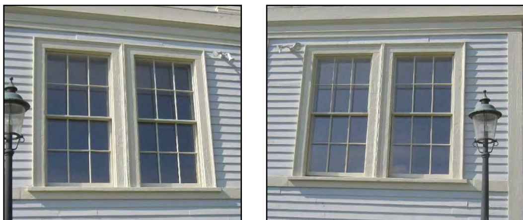
Interior storm windows installed Note muntin reflection in top sash
