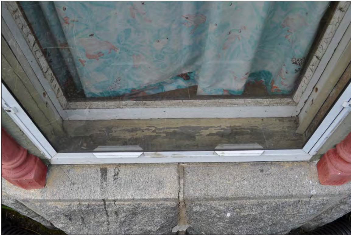
21. South elevation, tower, camera facing down and north. Note deteriorated window sash and sill.
