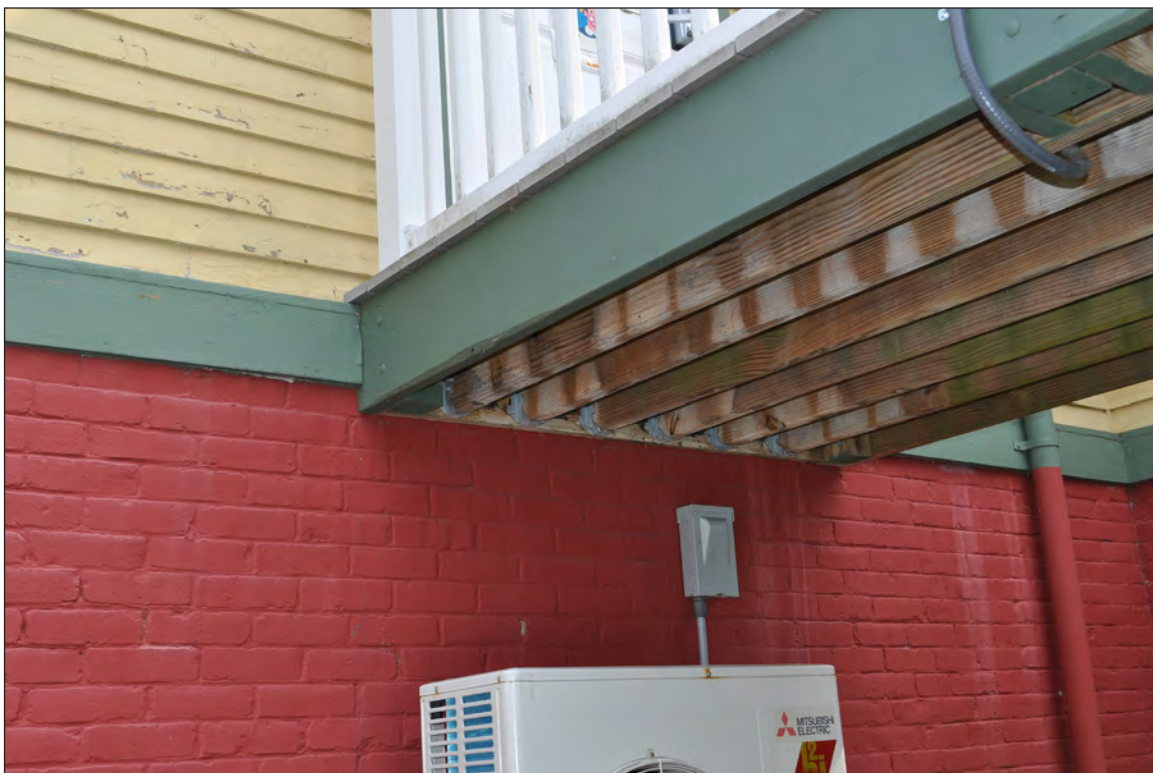
50. North elevation, camera facing southwest. Underside of deck, note bio growth.
