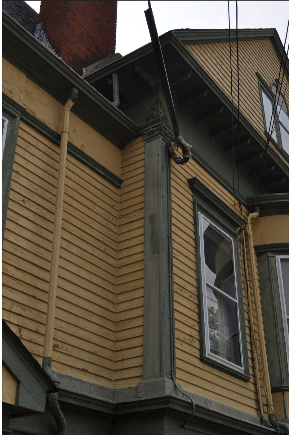
36. East elevation, camera facing northwest. Note condition of clapboards and corner pilasters.
