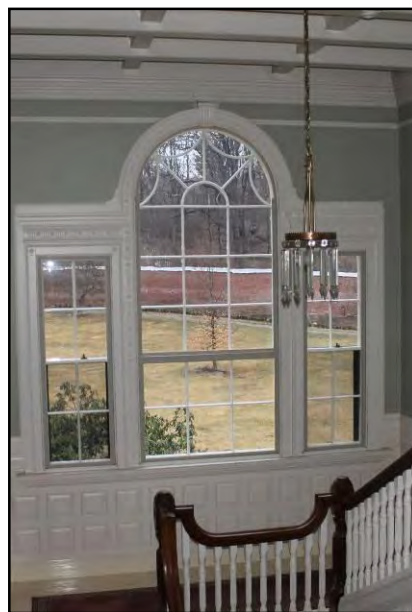
Palladian storm window installed
