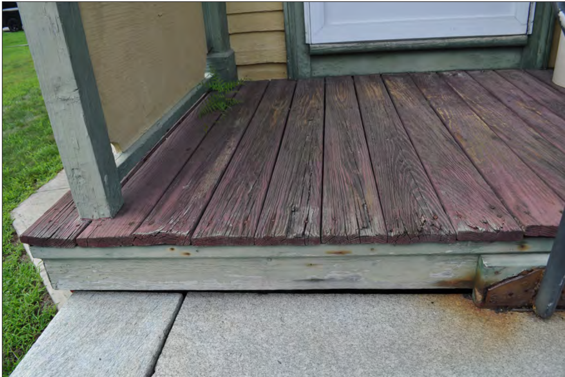
6. South elevation, deteriorated porch boards, camera facing down and north.
