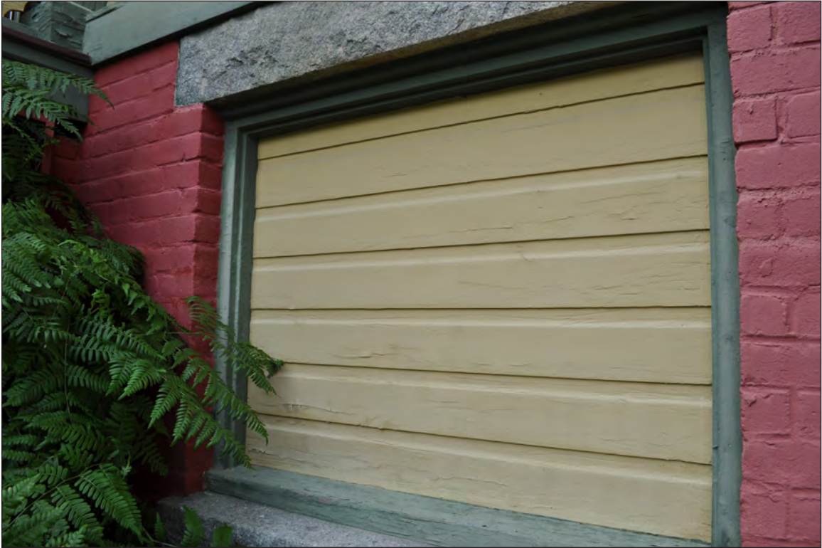
17. South elevation, infill of basement window, camera facing northwest.
