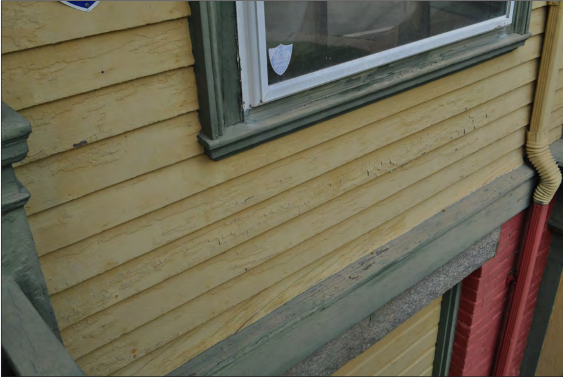
12. South elevation, camera facing down and northeast. Note deterioration of water table boards.
