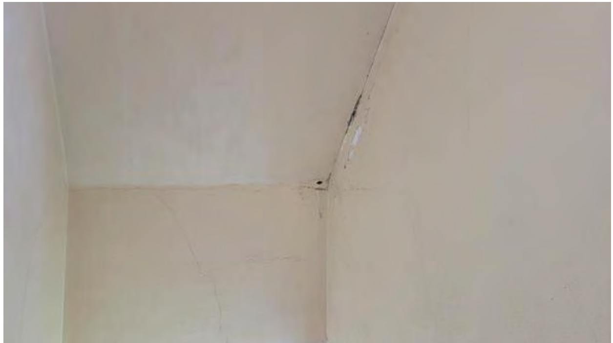
8. Additional stairwell ceiling and wall cracks and localized damage from leak. Not a structural concern.
