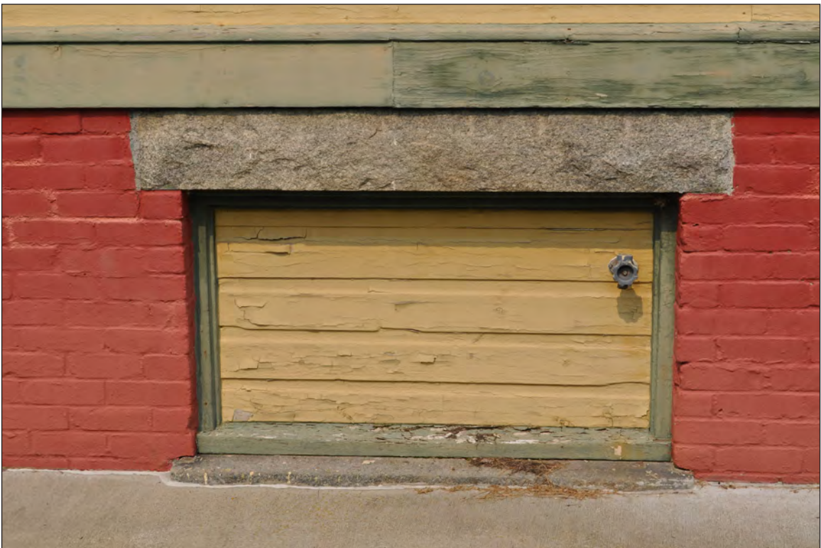
64. West elevation, infilled window, camera facing down and east.
