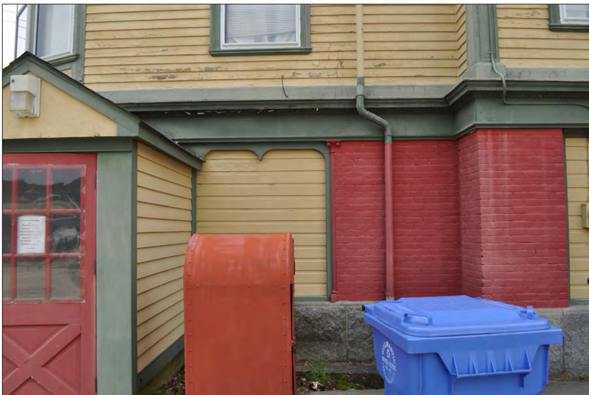
31. East elevation, infilled windows, camera facing west.
