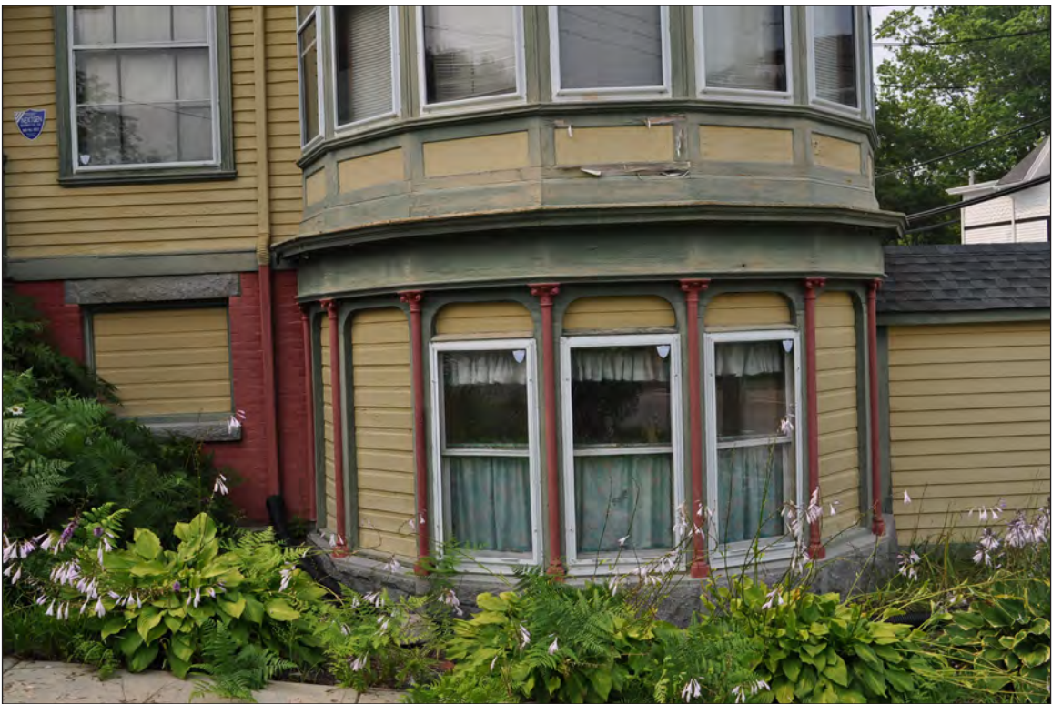
20. South elevation, tower, camera facing north. Note deteriorated of bulkheads below first-floor windows.
