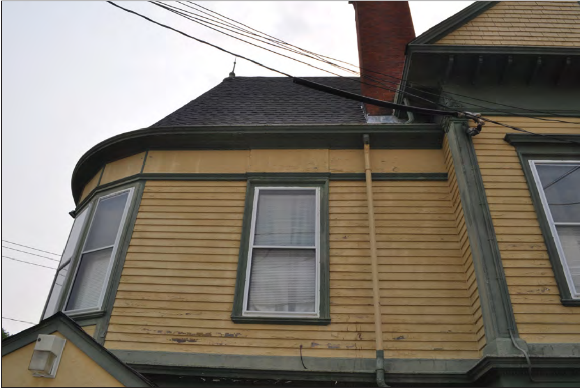
34. East elevation, camera facing up and west. Note condition of clapboards.
