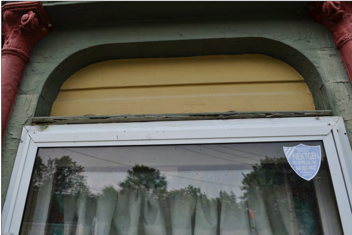
23. South elevation, tower, camera facing up and north. Note deteriorated flashing at top of storm window and infilled transom above.
