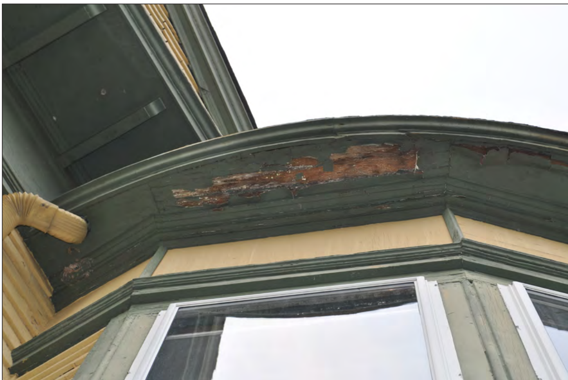
10. South elevation, west elevation of tower, camera facing up and northeast. Note deterioration of soffit boards.
