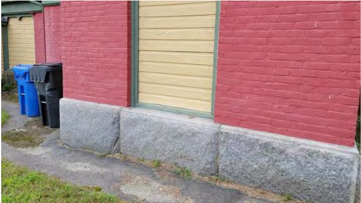
11. Typical granite quarry blocks at north, east and south walls. No sign of movement but vertical mortar joints require repointing.
