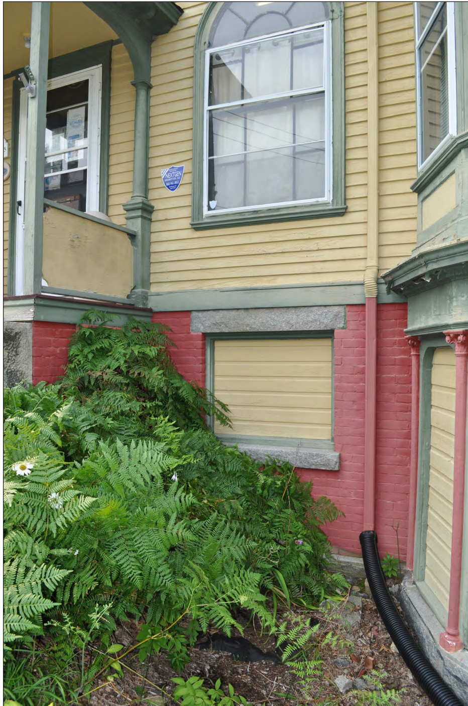
14. South elevation, vegetation growing against east elevation of stair.
