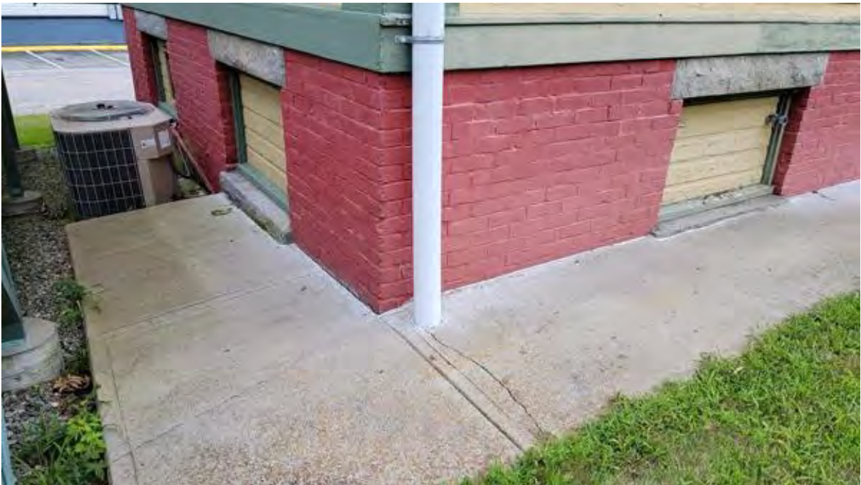
12. Concrete slabs along west wall protect wall from runoff. Concrete slabs should replace the bituminous swale to the northeast corner of the building.
