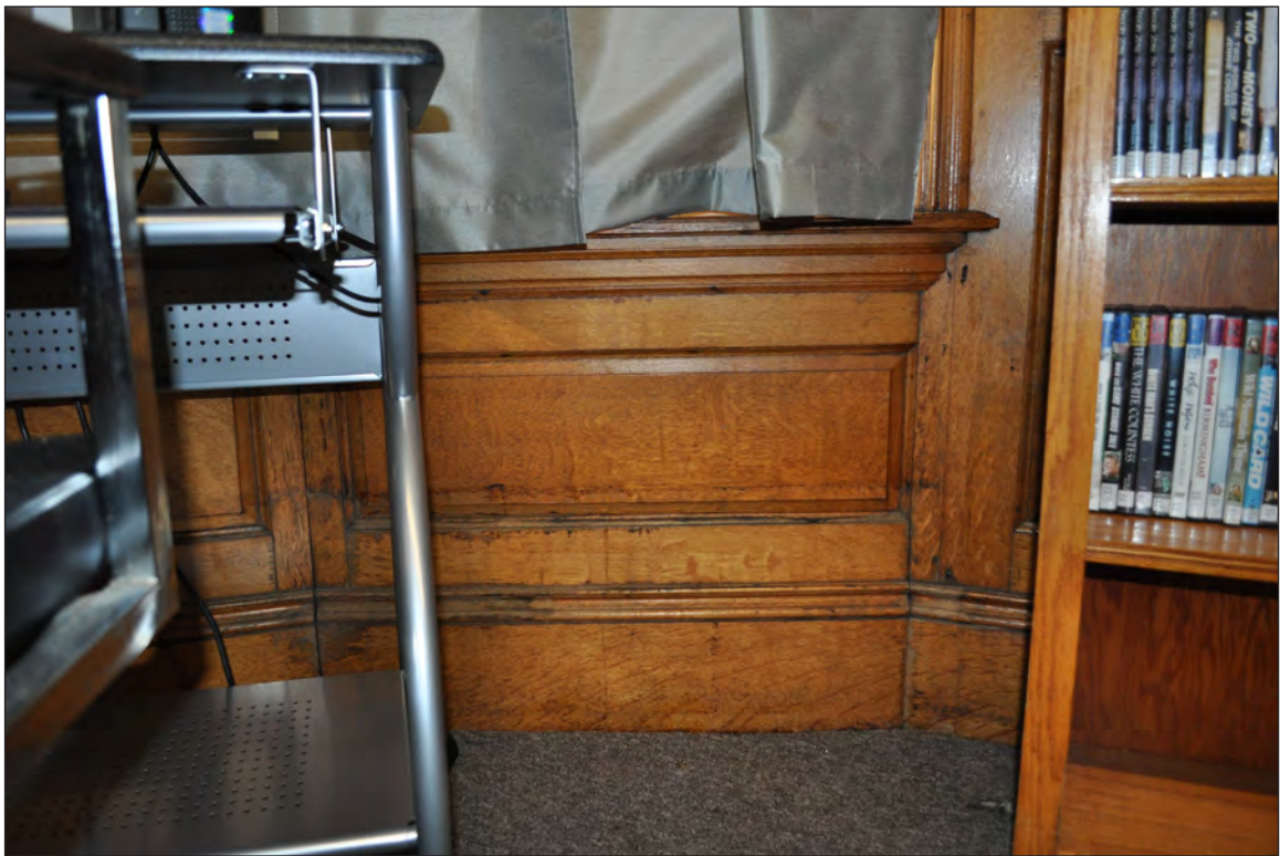
98. First-floor, computer room (201), camera facing southwest. Note staining on panel below window.
