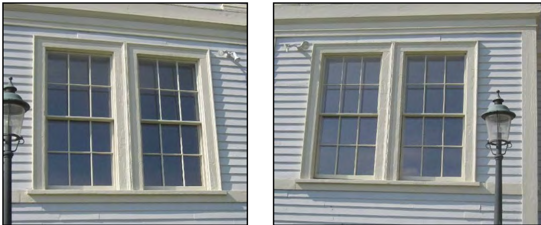
Interior storm windows installed Note muntin reflection in top sash
