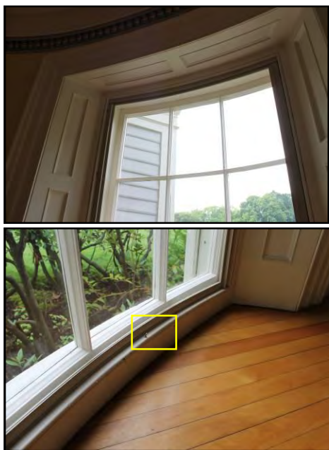
Above: additional rivet pin at bottom to hold curve of storm window
