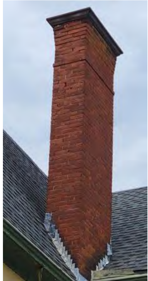
16. East chimney also in good condition but in need of some repointing.
