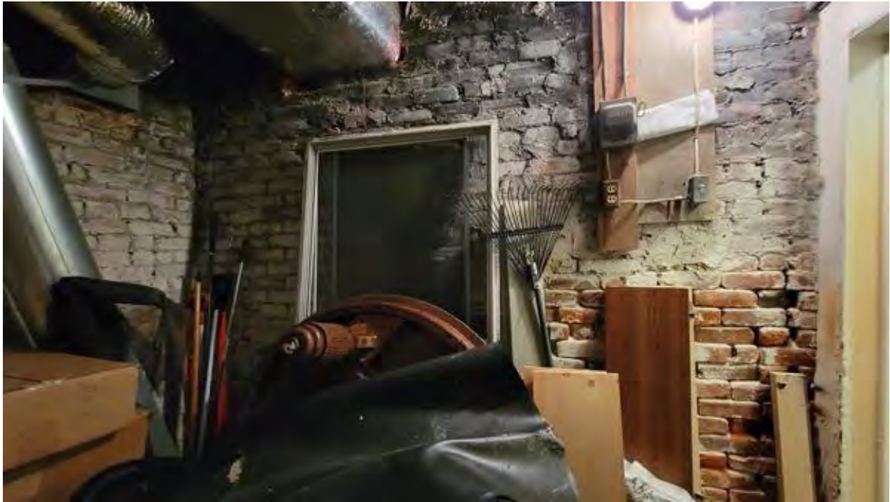
1. South wall of Furnace Room showing irregular brickwork and deterioration due to rising damp. Treatment is required to arrest the damp. Replacement of damaged brick units and repointing of mortar joints is also needed.
