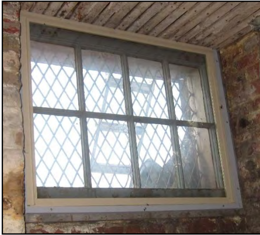
Basement window installation of storm window sash.
