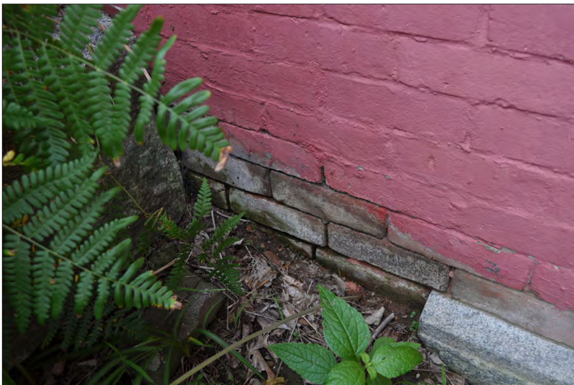
16. South elevation, vegetation growing against east elevation of stair. Note paint deterioration and missing mortar.
