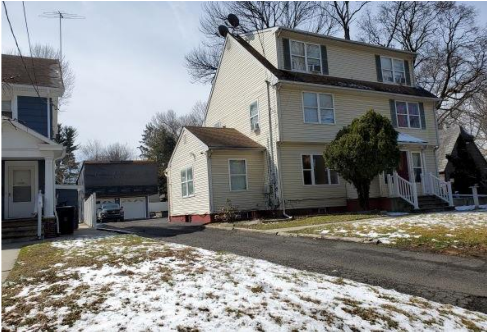
Image 2. Photo of subject principal structure at 812 Plainfield Ave, Block 506, Lot 12 (yellow house). Subject 2-car garage is to left of yellow house. Neighboring 2-car garage on Lot 11 shown to the right of yellow house. Looking southwesterly from Plainfield Ave.
