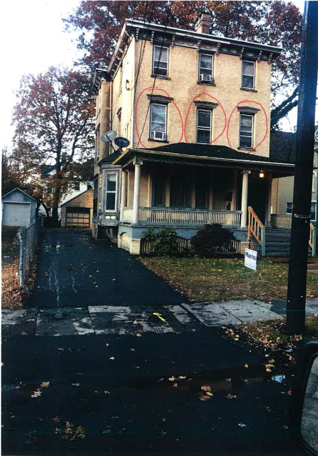
829 1 st Place. Asphalt driveway apron to be replaced with tinted concrete. The slate will be retained and reset. The three (3) 2 nd floor vinyl windows are to be replaced with Marvin wood 1 over 1 windows.
