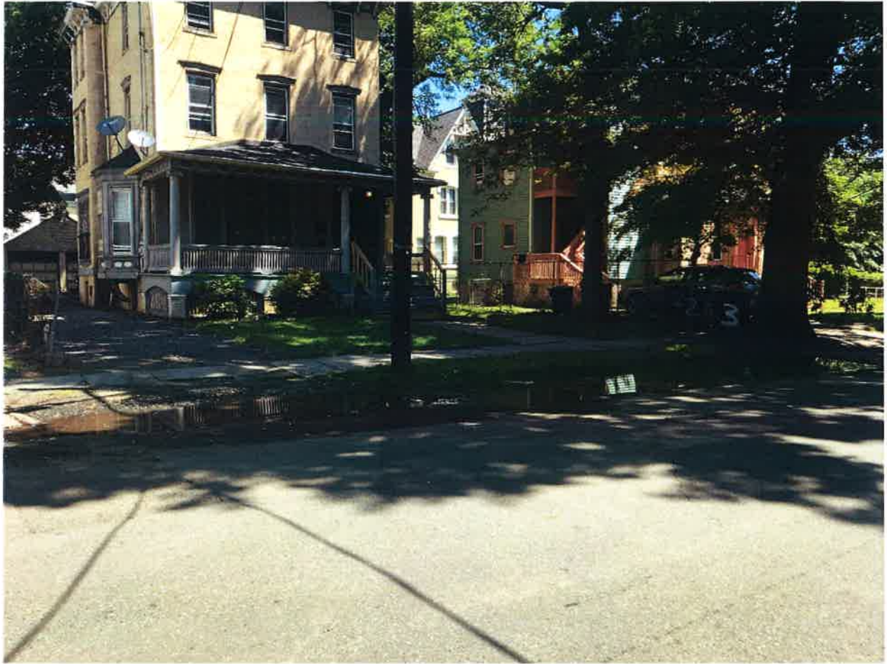
829 1 st Place before installation of asphalt driveway.
