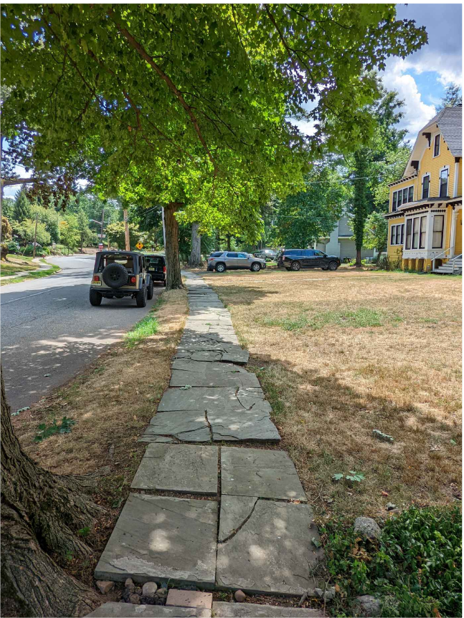
② SIDEWALK LOOKING SOUTH WALKWAY RAISED BY TREE ROOTS
