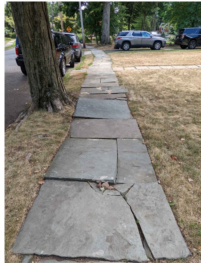
③ SIDEWALK LOOKING SOUTH CRACKED BLUESTONE SIDEWALK
