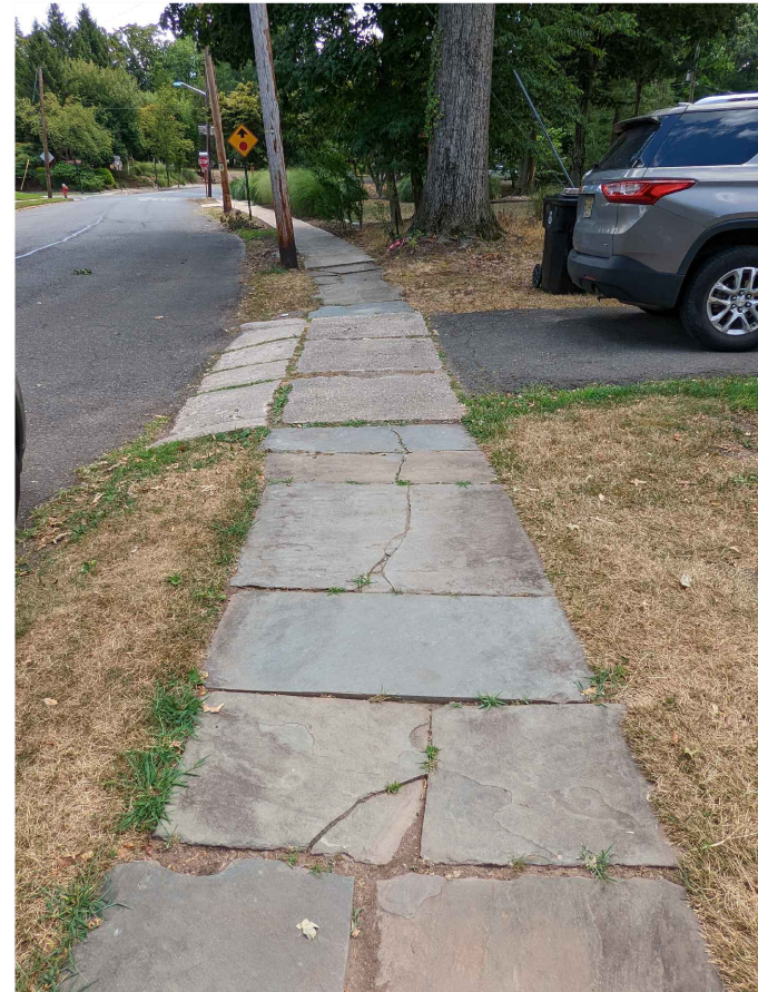
⑥ SIDEWALK LOOKING SOUTH CRACKED BLUESTONE SIDEWALK
