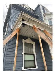
INSTALL 4x4x10 COLUMNS TO MATCH EXISTING COLUMNS,
