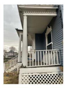
REPLACE ALL DECK FLOORING WITH TREADS (BULL NOSED) 1X4 TONGUE AND GROOVE CEDAR WOOD AND PAINT HASBROUK BROWN OR SIMILAR EXTERIOR GRADE BENJAMIN MOORE PAINT, (280 SF). USE 3.5" EXTERIOR SCREWS:
