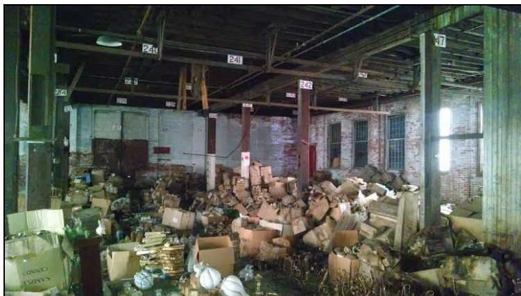
Storage, building interior
