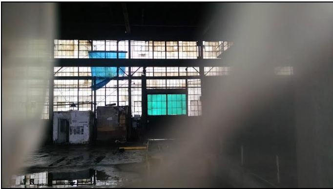
Building interior, vacant
