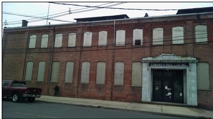
Looking north at front façade along South Avenue
