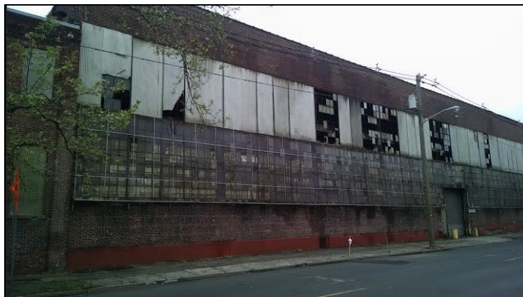
Looking north at front façade along South Avenue
