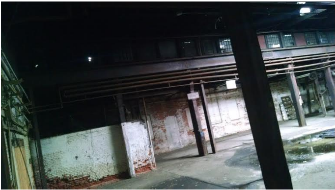
Building interior, vacant
