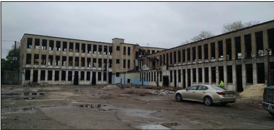
Rear of 639-661 South Avenue “Royal Apex Building” demolition work in progress
