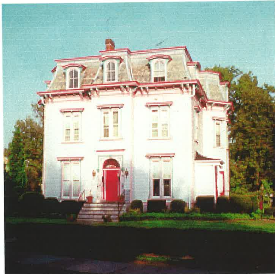
Crescent Area Historic District
