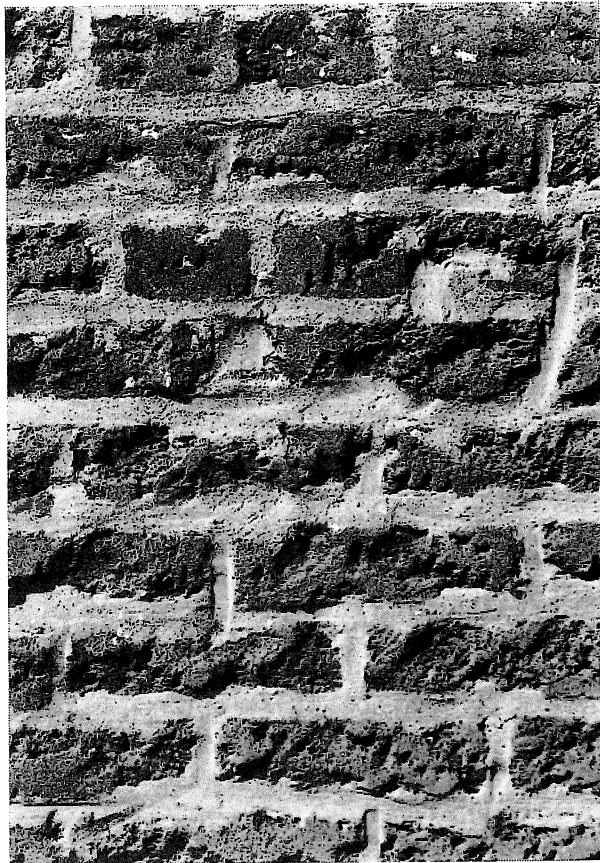
Sandblasting and improper repointing can do extensive damage to the outer surface and expose the porous inner part of brick.
