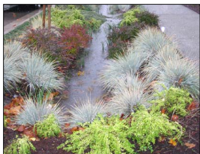
Best management practices such as bioswales help to increase the natural infiltration of stormwater. Bioswales are landscape elements designed to remove silt and pollution from stormwater runoff (Source:MRSC).
