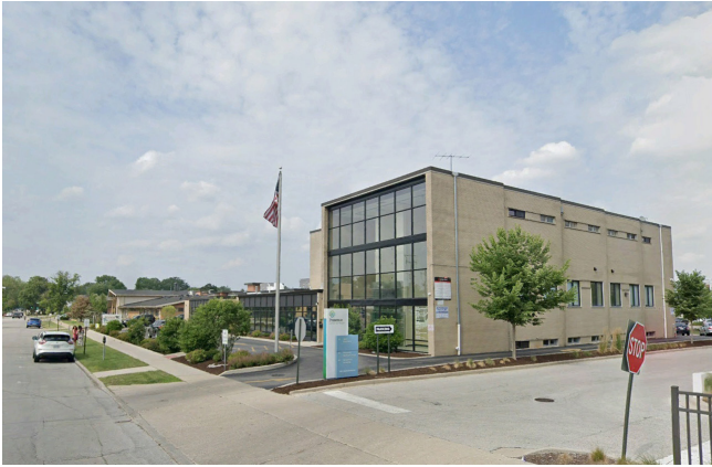
Figure 93: Businesses and setbacks along Washington Avenue
