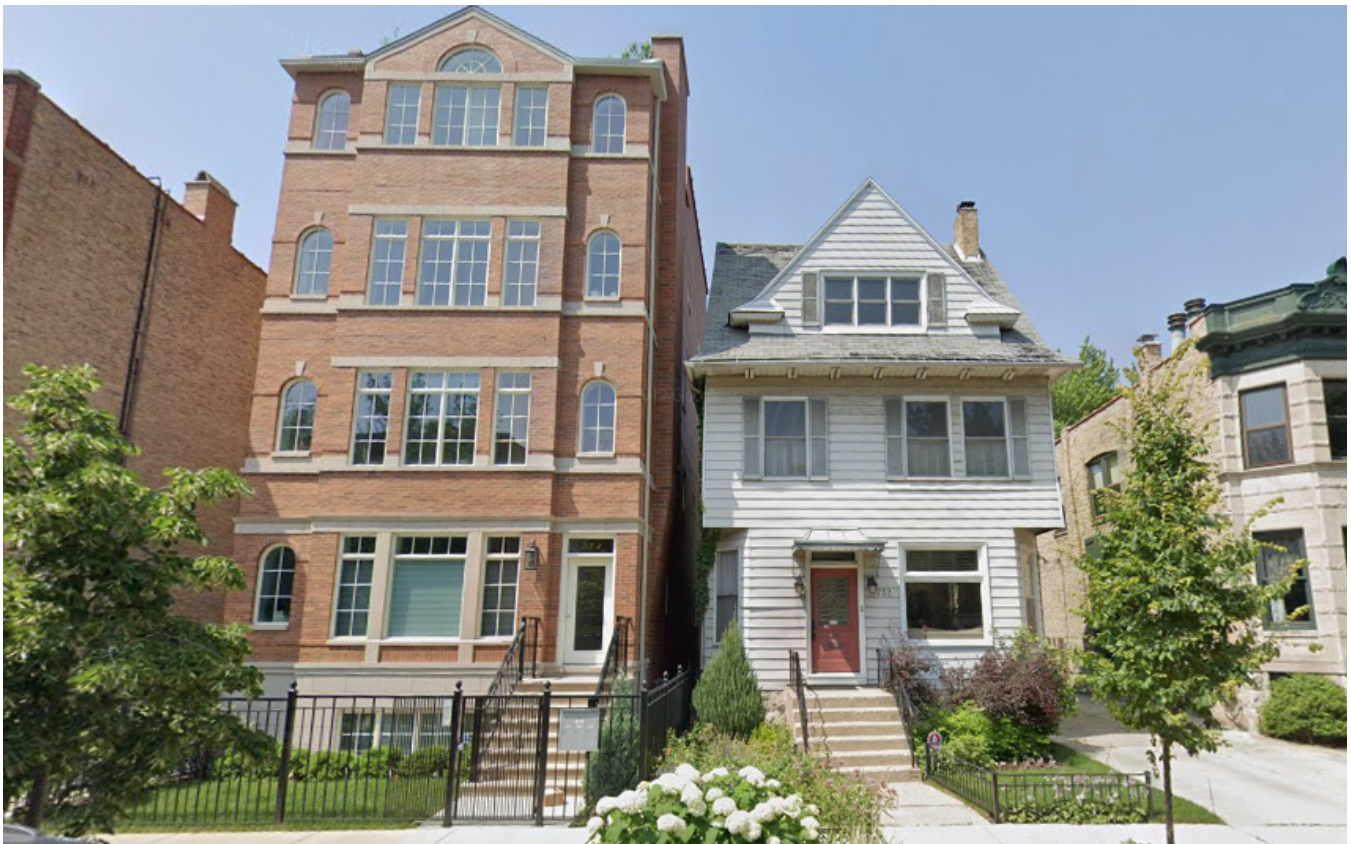
Figure 64: Goal #6 suggests a gradual stepdown from a higher- to lower-density. The above example shows an abrupt transition from a 4-story condo building to a single-family home. On the opposite end of the street, the same transition occurs by gradually stepping down building heights. To make the transition effective, all buildings should hold the same setback from the street.
