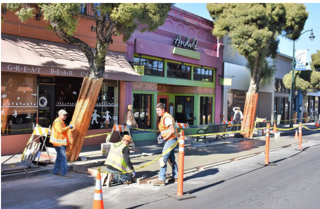
Figure 37: Construction of parklet in Los Gatos, California
