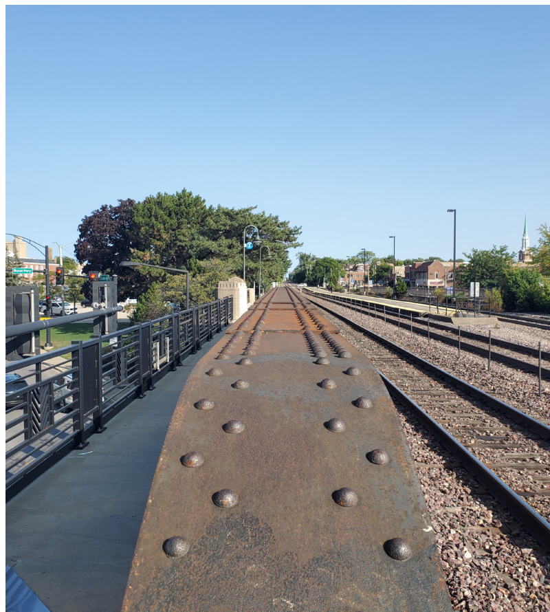
Figure 12: Metra Union Pacific Northwest (UP-NW) Line platform
