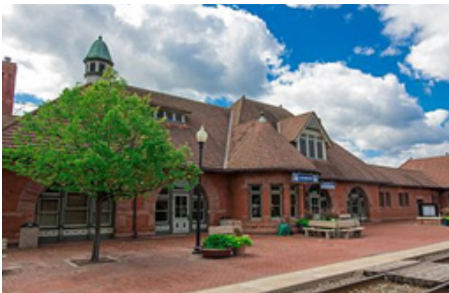
Figure 59: Kalamazoo Transportation Center platform
