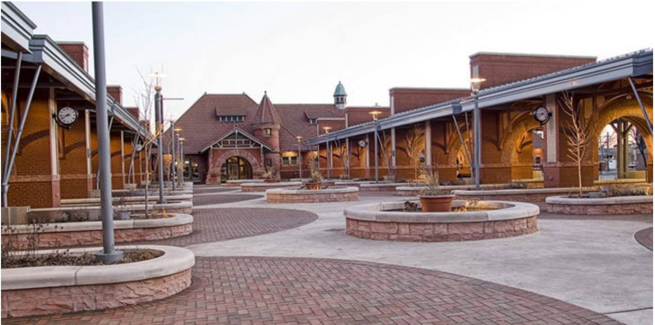
Figure 57: Characterizing infrastructure at Kalamazoo Transportation Center
