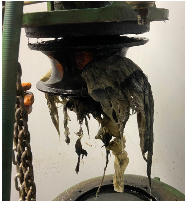
Wipes and debris in pump impeller at Lift Station #6
