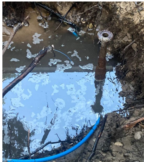
Water leak 6254 Ridge Road
