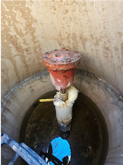
Air Relief Valve Before
