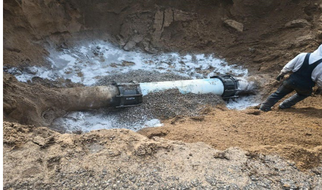
Perimeter Road force main repair
