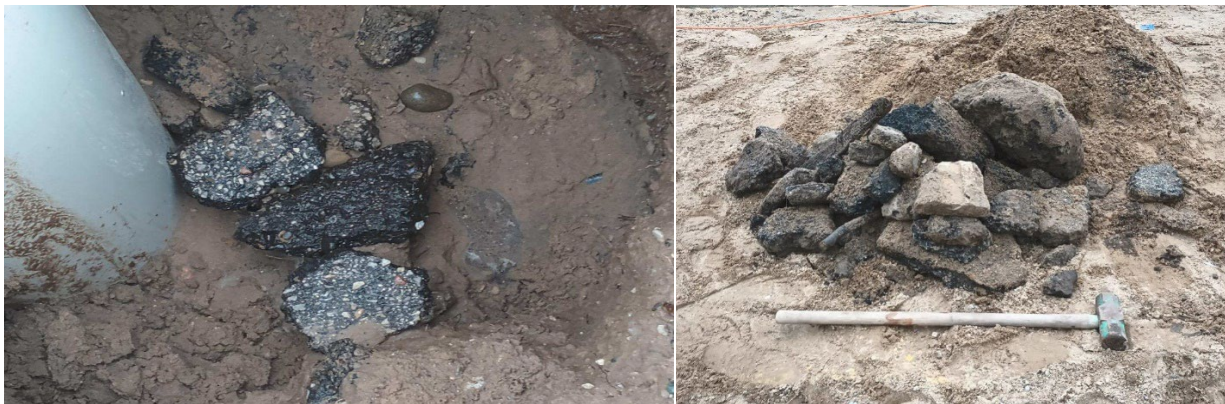
Backfill material next to meter pit at 5188 Bachman Rd
