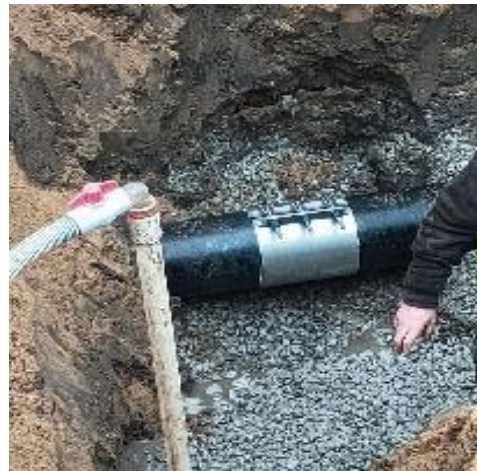
Repair clamp installed on water main
