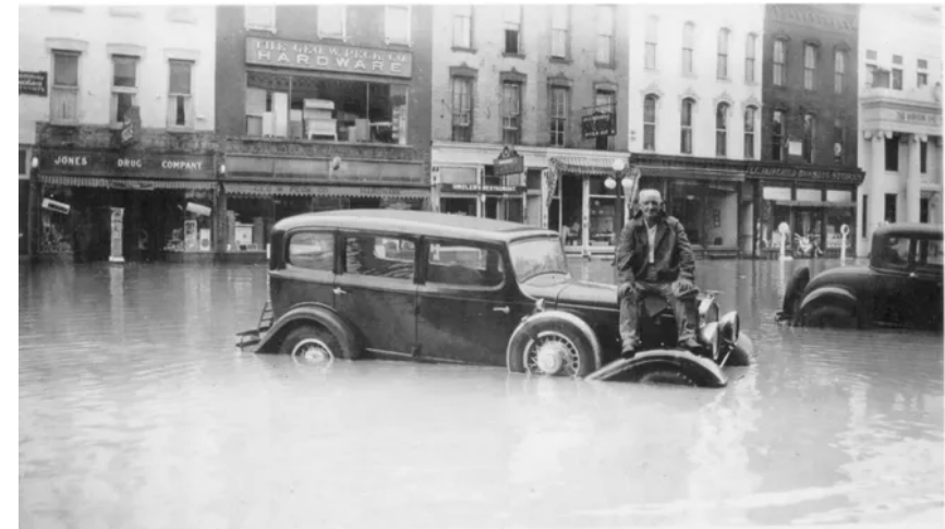
Bath, NY, 1935. Now protected by levees.
