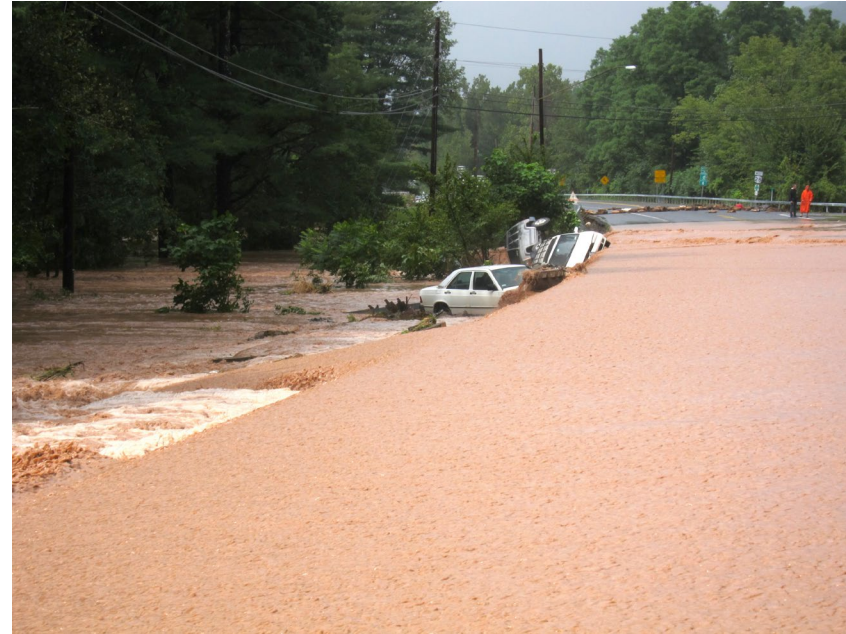
Flooding along Route 28 in Mt. Tremper, NY due to Tropical Storm Irene (Aug. 2011).
