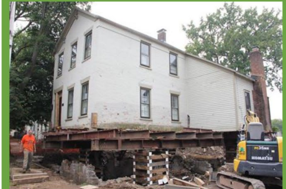
Elevation of Historic Flood-Prone Home in Stockade Neighborhood, Schenectady, NY
