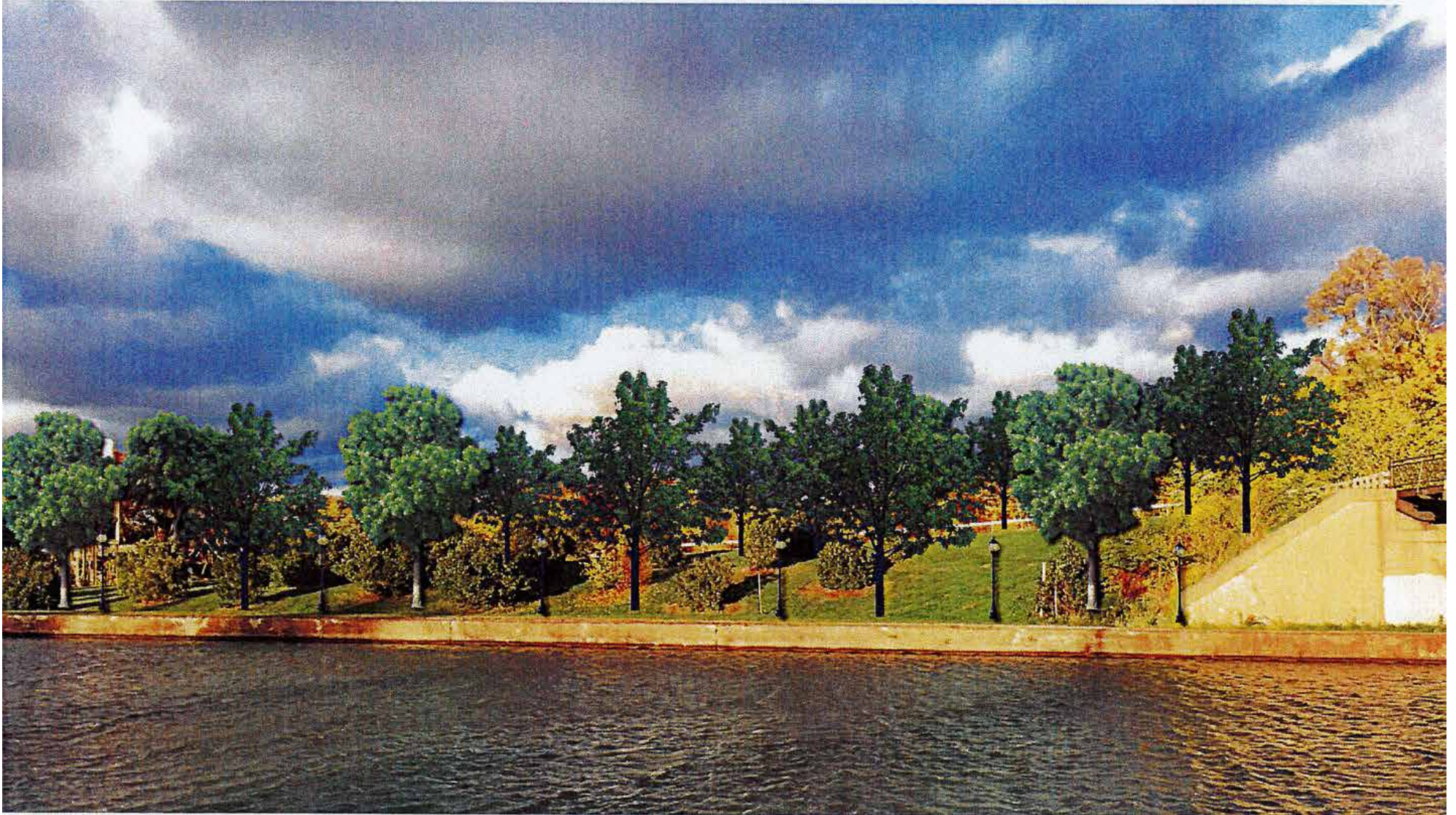
Lion's Park - South End/Towpath at Glenwood Avenue Bridge with trees and lighting.
