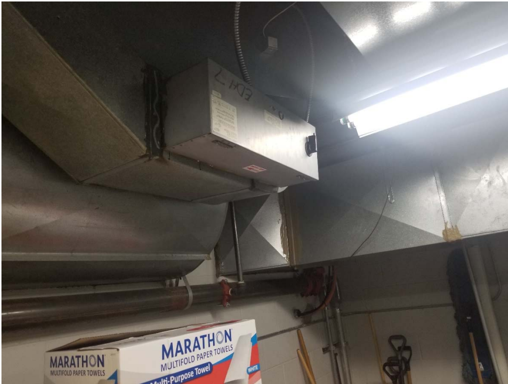
M7 Electric Duct Coil
