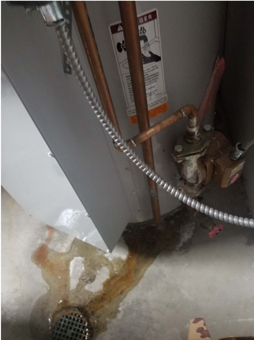
P7 Leak at domestic water heater
