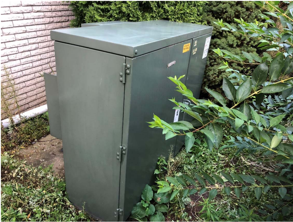
Picture E1 – DTE Pad Mounted Transformer
