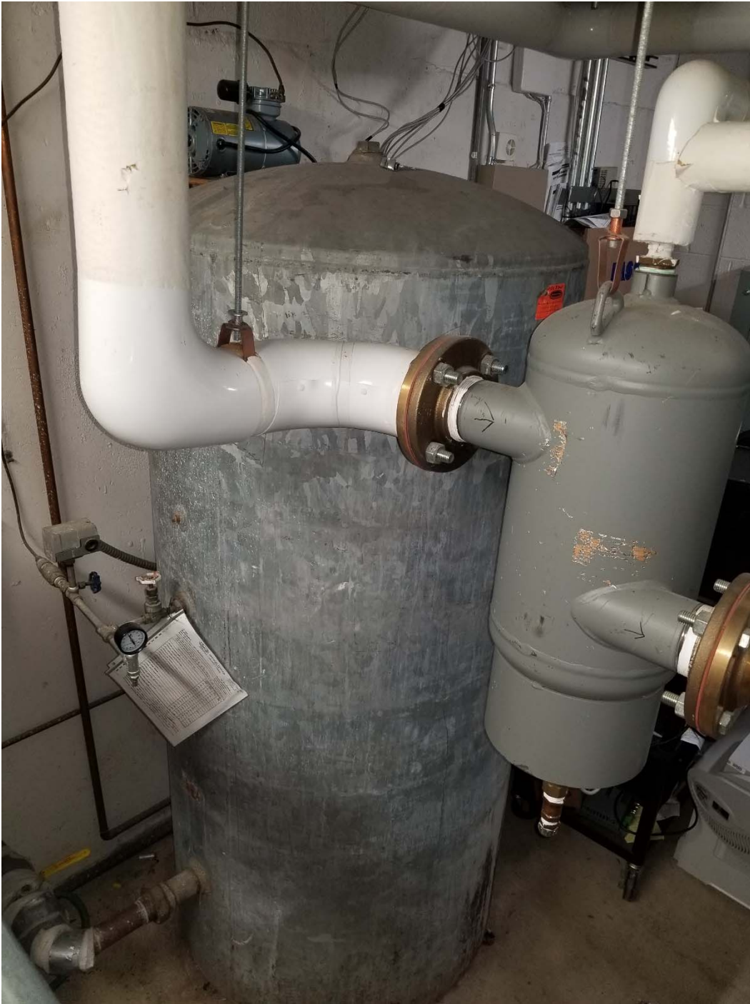
P5 Well Compression Tank
