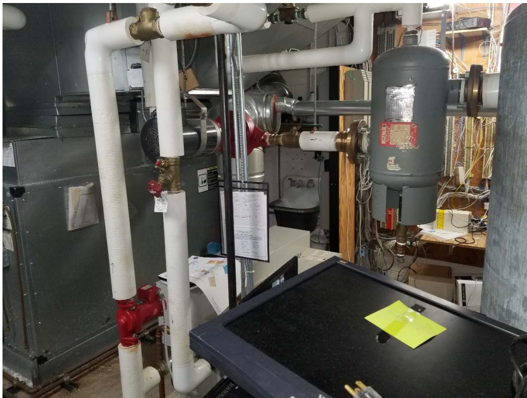
M2 Heating system pump and air separator
