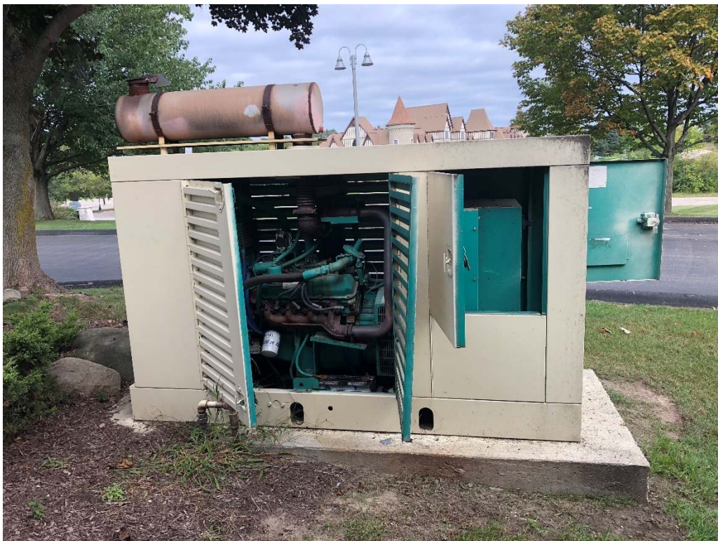
Picture E4 – Existing 100KW Generator
