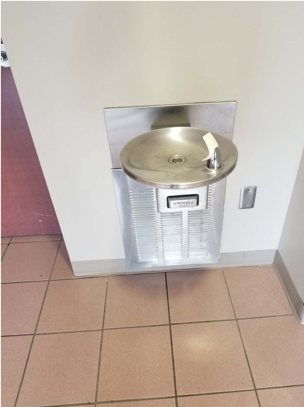
P9 Electric Water Cooler
