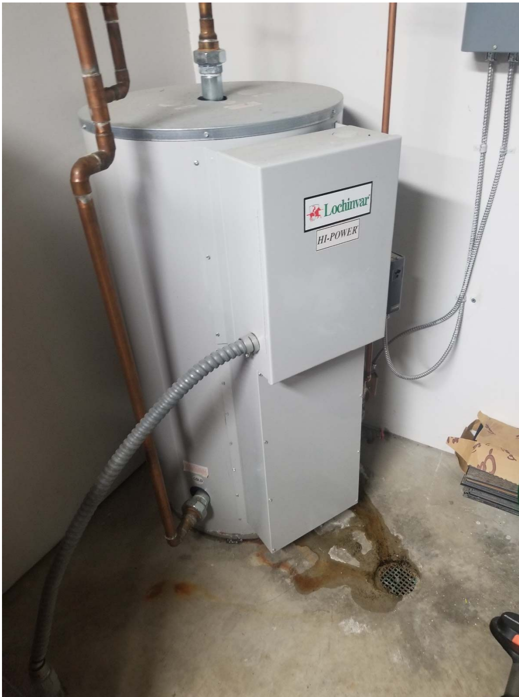
P6 Electric Domestic Water Heater
