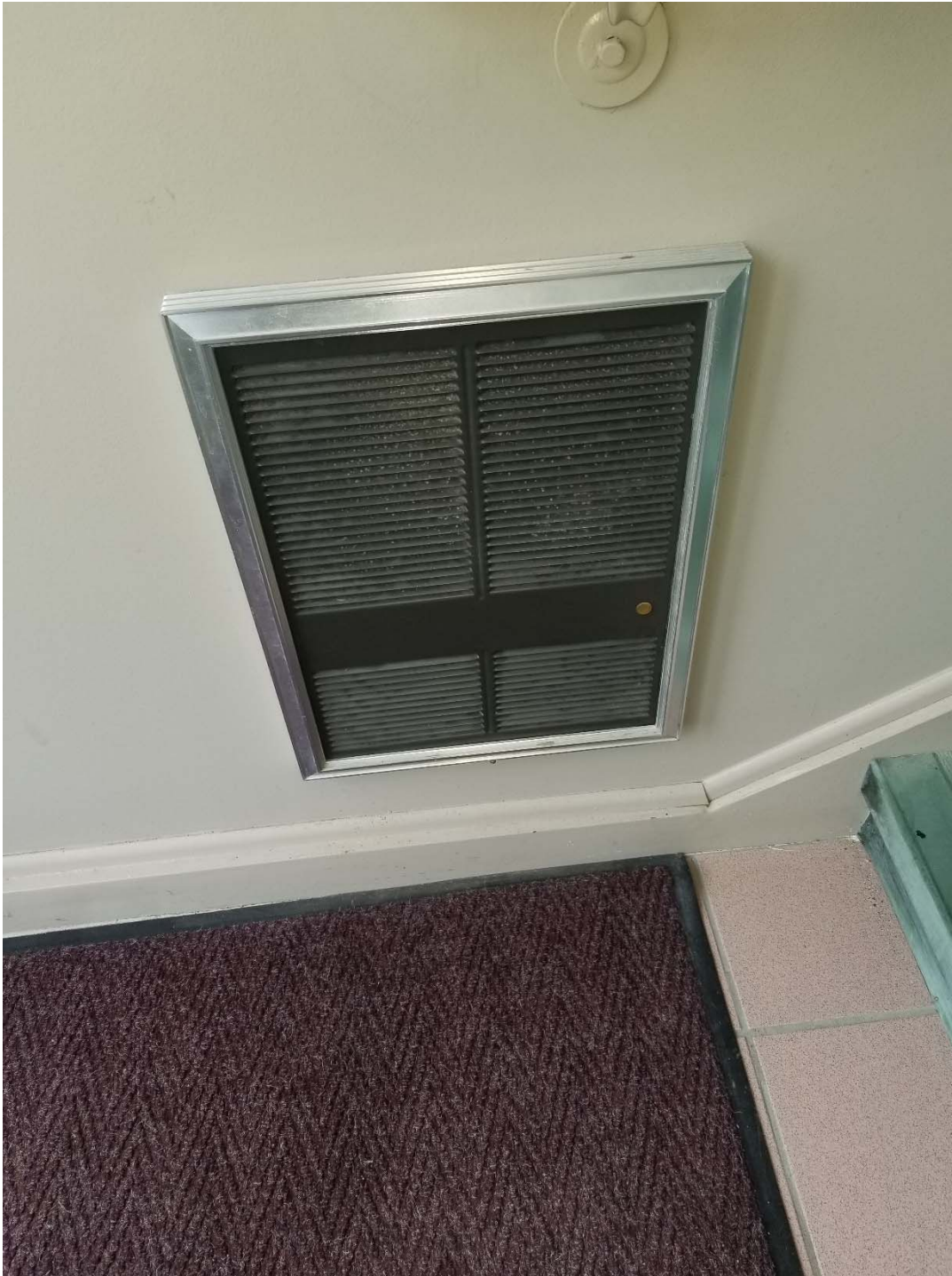
M5 Electric Cabinet unit heater
