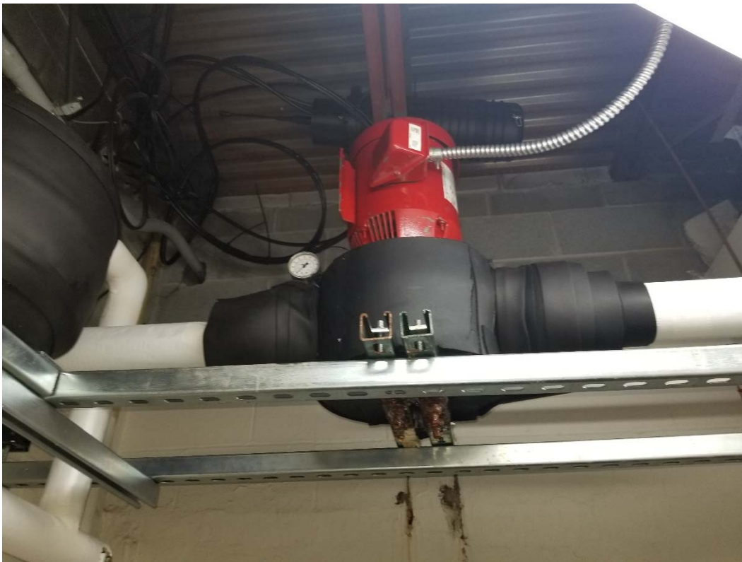
M8 Remote Heating Hot Water Circulating Pump
