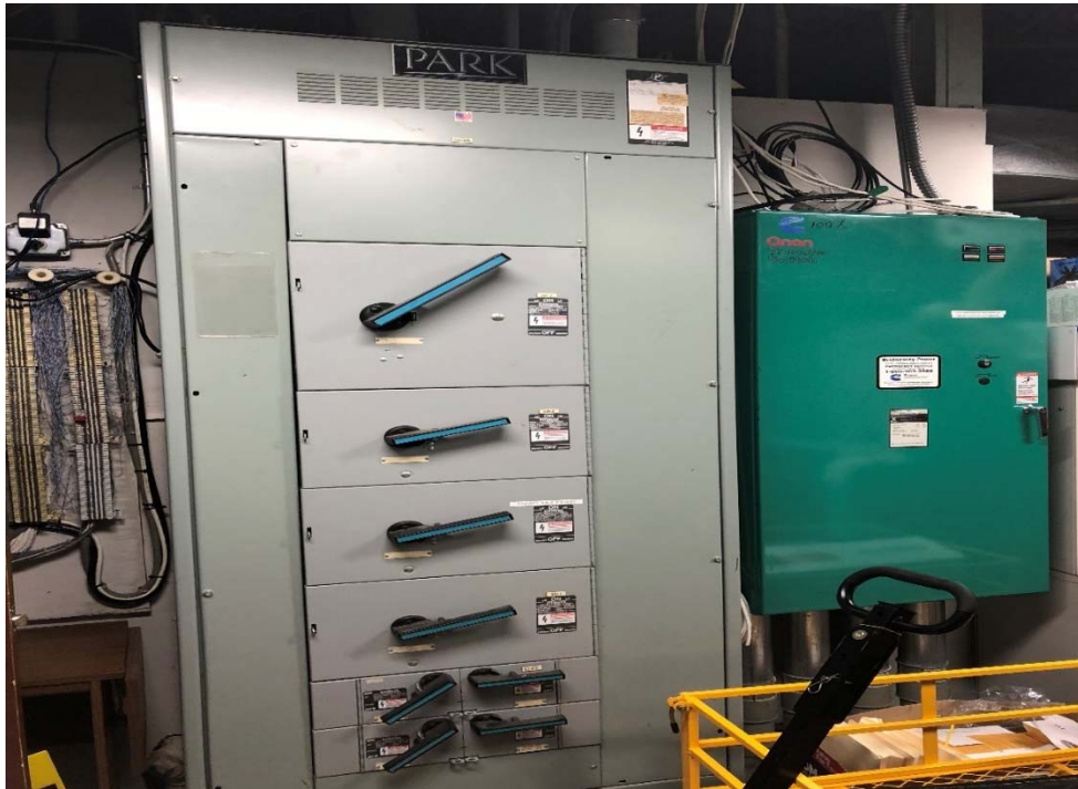
Picture E5 – Existing ATS and Emergency Load panel DP-SB
