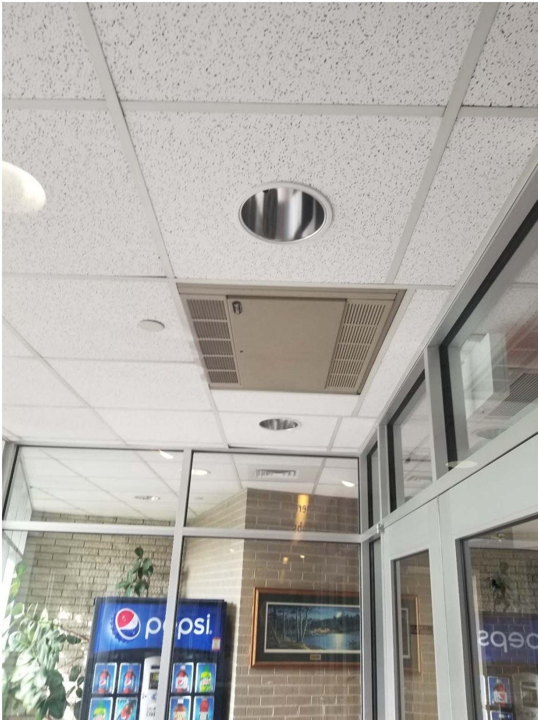
M6 Hydronic Cabinet Unit Heater
