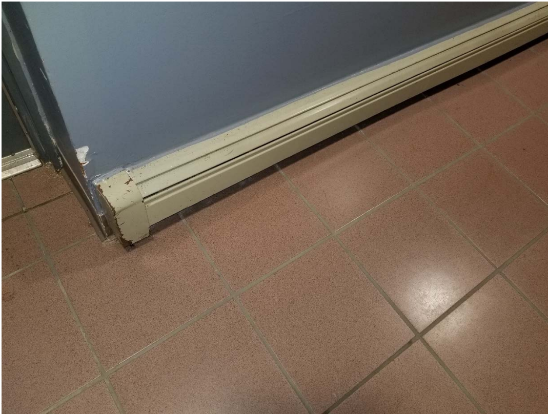
M3 Baseboard Fin Tube Radiation
