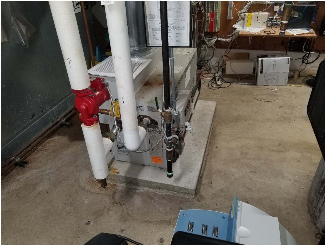
M1 Gas Fired Boiler
