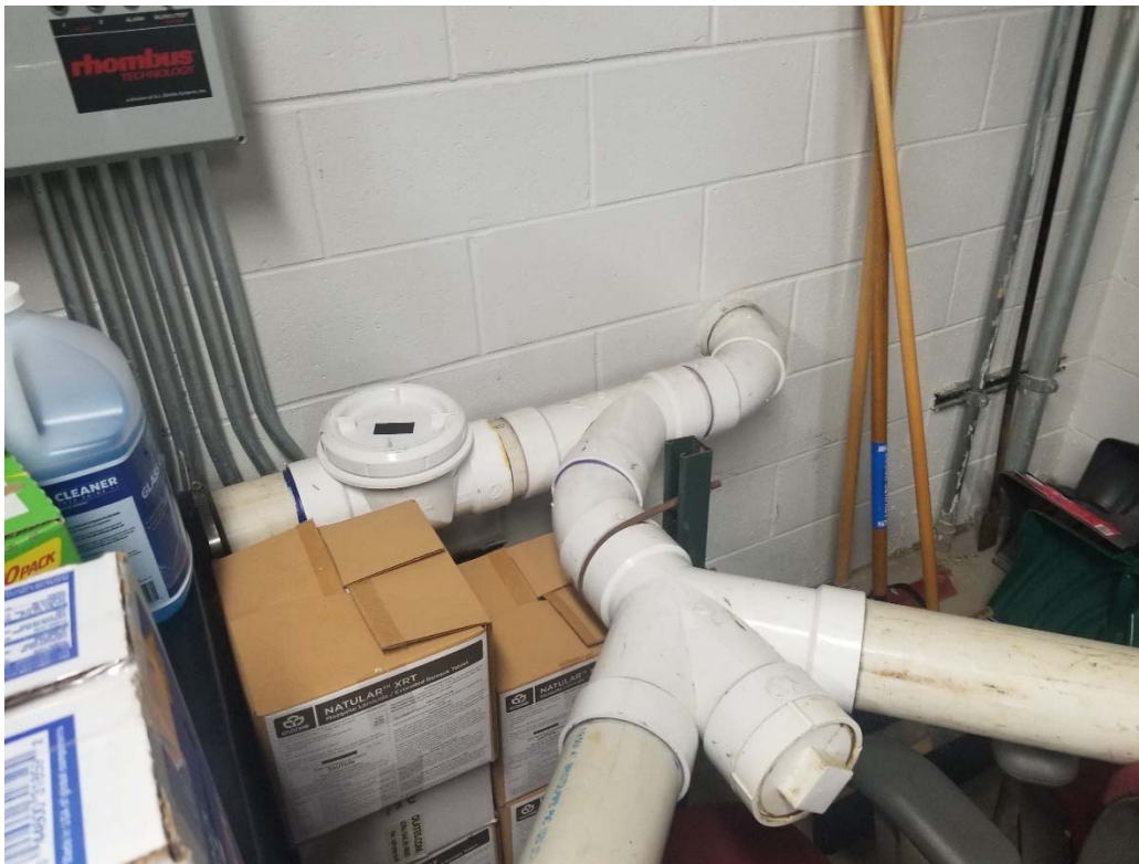
P1 Sanitary out of Building to Septic Field
