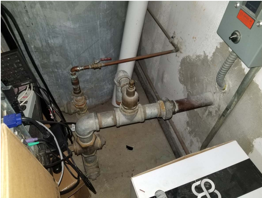
P4 Original Well Water Entry into Building
