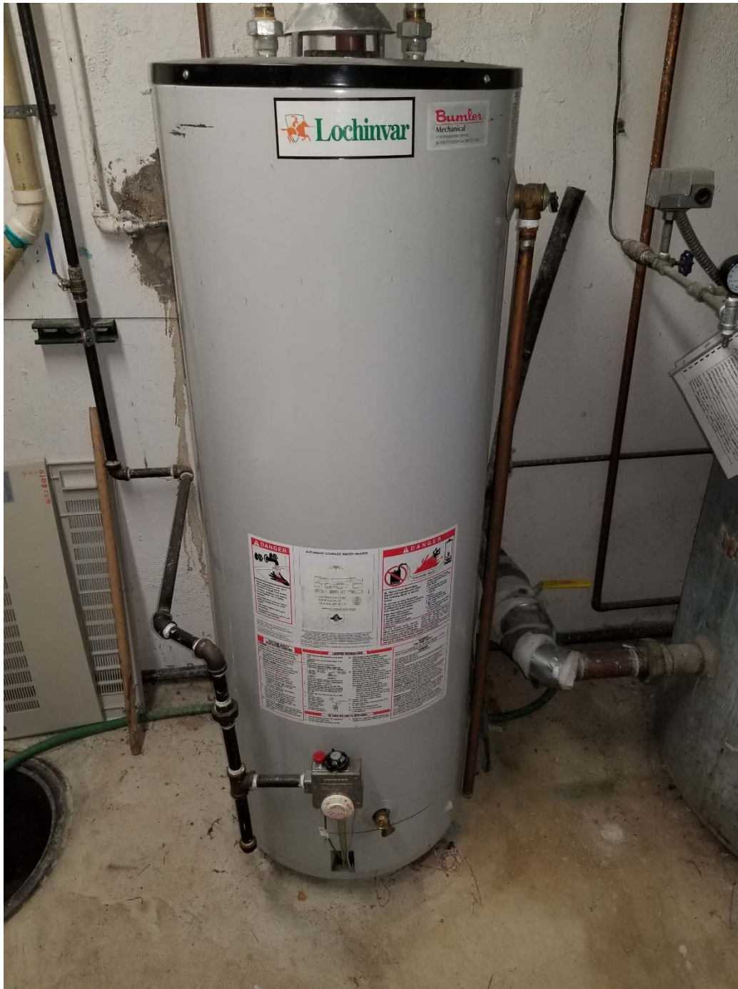
P8 Gas Fired Domestic Water Heater
