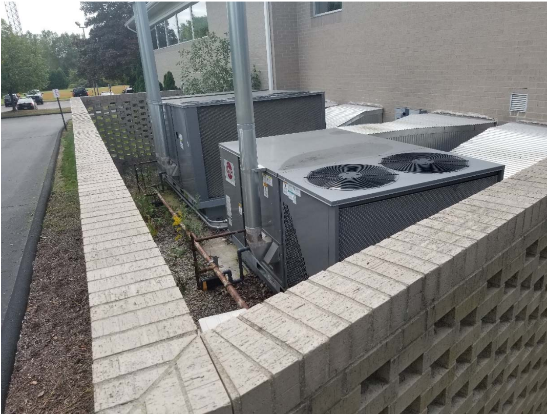
M11 Gas Fired Roof top units on grade
