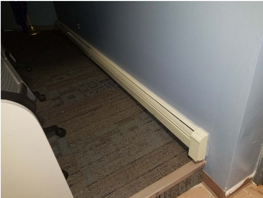
M4 Baseboard Fin Tube Radiation
