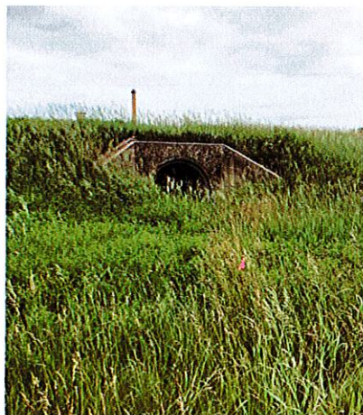
Wetland M: Culvert to Storm Network
