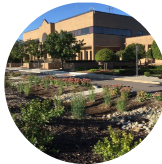
Bioswale installation at Clinton Township Civic Center
