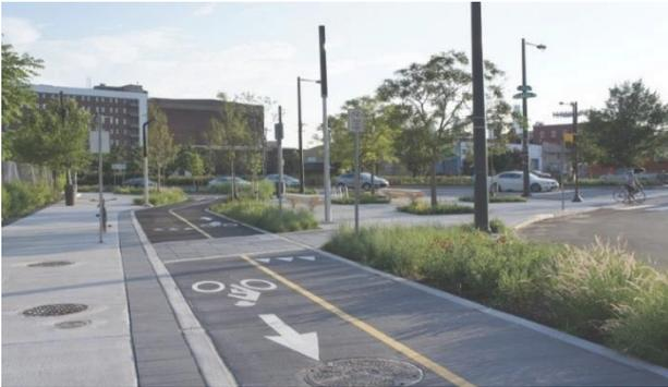
Figure 7: Example of Cycletrack with landscaped barrier
