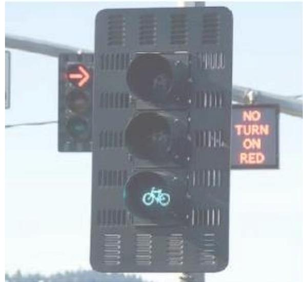
Figure 10: Bicycle specific signal head
