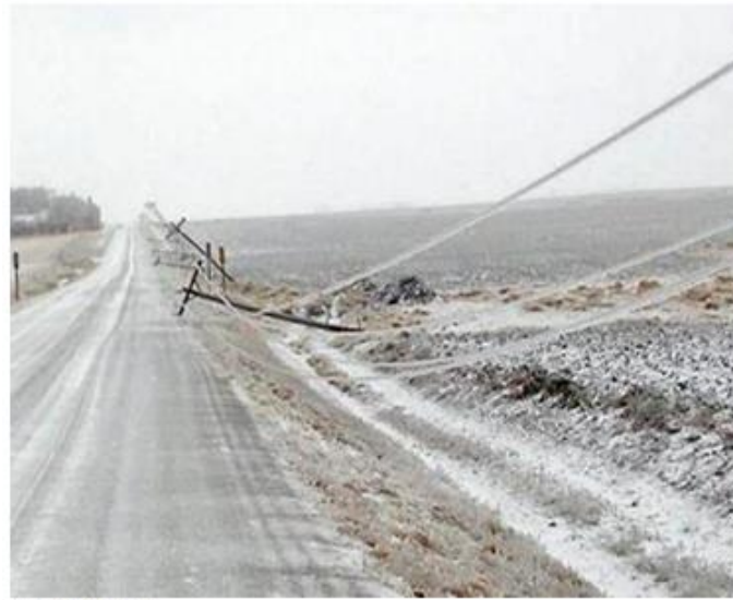
Figure #115 Downed Powerlines
