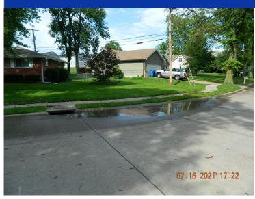
Stormwater runoff from the upper reaches of the drainage area flows south and ponds on a paved patio at 2706 Lakeport Drive and a flat or low-lying area at 2712 Lakeport Drive. There is minor yard rutting evident at the rear southeast corner of the property at 2715 Lakeport Drive. A portion of the surface drainage crosses the public sidewalk and flows onto Lakeport Drive before entering a curb inlet in front of 2712 Lakeport Drives and is considered a nuisance.
