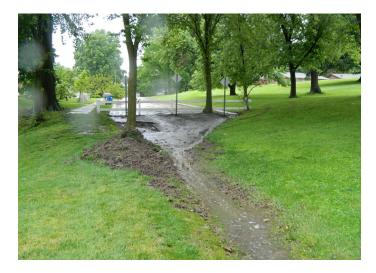
Drainage from Haas Avenue flows along a shallow swale/ berm within an unimproved portion of the roadway to an area inlet located just north of Essex Avenue. The underseepage has infiltrated the side slope of the berm on more than one occasion and flows to a residential structure at 11465 Essex Avenue. The owner reports that water frequently enters the basement through openings in the foundation.
