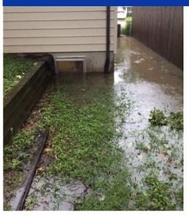
Stormwater runoff emanating from either (8) residential lots located north and east of this location flows to the rear of the property where it is impeded by physiclal barriers and the yard grade. The runoff is frequently excessive and has entered a rear basement window of the home on several occasions. There is minor yard erosion evident in some areas of the rear and side yard.
