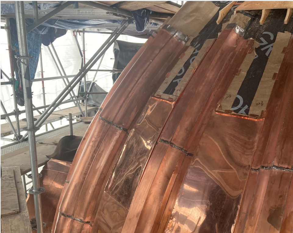
Below: Ribs of the dome are installed. Flat panels are located between each rib.
