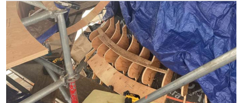
Below: wood blocking to support copper.
