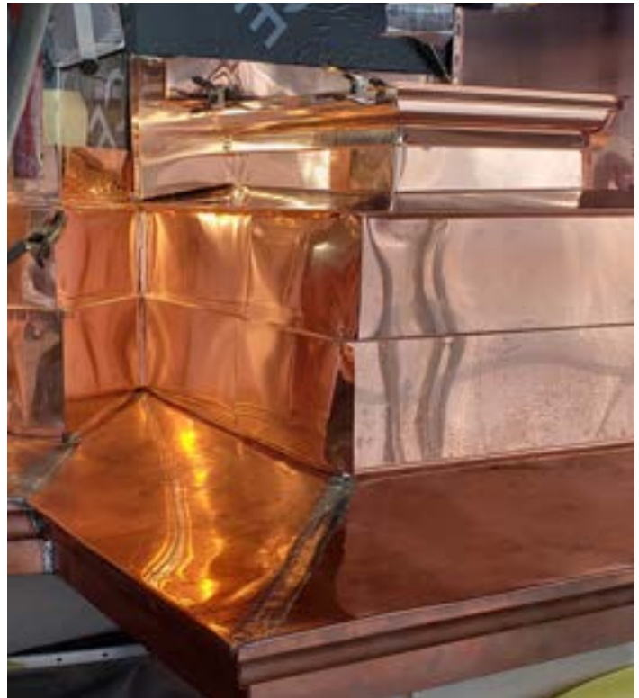
Copper work at the base of an eagle perch.
