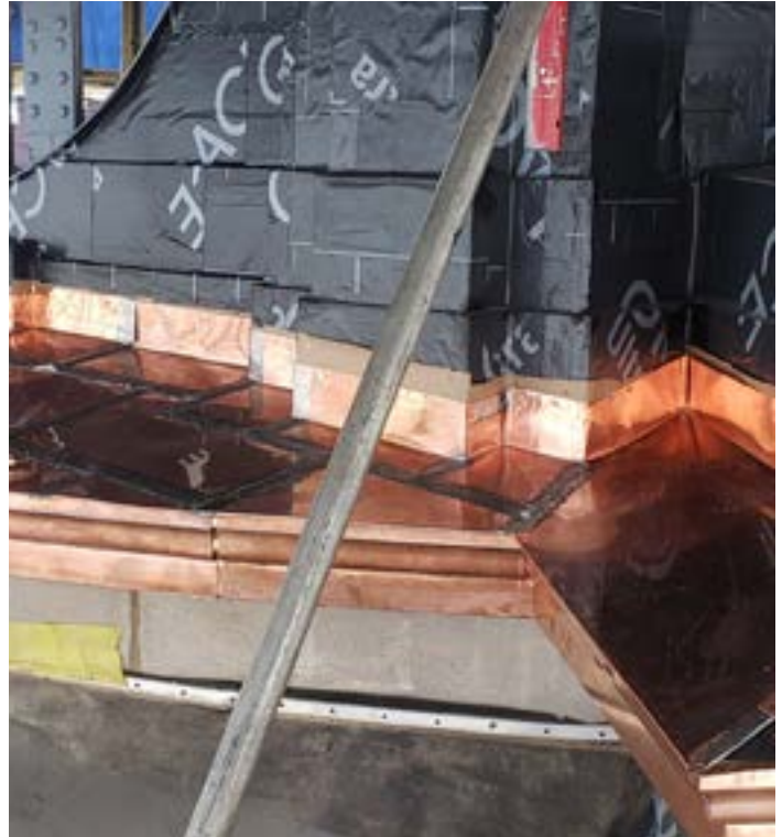
Vertical copper work installation.
