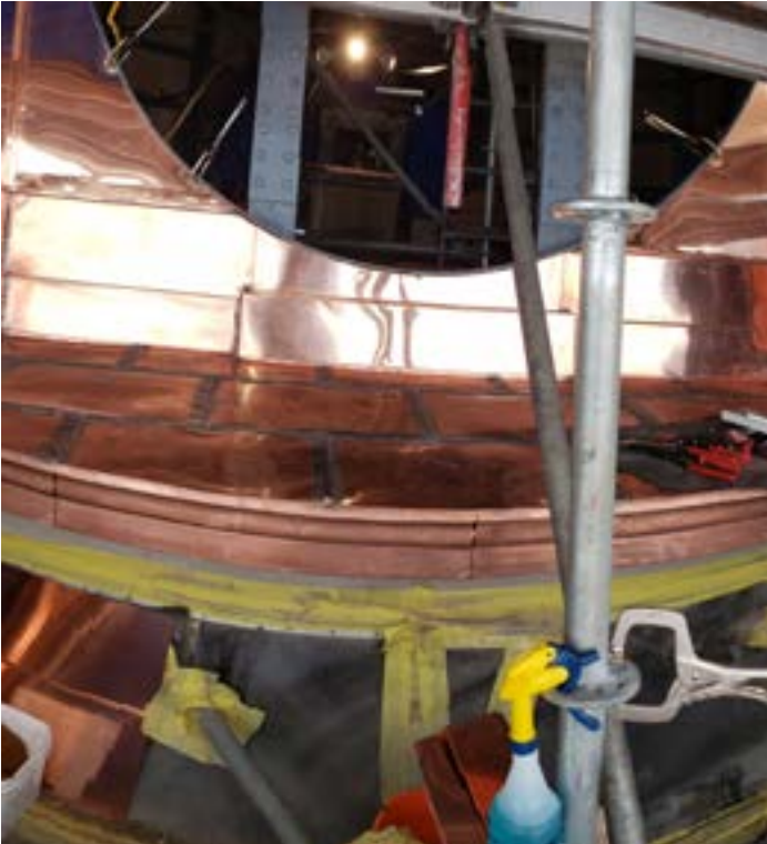
Copper work at the base of the clock dial.
