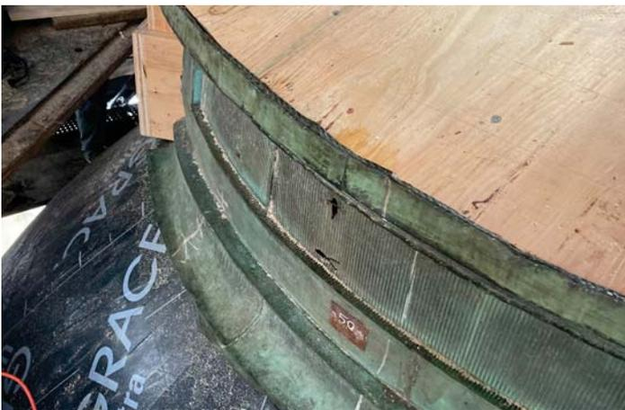
An original, single piece of copper used as a band around the dome.
