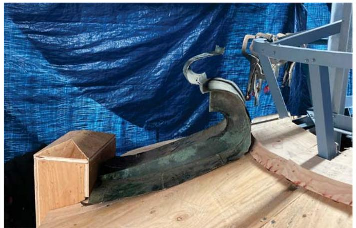
An original piece of copper used as a pattern at the base of the lantern.
