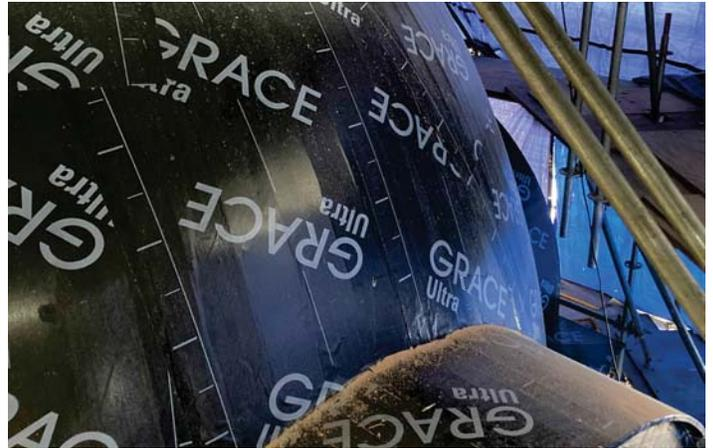
Ice and water shield applied to the dome exterior.
