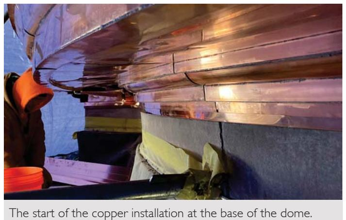
The start of the copper installation at the base of the dome.
