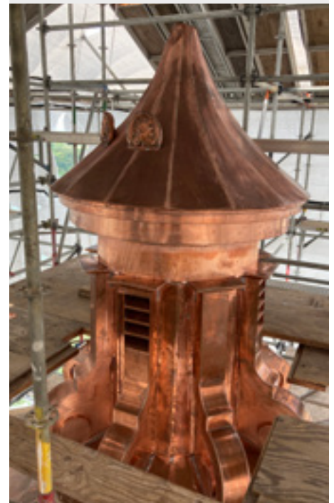
Top of the new copper dome lantern.
