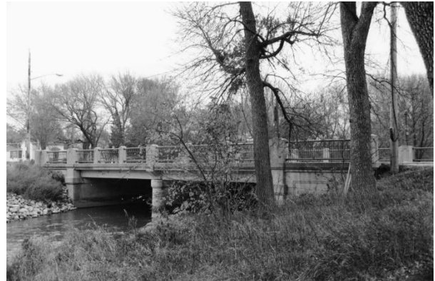
Bridge No. 5151 (Highway 19 Bridge over Redwood River)
