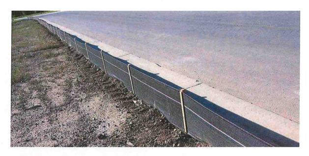
Silt fence, as shown in the detail drawings, must be installed properly to be effective. That means the bottom of the fence must be installed in a 6 inch deep trench and anchored with soil.
