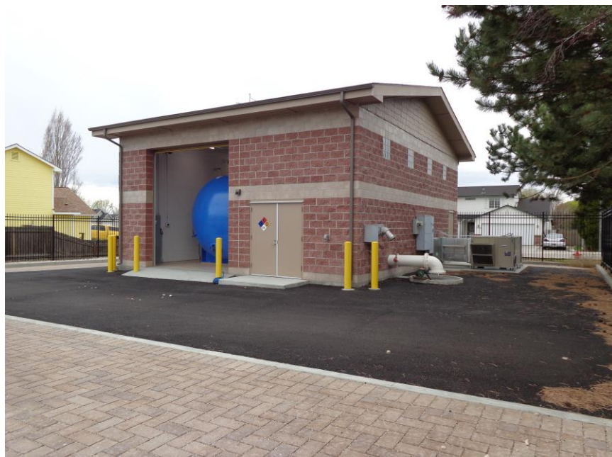
Figure 19: Manganese pressure filtration system inside concrete masonry unit (CMU) building.
