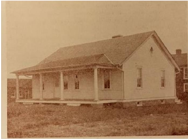
Figure 35. Available original photos of the Cottage show an unobstructed roof above the entrance.
