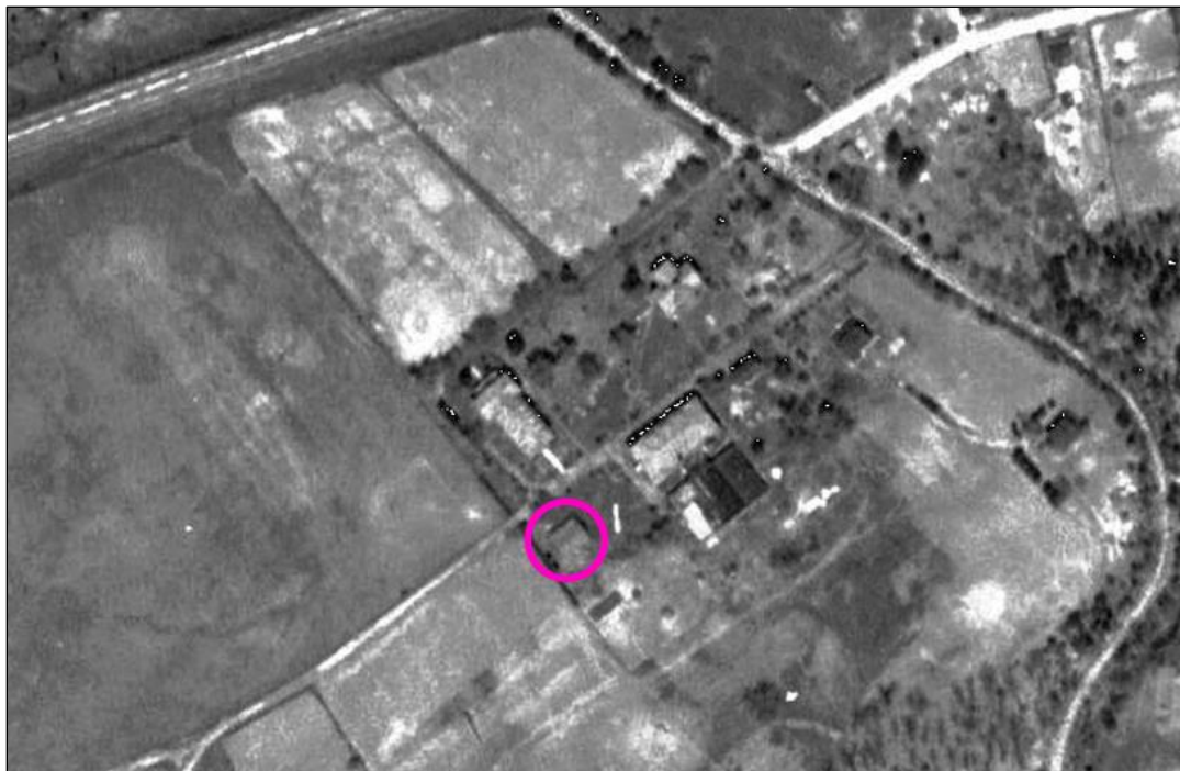
Figure 13: 1937 Aerial Image Showing the Three Main Buildings of the Campus (Prince William County 1937). The Cottage is located to the southwest of the H-shaped Carnegie Building as is in the pink circle.
