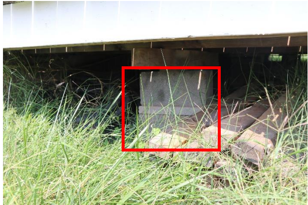
Figure 18. Intermediate CMU block piers supported the front porch joists (red box).
