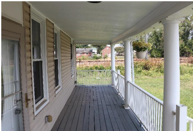
Figure 15. The front porch extended approximately 7-feet from the Cottage facade.
