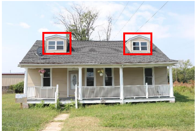
Figure 36. Two dormers (red boxes) are present on the Cottage entrance side roof slope.
