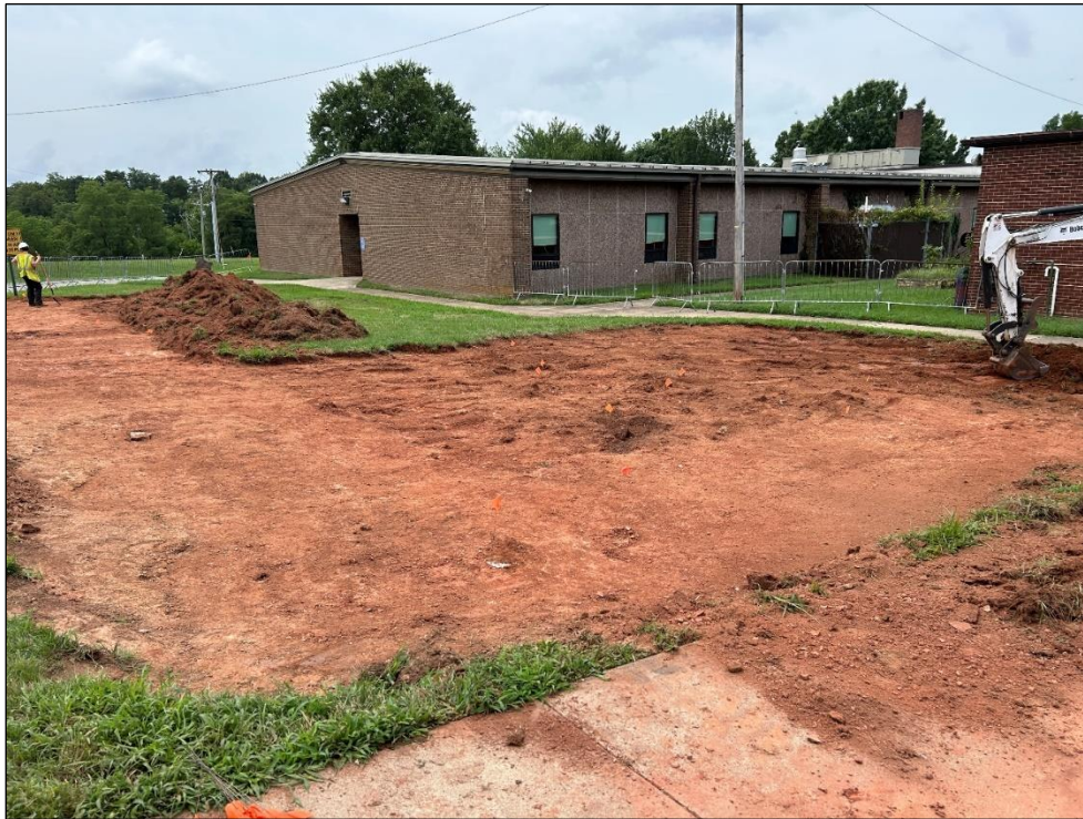
Photo 10: Stripped Area C in Progress, Facing Southwest.
