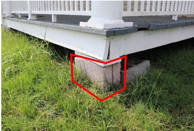
Figure 17. Hollow CMU blocks supported the porch columns (red box).
