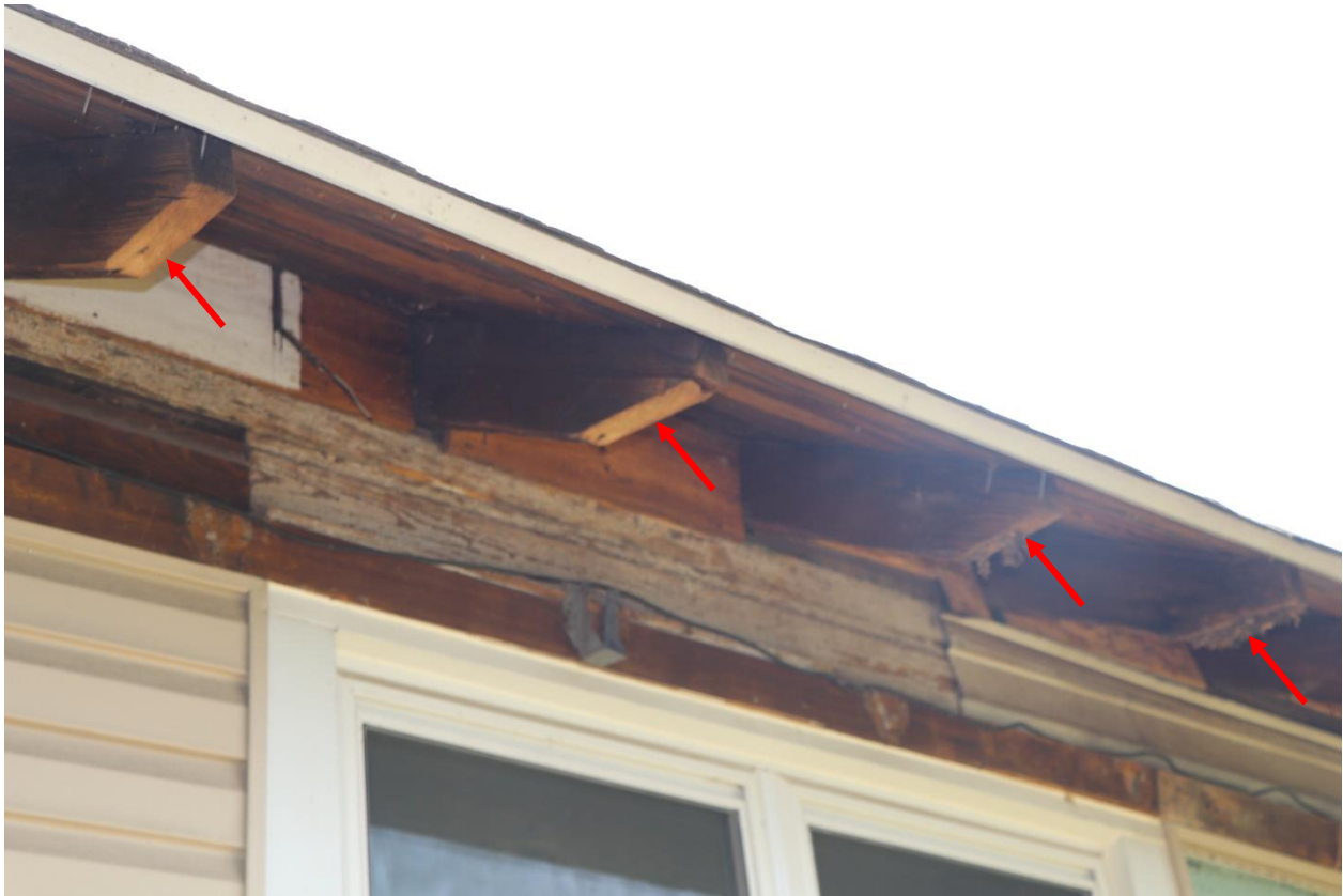
Figure 31. The roof rafters (red arrows) bear on the east-west perimeter walls.
