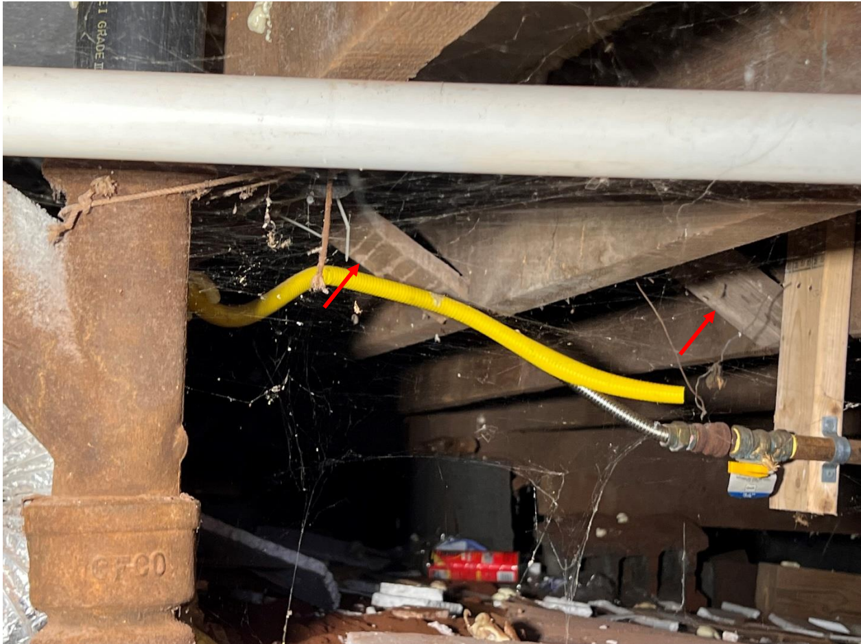
Figure 25. WJE observed wood blocking (red arrows) between the First Level floor joists.
