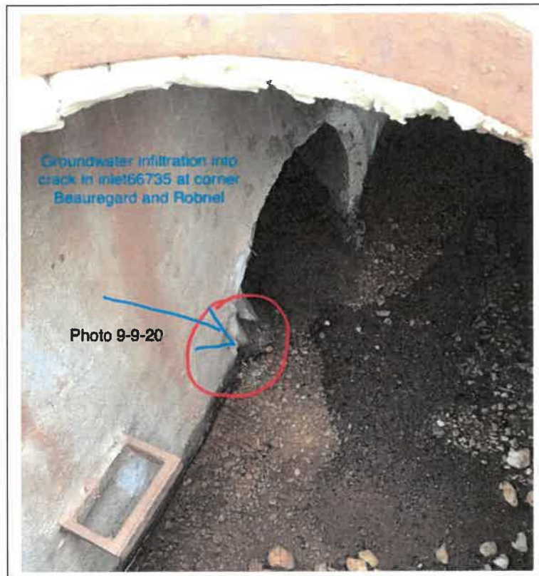
Figure 7 The source of water coming out of outfall #59900
