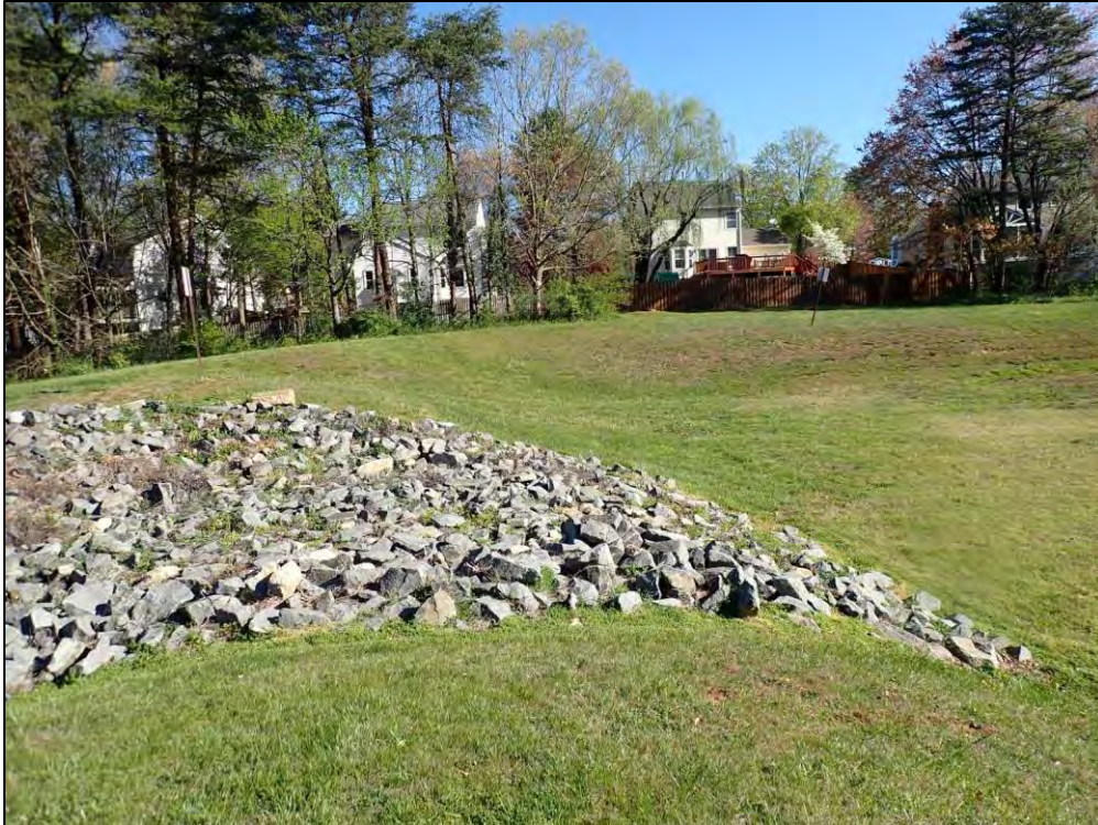
9309: Emergency Spillway, Overall. Shrubby, low-growing vegetation, and/or vine material growing on the embankment (Monitor).
