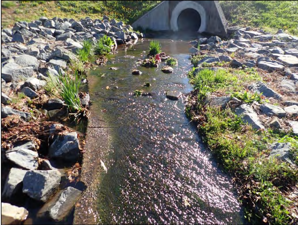
9326: From the Trickle Ditch, looking upstream toward Inflow Structure D5. The low-flow ditch is clogged with sediment/debris (Monitor).
