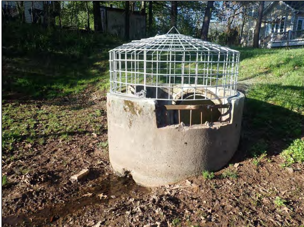
9262: Control Structure B2, front. Buildup of trash, debris, and sediment (Routine Maintenance Needed).
