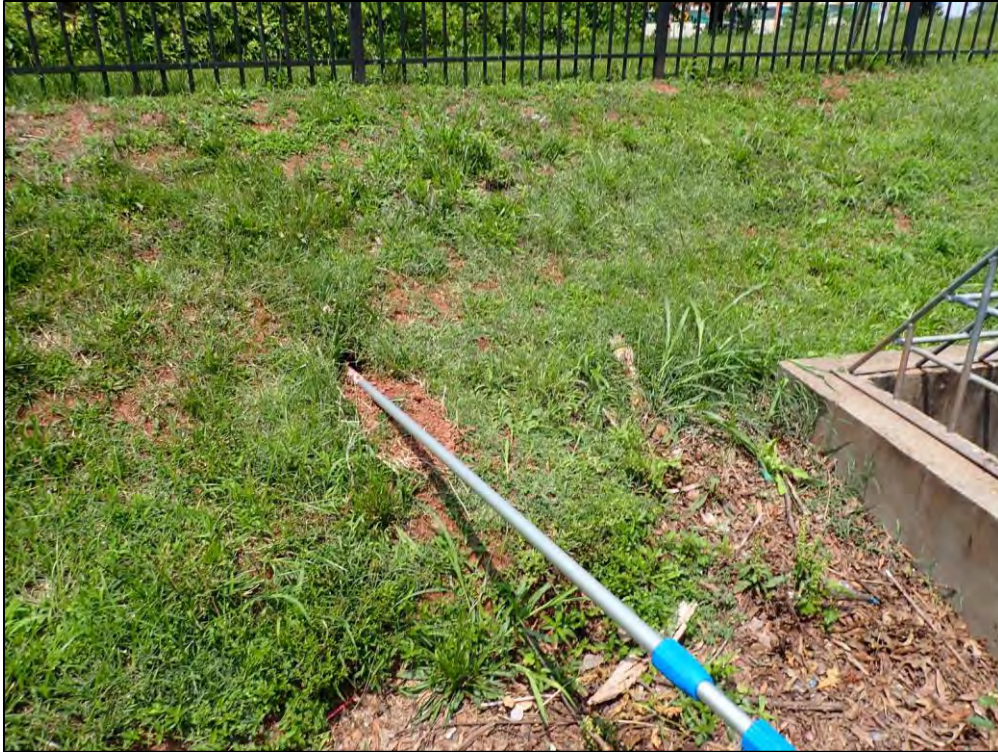
4788: Animal hole, overall. Evidence of nuisance animals (Immediate Repair Needed).
