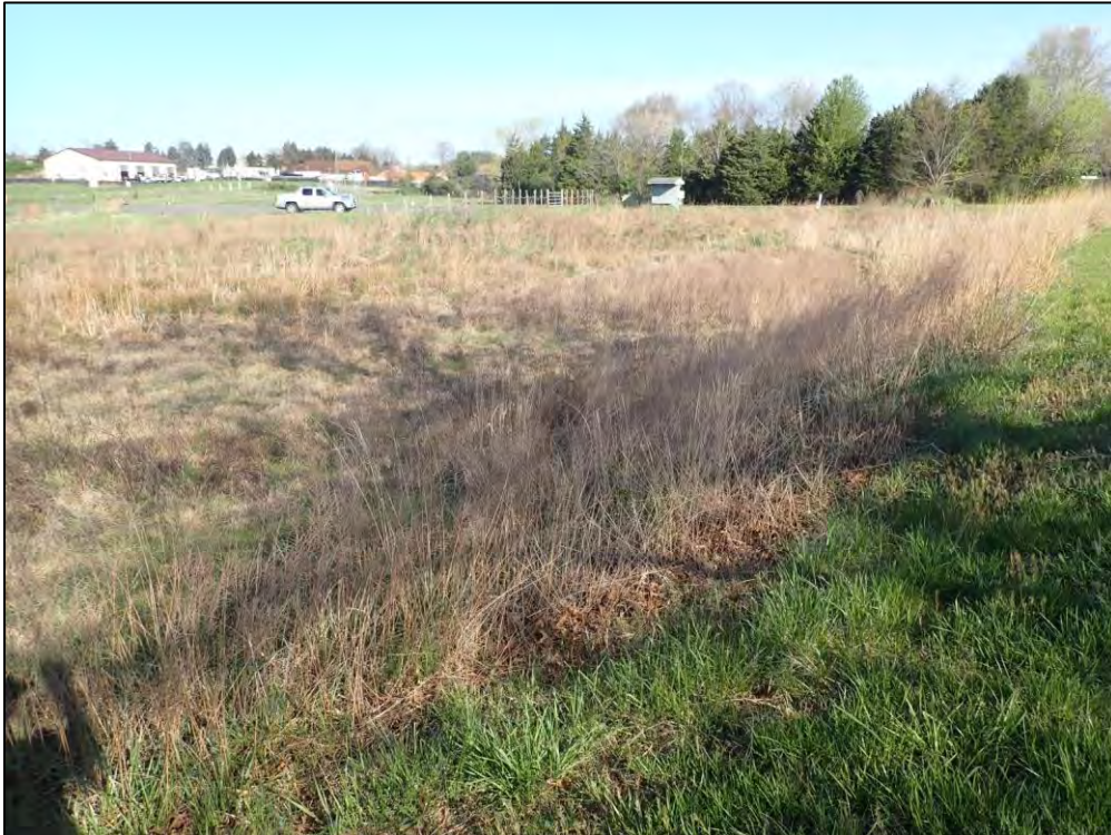
2723: Facility Overall. Overgrown vegetation was observed on the pond floor (Routine Maintenance Needed).
