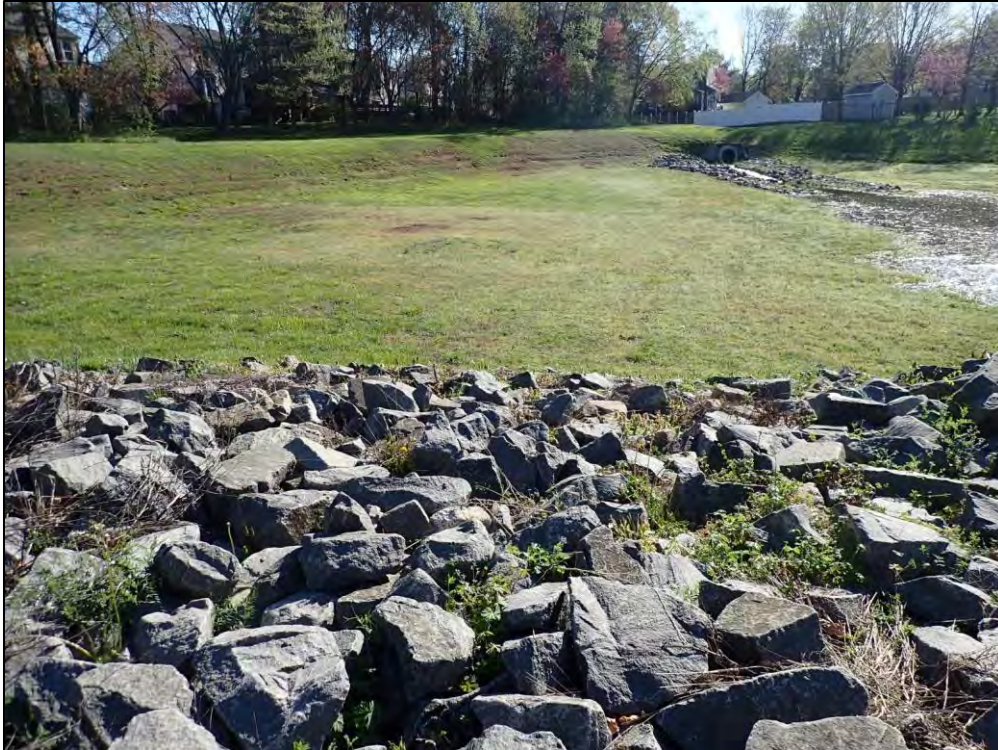
9311: From the Emergency Spillway, looking upstream. Shrubbery, low-growing vegetation, and/or vine material growing on the embankment (Monitor).
