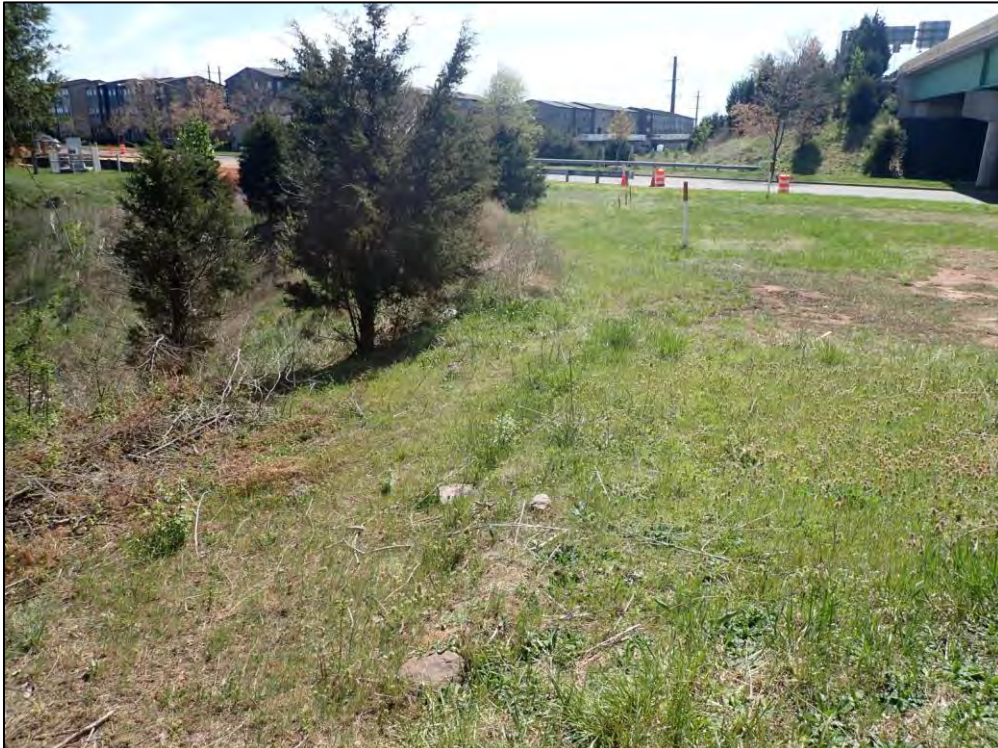
2768: Dam overall. Woody vegetation on the embankment (Routine Maintenance Needed).
