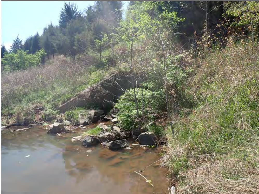
2812: Inflow 10, overall. Woody growth around inlet structure (Routine Maintenance Needed).
