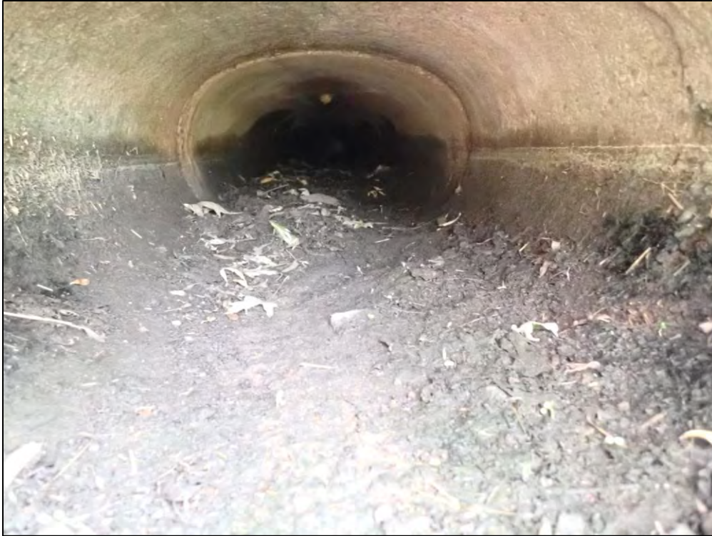
4738: Inside Inflow Structure D1. Buildup of trash, debris, and sediment (Routine Maintenance Needed).
