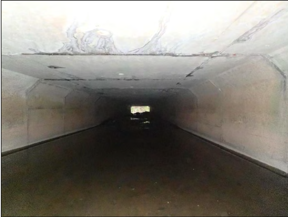
2781: Inside Inflow 4, looking along the Northern pipe. Buildup of trash, debris, and sediment (Routine Maintenance Needed).
