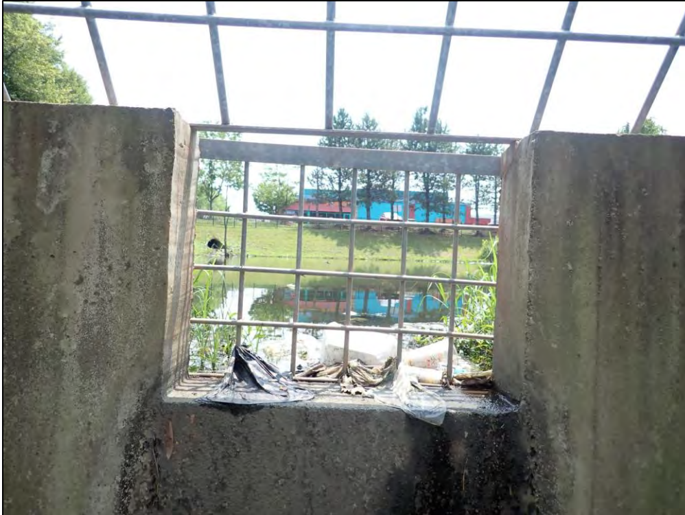
4778: Inside Control Structure 37, looking upstream toward the upper orifice. Trash, debris, or other material in BMP device (Routine Maintenance Needed).
