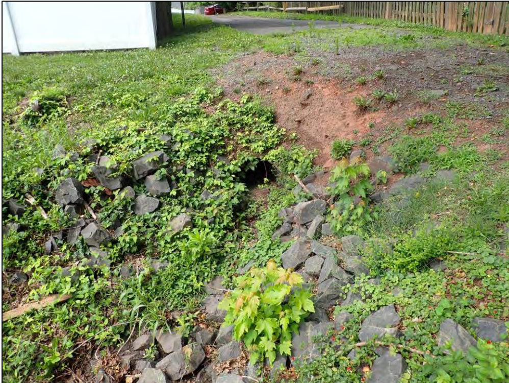
4750: Inflow Structure A1, front. Sparse vegetative coverage (Monitor).
