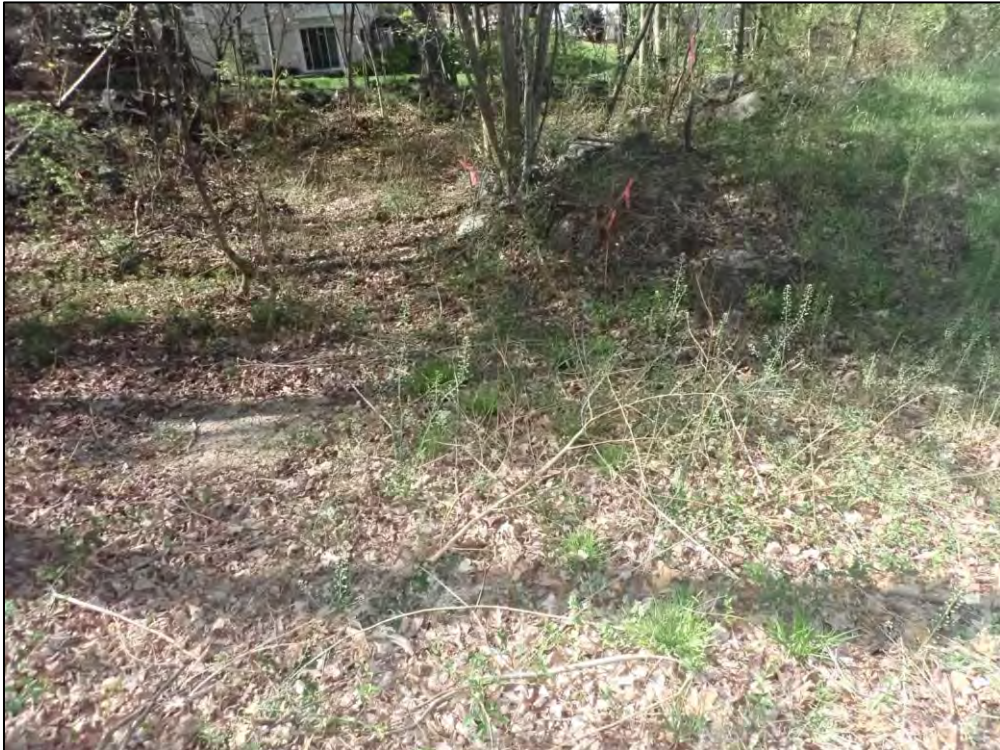
9356: Emergency Spillway, Overall. Woody vegetation on the embankment (Routine Maintenance Needed).
