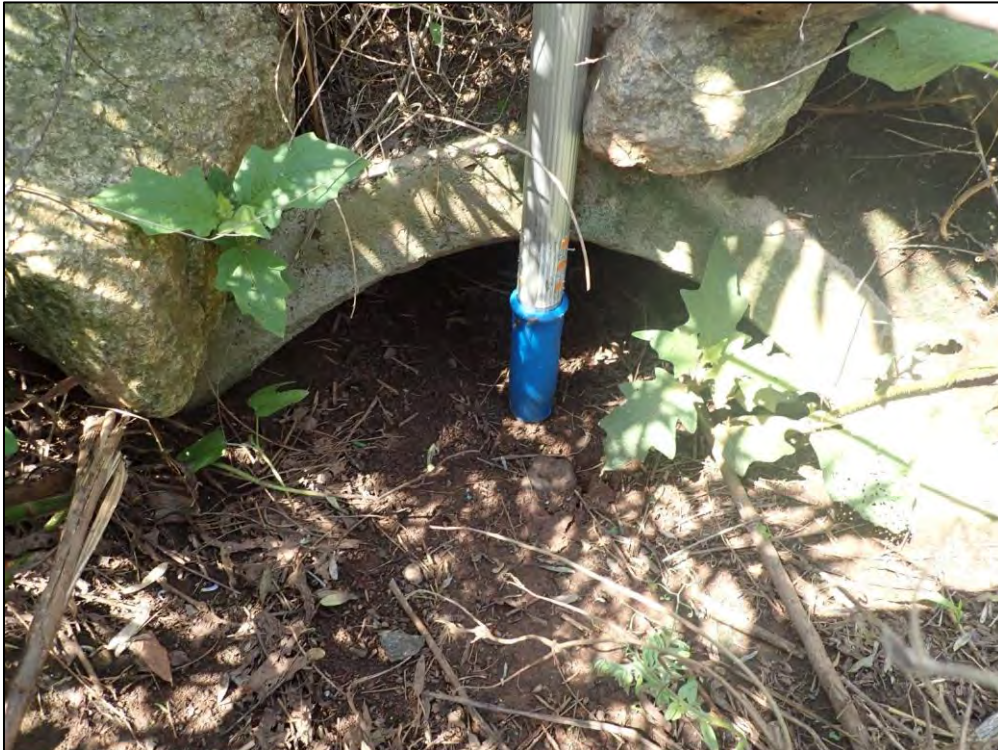
4464: Inflow Structure 3A, closeup. Buildup of trash, debris, and sediment (Immediate Repair Needed).
