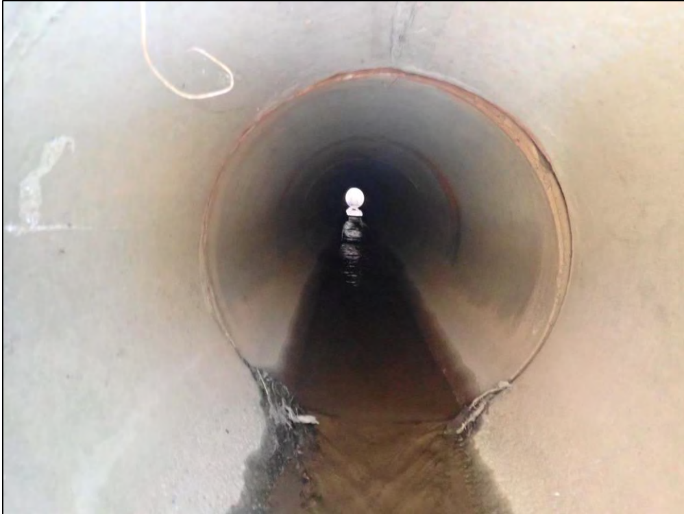
9347: Inside the Outfall. The outfall structure has separated from the principal spillway barrel (Routine Maintenance Needed).
