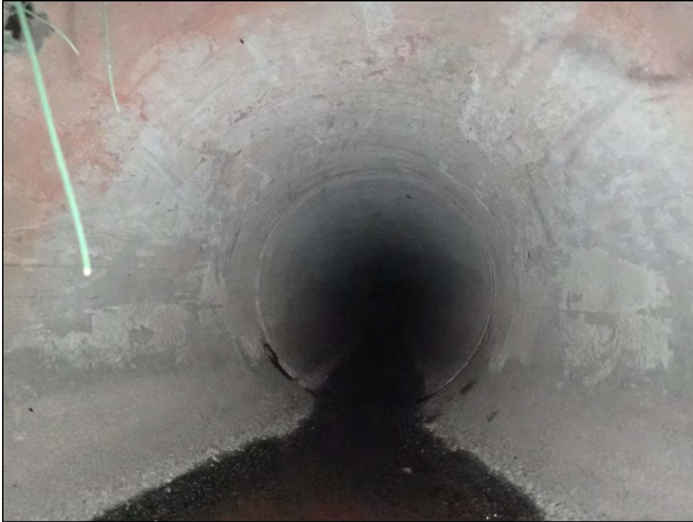
2818: Inside the Outfall. Damage to inlet pipe or structure (Routine Maintenance Needed).
