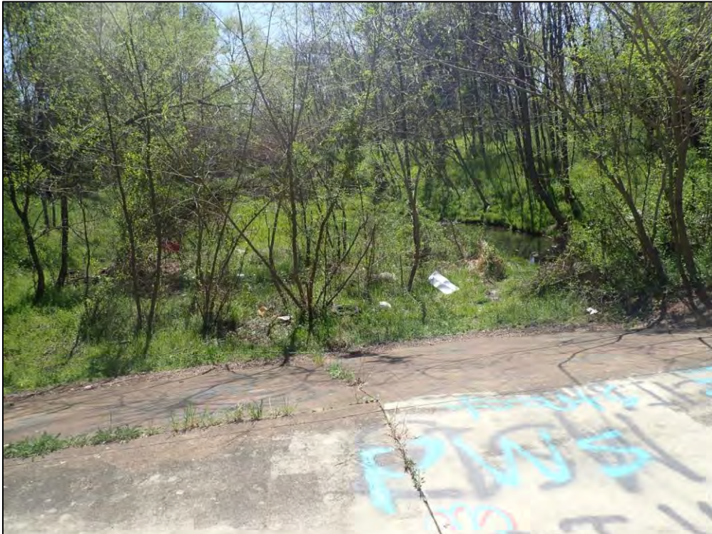
2847: Looking downstream along the Emergency Spillway. Woody vegetation on the embankment (Routine Maintenance Needed).
