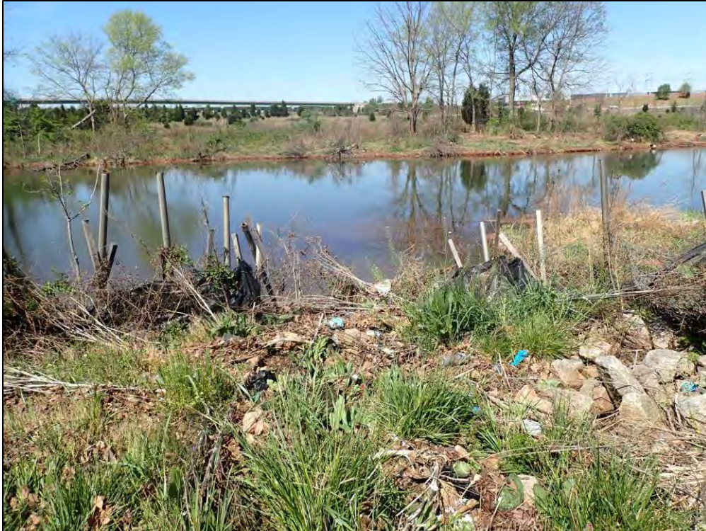
2777: Inflow 3, downstream. Buildup of trash, debris, and sediment (Routine Maintenance Needed).
