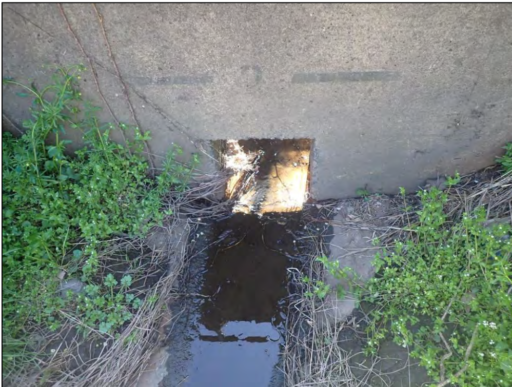
2837: Control Structure 3, low-flow orifice close-up. BMP Orifice Plate is missing (Immediate Repair Needed).
