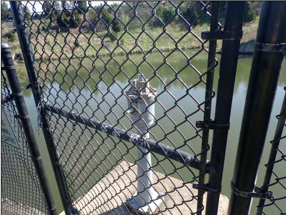
2759: Control Structure, closeup of the Dewatering Valve Apparatus.
