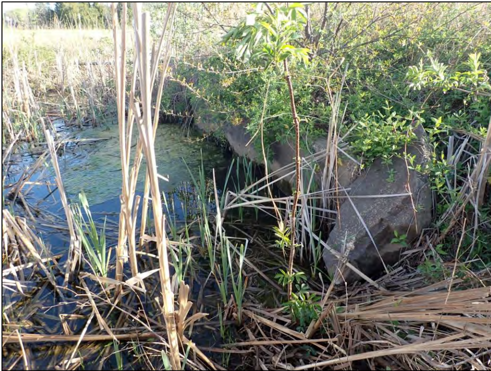
2698: Outfall, Overall. Woody vegetation growing within 5' of outlet and barrel (Immediate Repair Needed).
