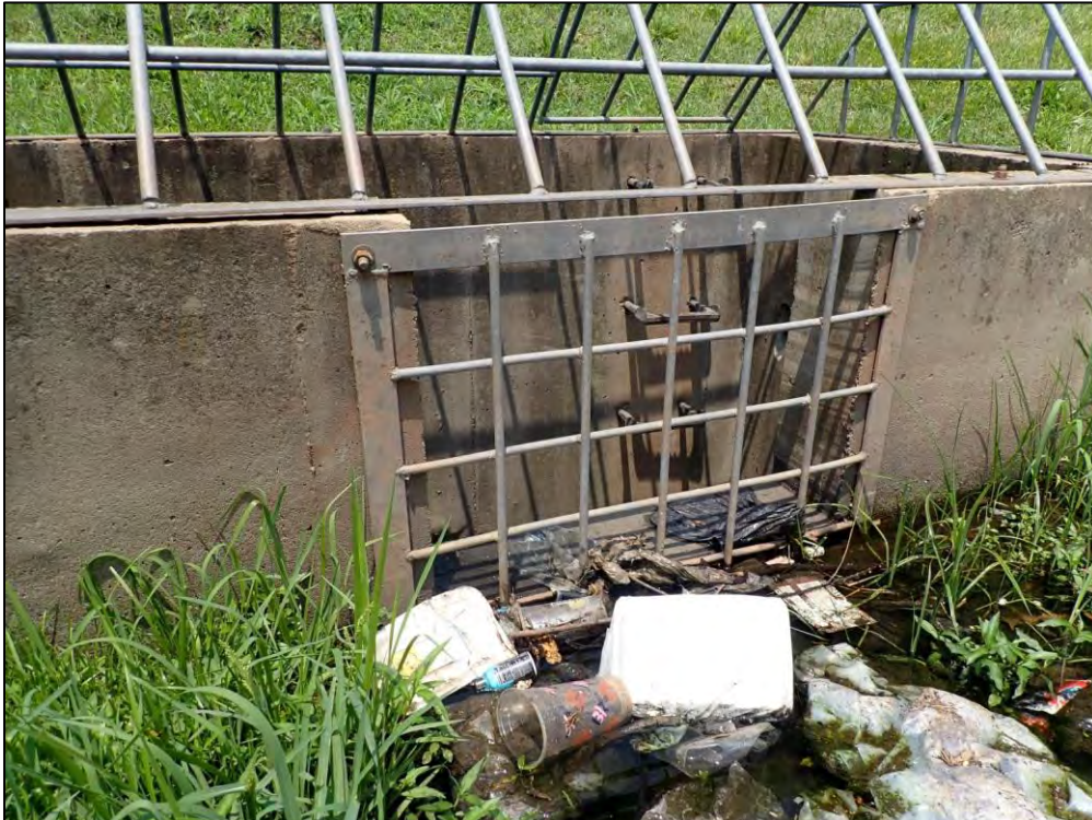
4775: Control Structure 37, overall looking toward the upper orifice. Trash, debris, or other material in BMP device (Routine Maintenance Needed).
