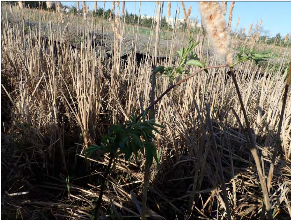
2700: From the Outfall, looking downstream. Overgrown vegetation was observed on the pond floor (Routine Maintenance Needed).
