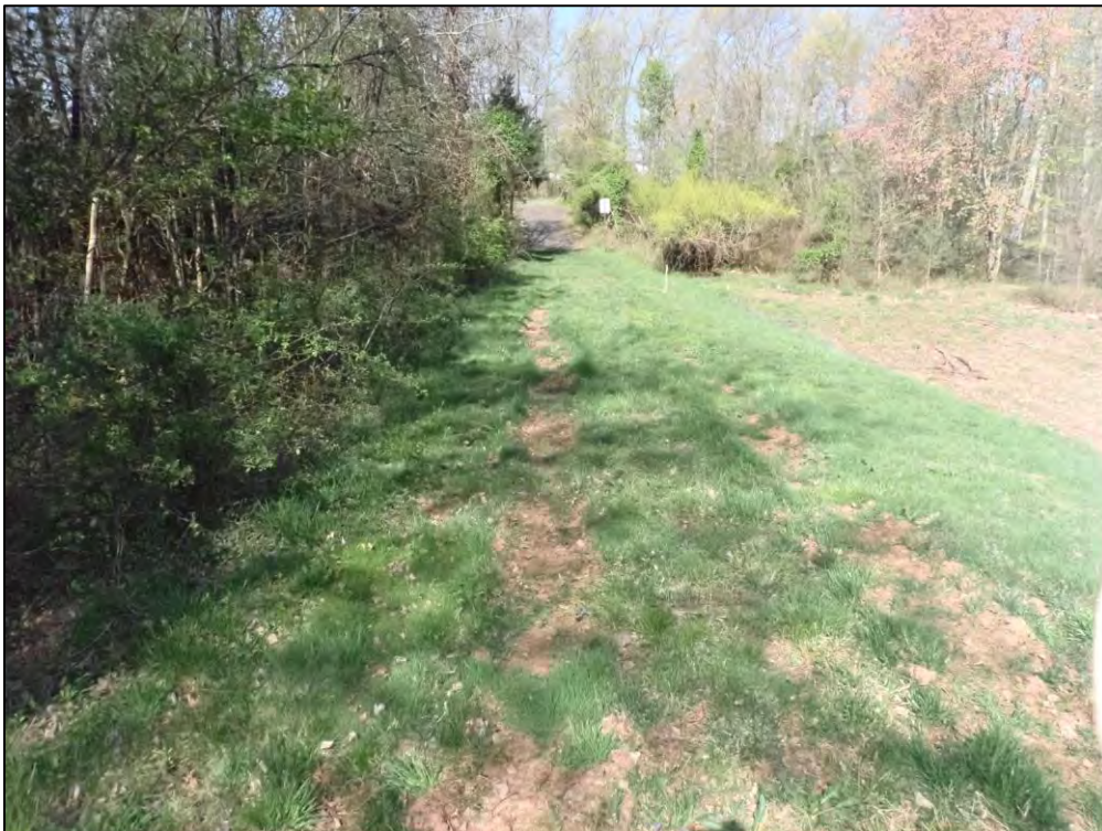
9350: Dam, Overall. Sparse vegetative coverage (Monitor).
