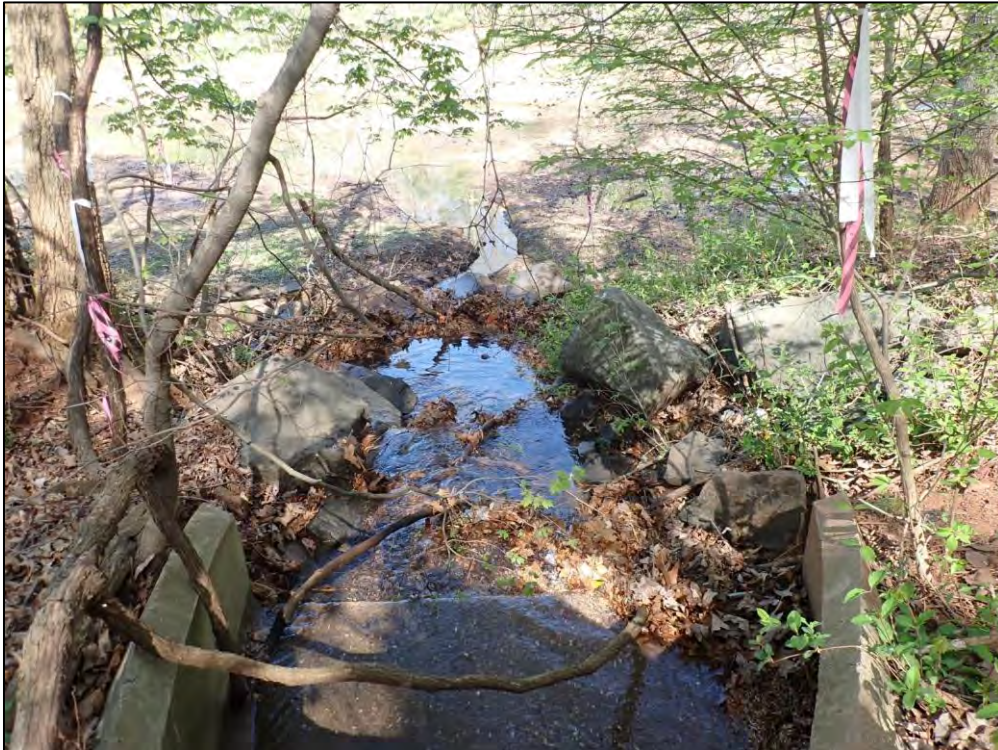
9374: From Inflow Structure D1, looking downstream. Buildup of trash, debris, and sediment (Monitor).
