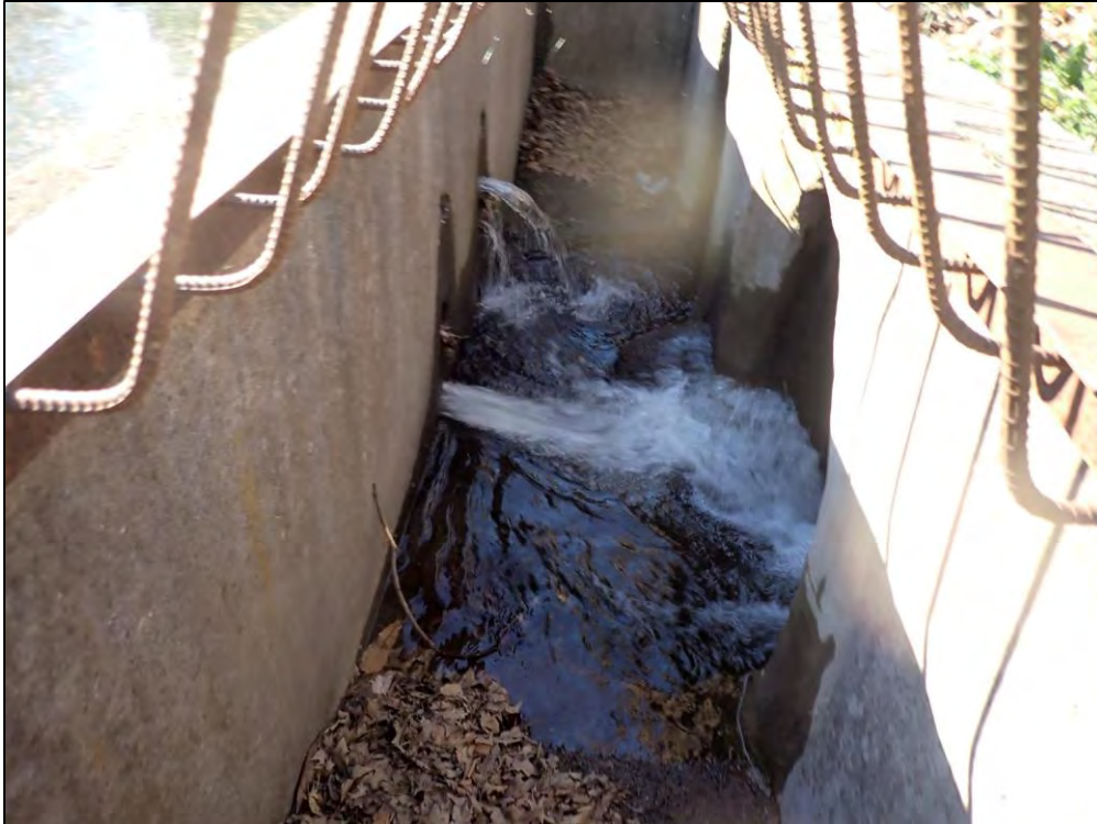
9301: Inside Control Structure D4. The low-flow orifices are blocked (Immediate Repair Needed).
