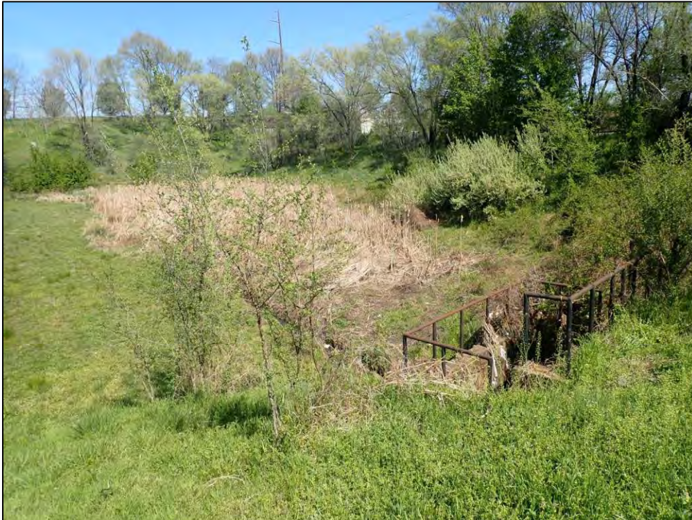
2861: Facility Overall. The ponding area is showing signs of poor health (i.e. nutrient overload, excess aquatic vegetation, or turbidity) (Routine Maintenance Needed).
