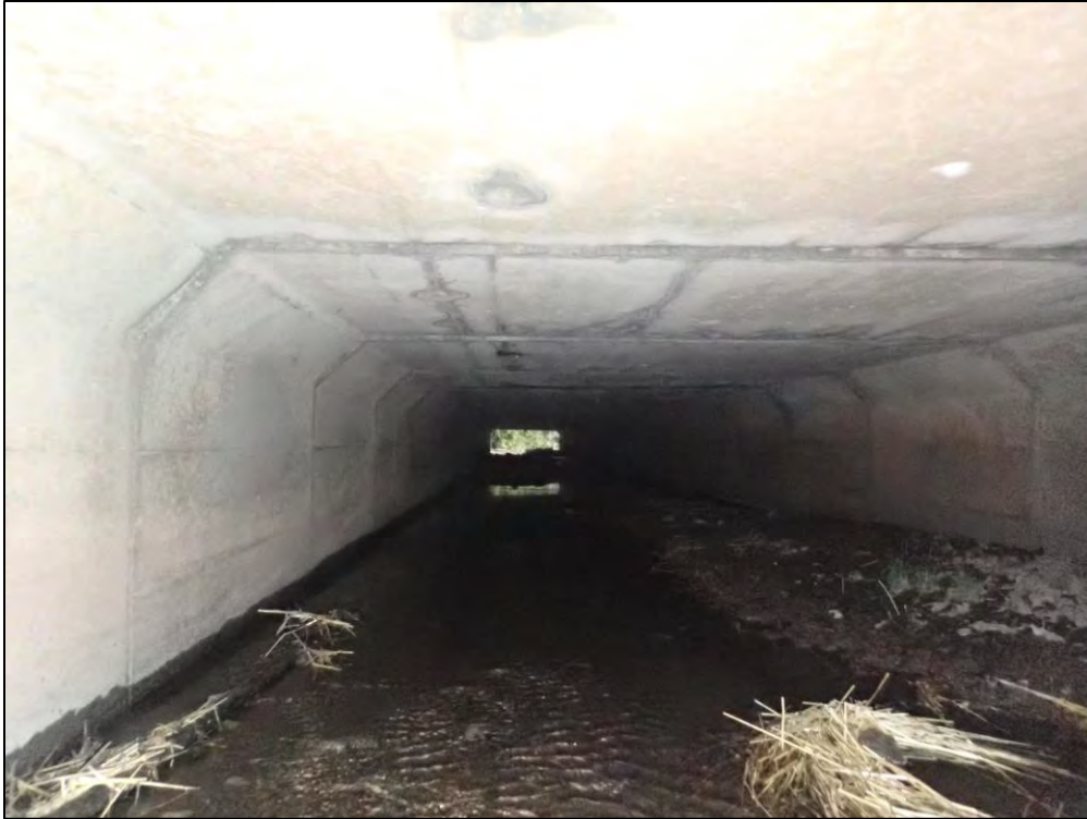
2783: Inside Inflow 4, looking along the Southern pipe. Buildup of trash, debris, and sediment (Immediate Repair Needed).
