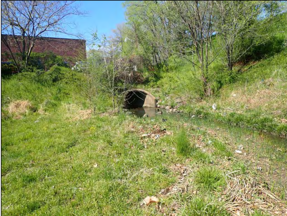
2854: Inflow Structure 2, Overall. Buildup of trash, debris, and sediment (Monitor).
