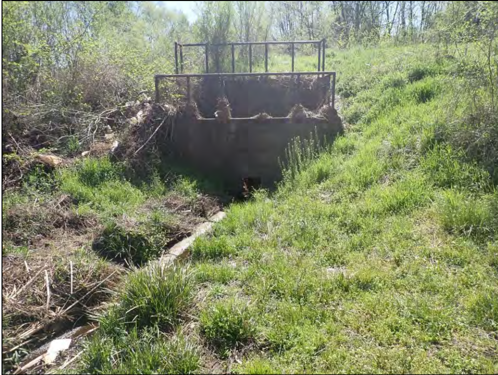
2836: Control Structure 3, front. Trash, debris, or other material in BMP device (Routine Maintenance Needed).
