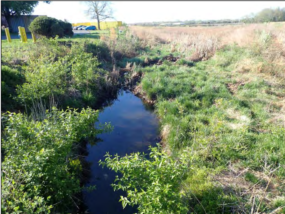
2719: From Inflow Structure D9, looking downstream. Overgrown vegetation was observed on the pond floor (Routine Maintenance Needed).
