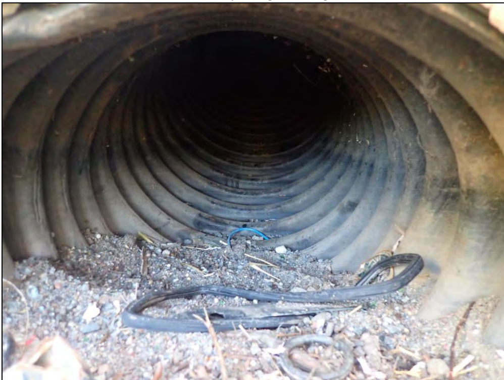
2755: Inside Inflow 4. Buildup of trash, debris, and sediment (Routine Maintenance Needed). Woody growth around inlet structure, Non-woody overgrown veg. (Routine Maintenance Needed).
