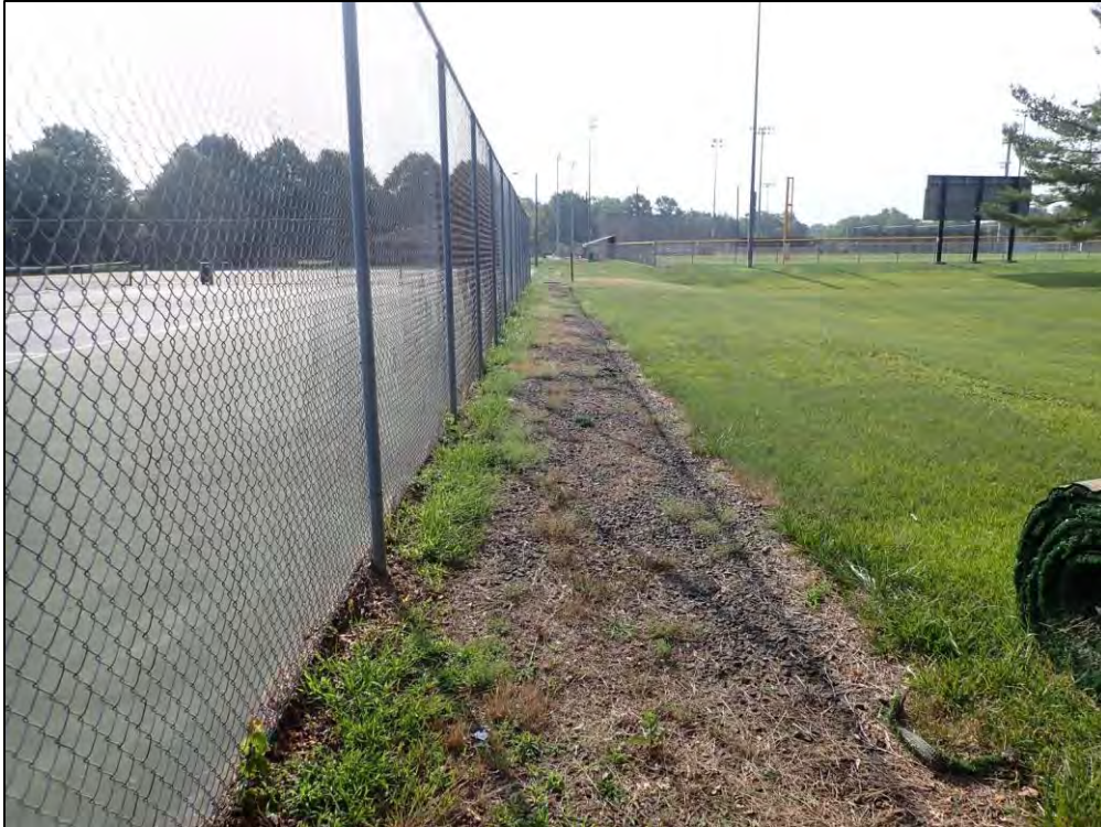
4590: Infiltration Trench Surface. Overgrown Vegetation Present (Immediate Repair Needed).
