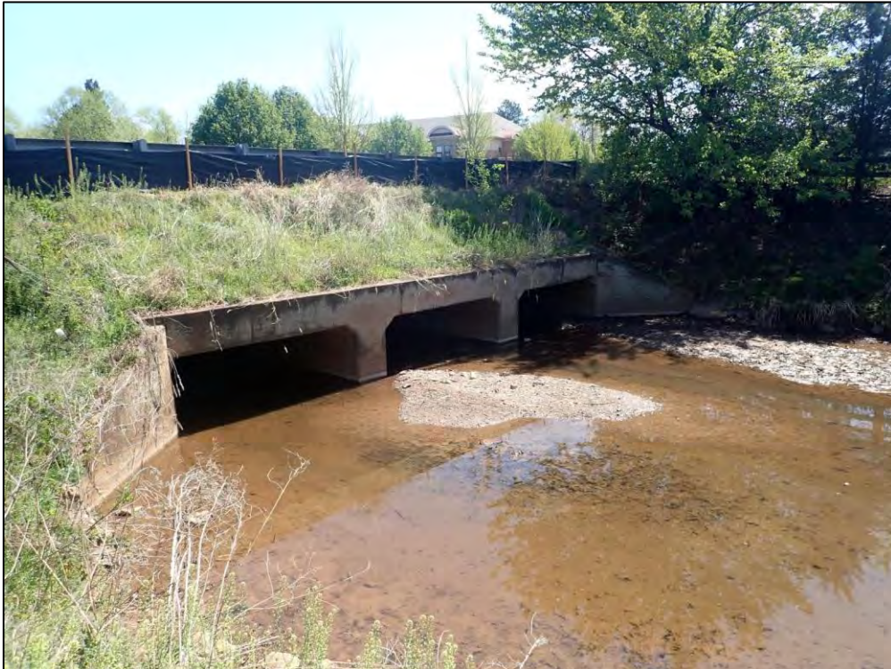
2780: Inflow 4, front. Buildup of trash, debris, and sediment (Routine Maintenance Needed).
