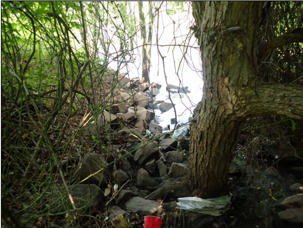
4793: From Inflow Structure 1, looking downstream. Woody growth around inlet structure (Routine Maintenance Needed).
