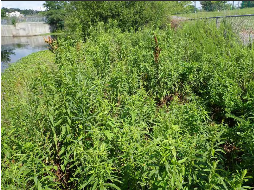
4448: Inflow 1, Overall. Woody growth around inflow structure (Immediate Repair Needed).
