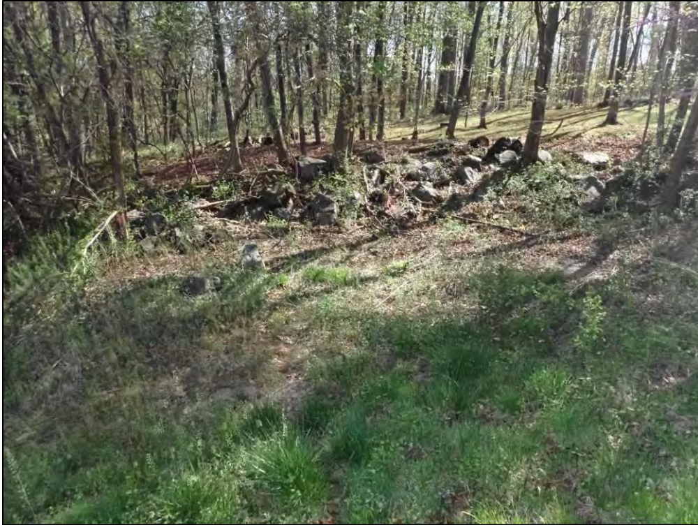
9355: Emergency Spillway, Overall. Woody vegetation on the embankment (Routine Maintenance Needed).
