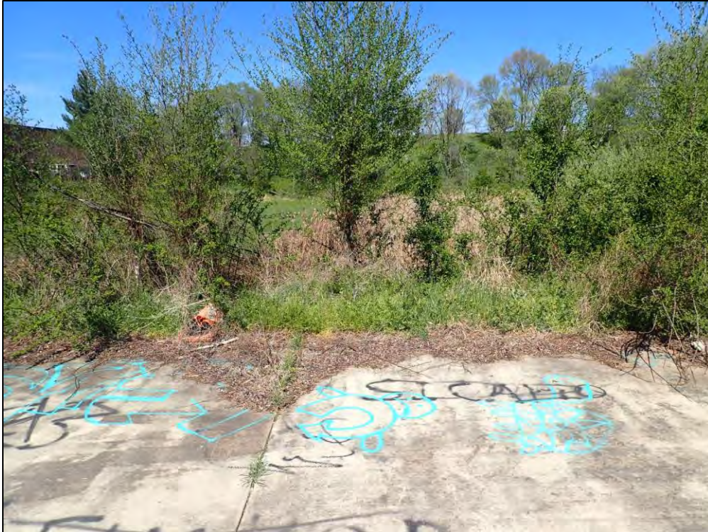
2846: Looking upstream along the Emergency Spillway. Woody vegetation on the embankment (Routine Maintenance Needed).
