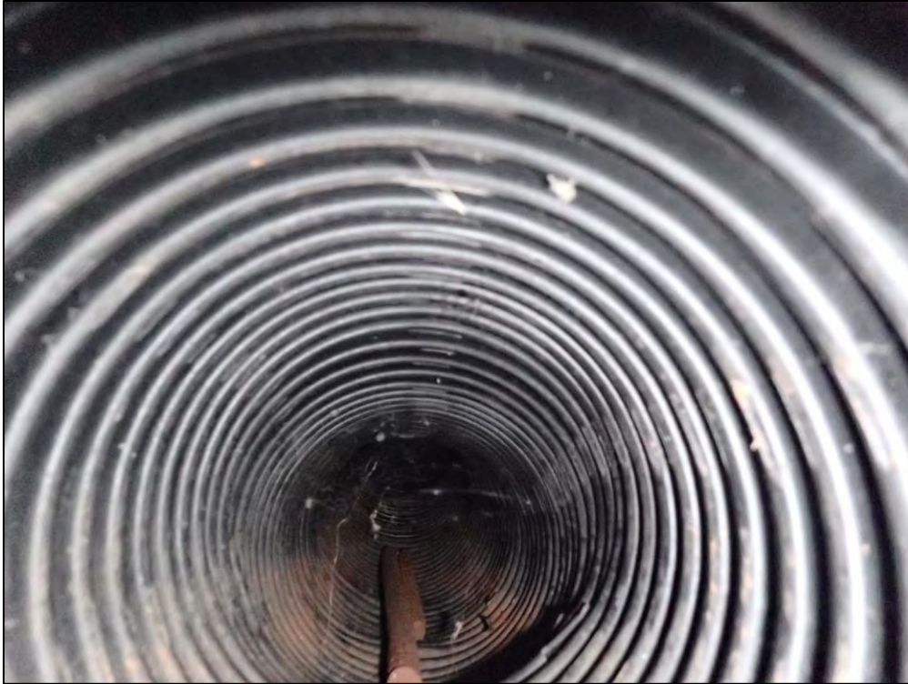
4600: Inside Control Structure I-29-017, looking upstream along the Northern underdrain. Debris observed within the underdrain (Immediate Repair Needed).
