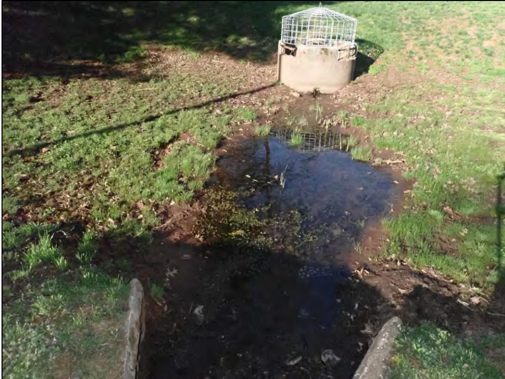
9284: From Inflow Structure A1, looking downstream. Buildup of trash, debris, and sediment (Monitor).
