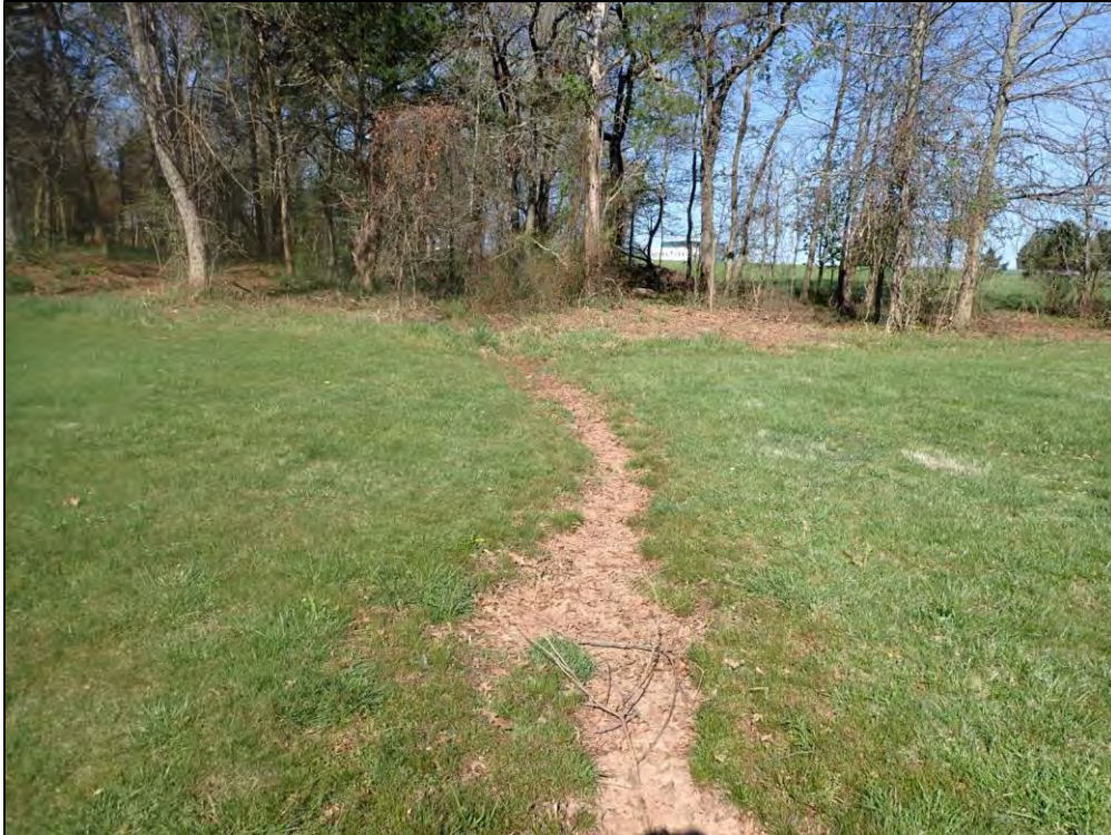
2739: Looking upstream along Inflow 1. Evidence of erosion or undermining around inlet (Routine Maintenance Needed).
