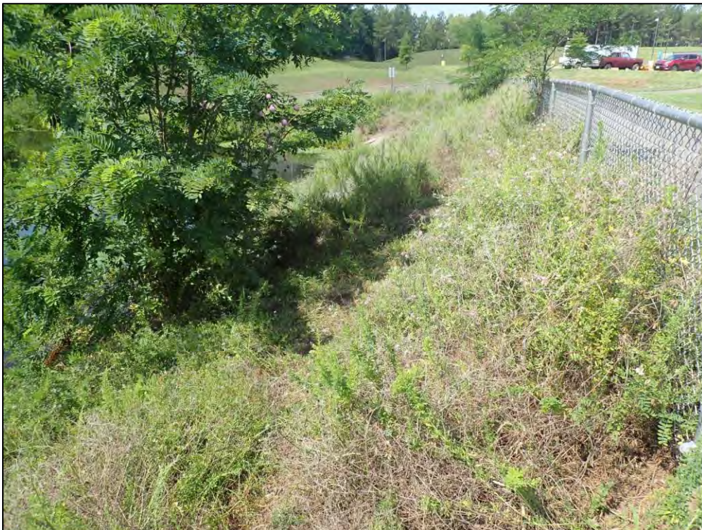
4431: Dam Overall, front slope. Shrubbery, low-growing vegetation, and/or vine material growing on the embankment (Routine Maintenance Needed).
