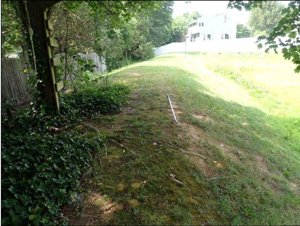
4736: Dam Overall. Sparse vegetative coverage (Monitor).
