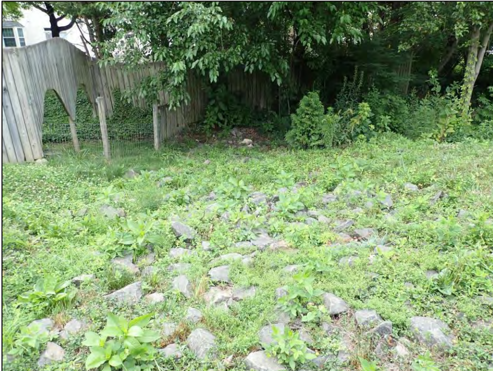
4735: Looking downstream along the Emergency Spillway. Shrubbery, low-growing vegetation, and/or vine material growing on the embankment (Routine Maintenance Needed).
