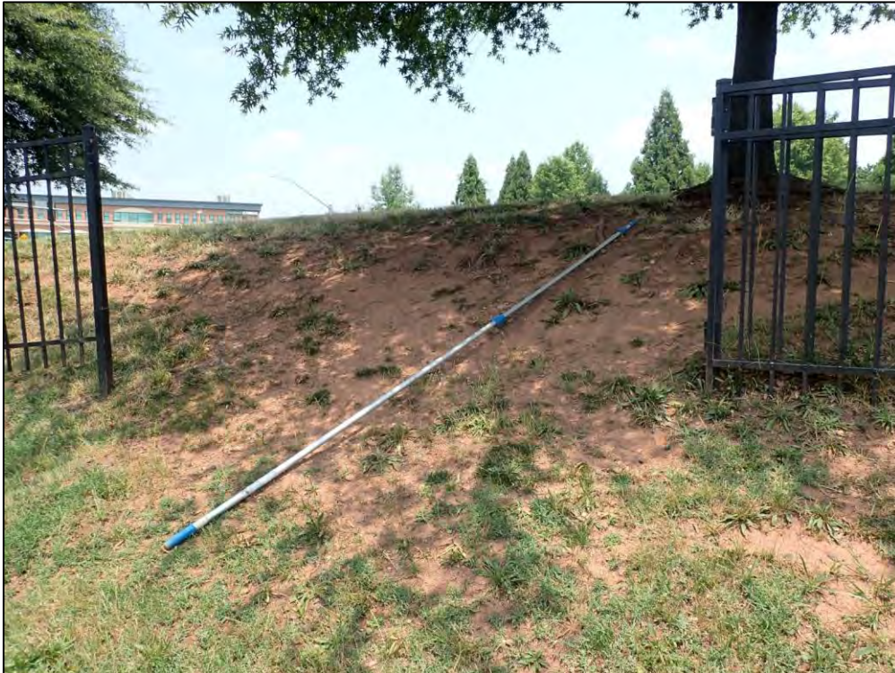
4771: Impoundment Area, Overall. Sparse vegetation or erosion (Routine Maintenance Needed).
