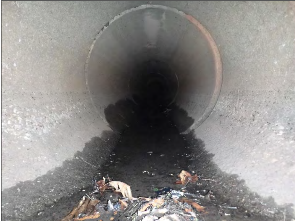
9283: Inside Inflow Structure A1. Joint Separation (Routine Maintenance Needed).
