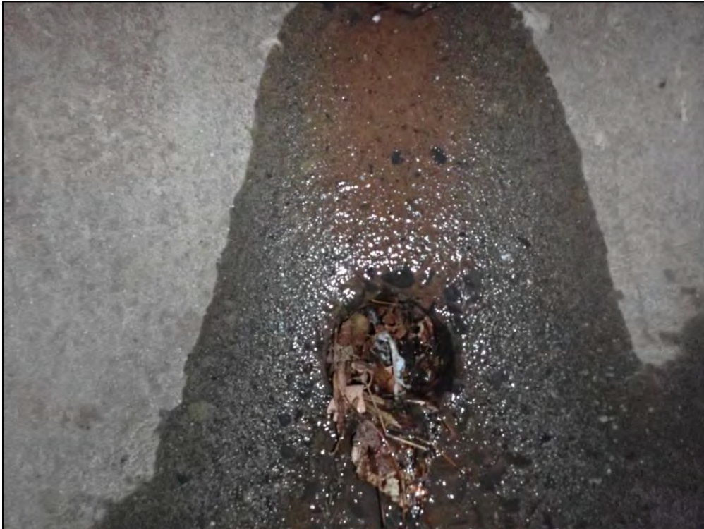
9294: Inside Control Structure D4, looking upstream toward the low-flow orifices. The low-flow orifices are blocked (Immediate Repair Needed).
