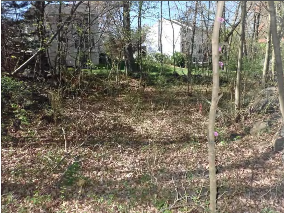
9358: Looking downstream along the Emergency Spillway. Woody vegetation on the embankment (Routine Maintenance Needed).
