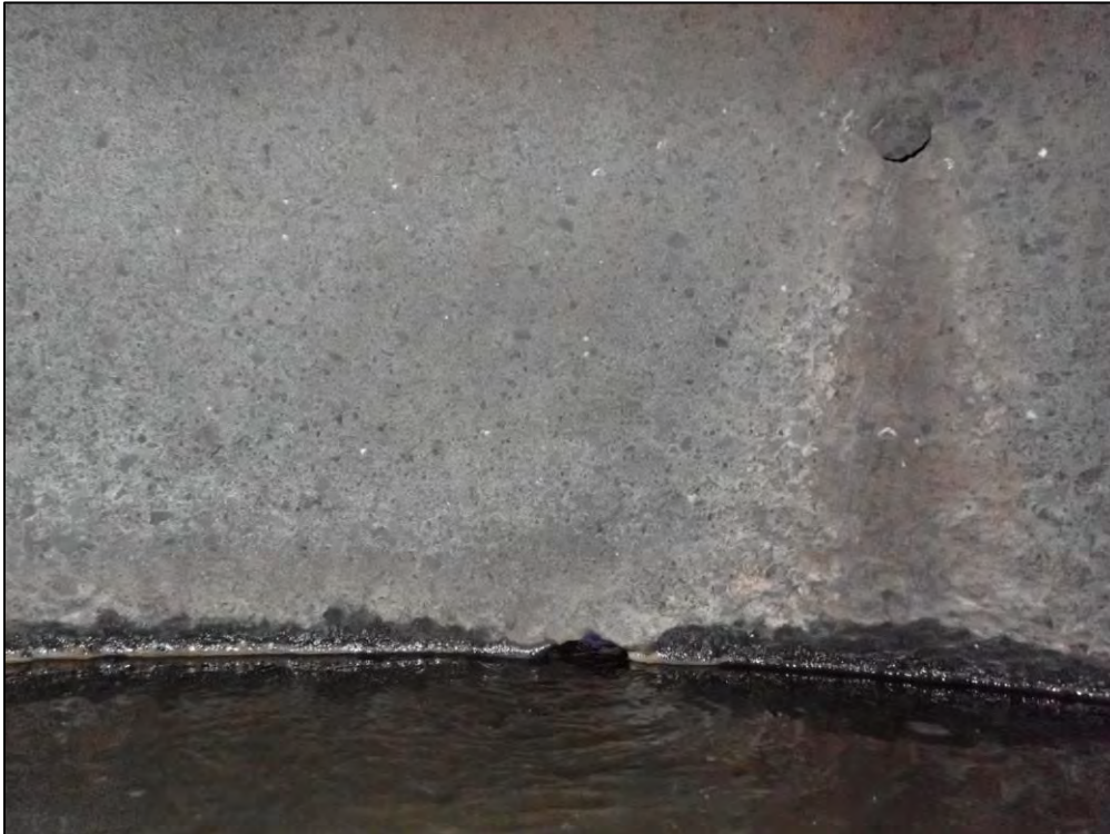
9342: Inside Control Structure, looking upstream toward the Northern low-flow orifice. The low-flow orifice is blocked (Immediate Repair Needed).
