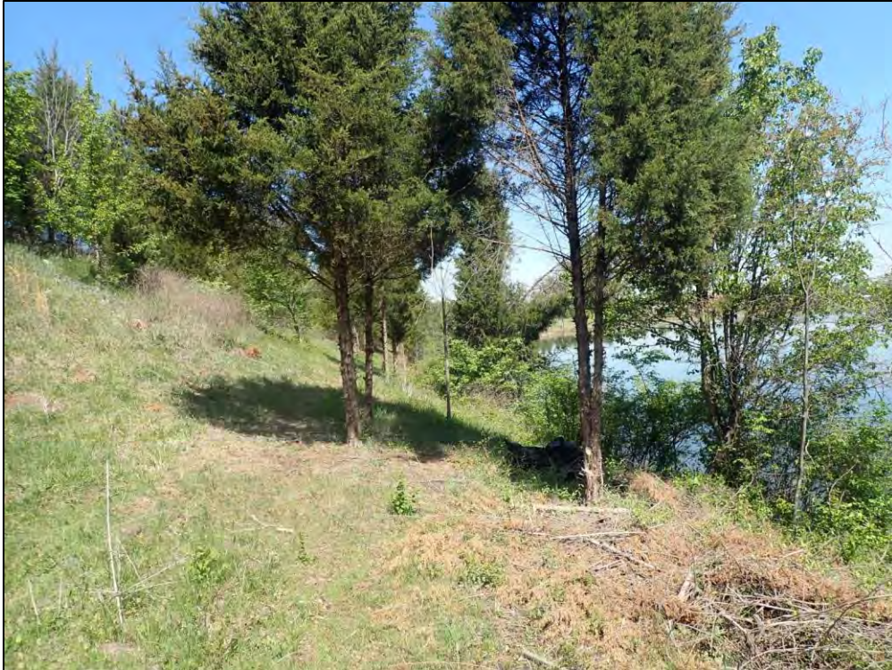
2767: Dam overall. Woody vegetation on the embankment (Routine Maintenance Needed).
