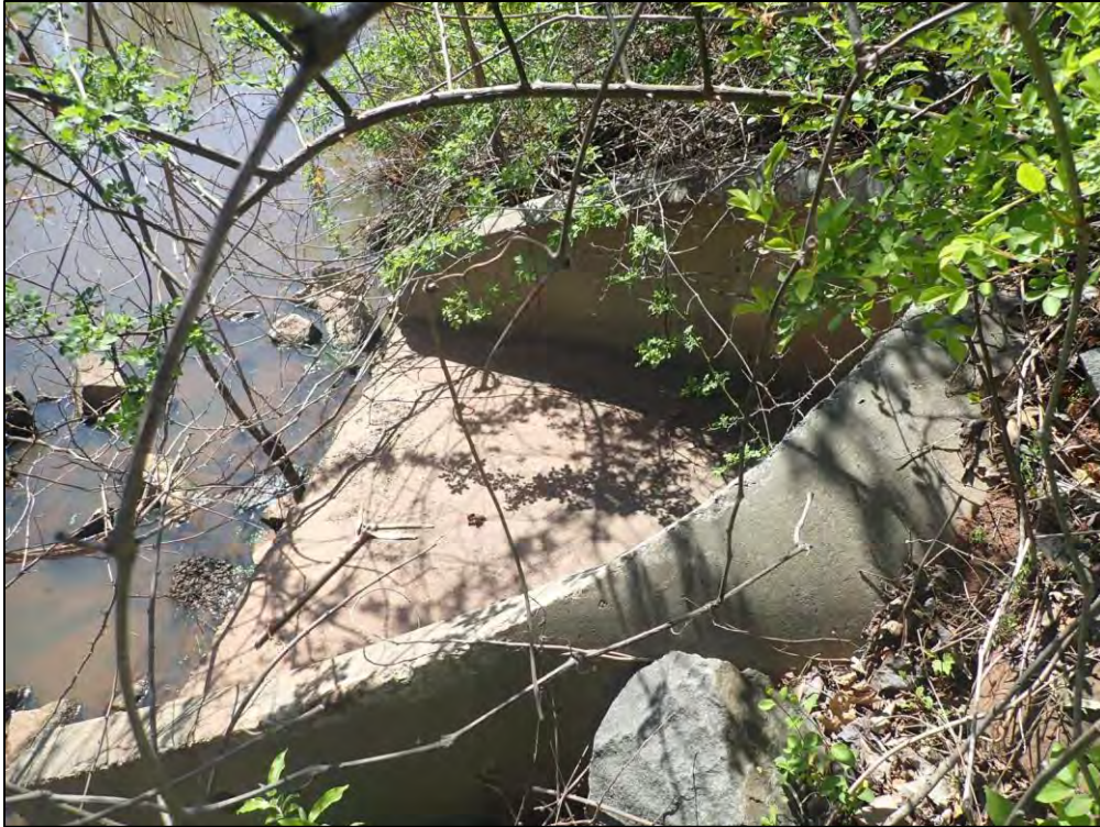
2828: Inflow Structure 2A, closeup. Woody growth around inflow structure (Routine Maintenance Needed).
