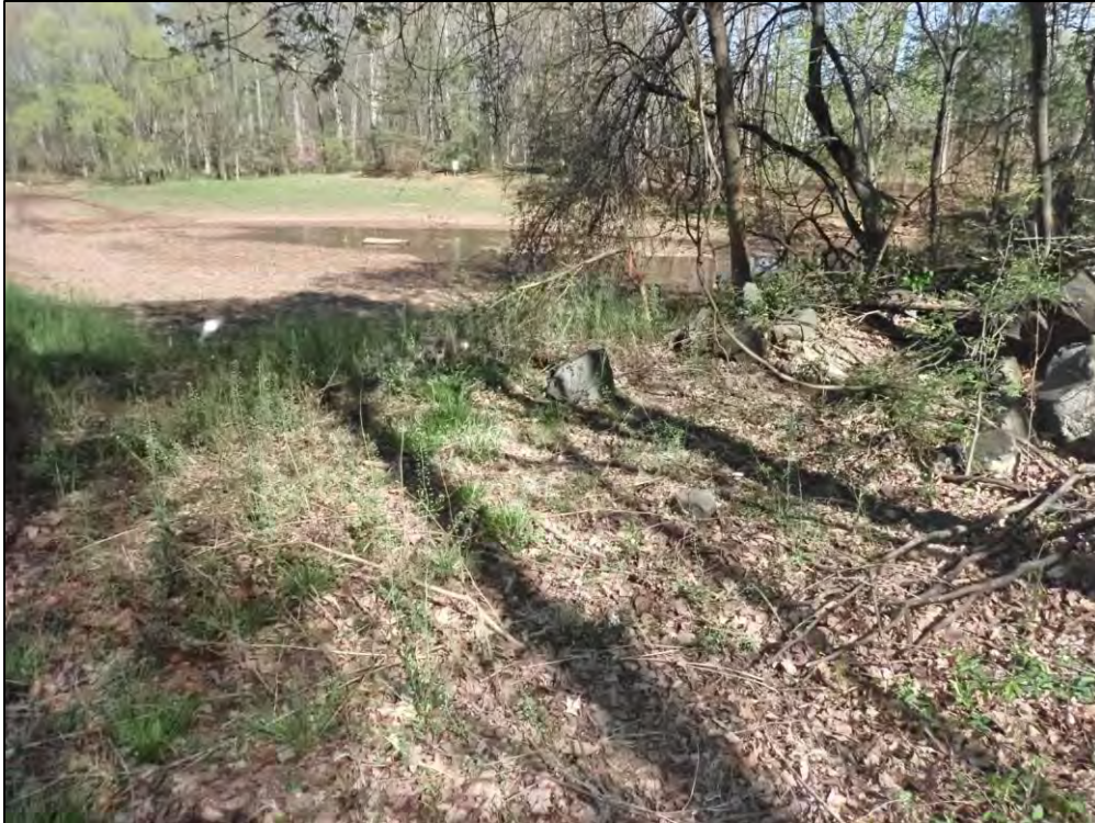
9357: Looking upstream from the Emergency Spillway. Woody vegetation on the embankment (Routine Maintenance Needed).
