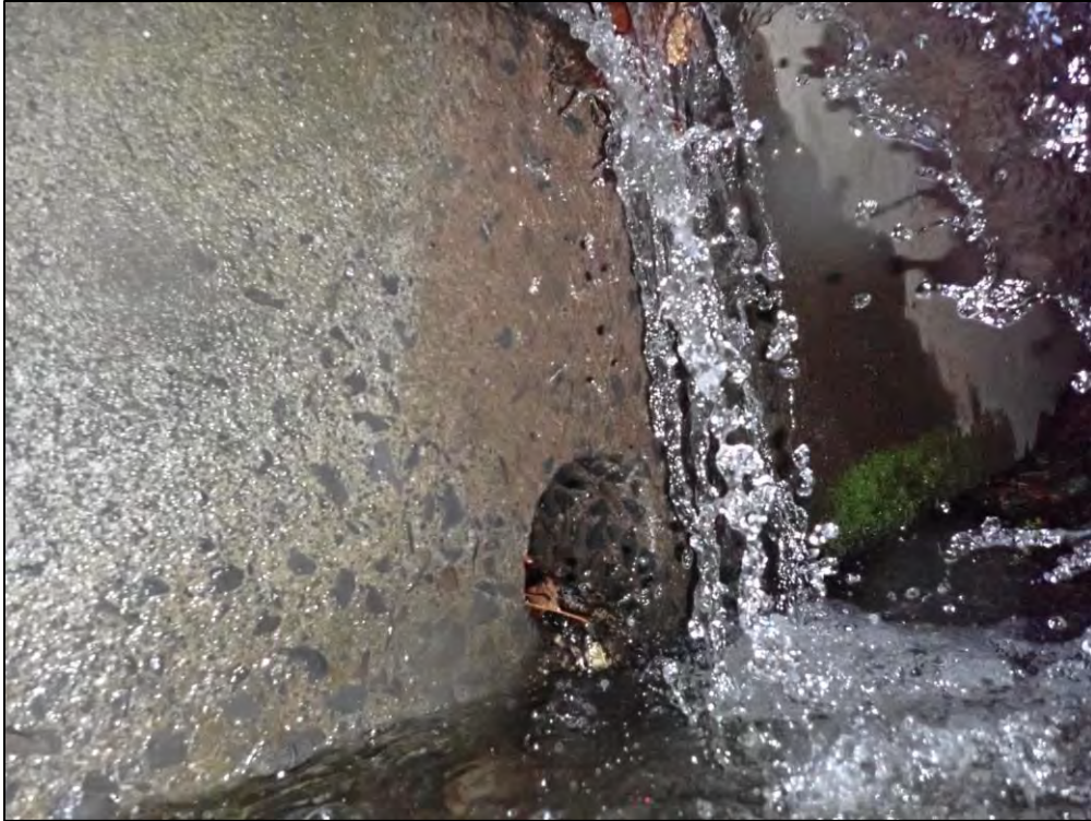
9297: Inside Control Structure D4, looking upstream toward the low-flow orifices. The low-flow orifices are blocked (Immediate Repair Needed).
