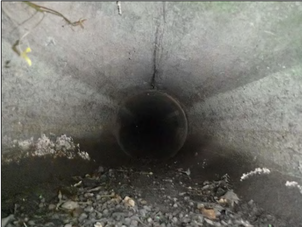
4752: Inside Inflow Structure A1. Buildup of trash, debris, and sediment (Routine Maintenance Needed).
