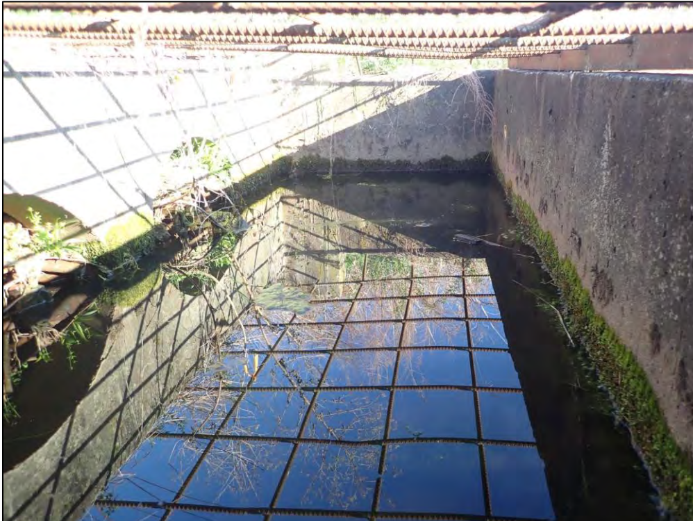
2695: Inside the Control Structure. Trash, debris, or other material in the BMP device (Routine Maintenance Needed).
