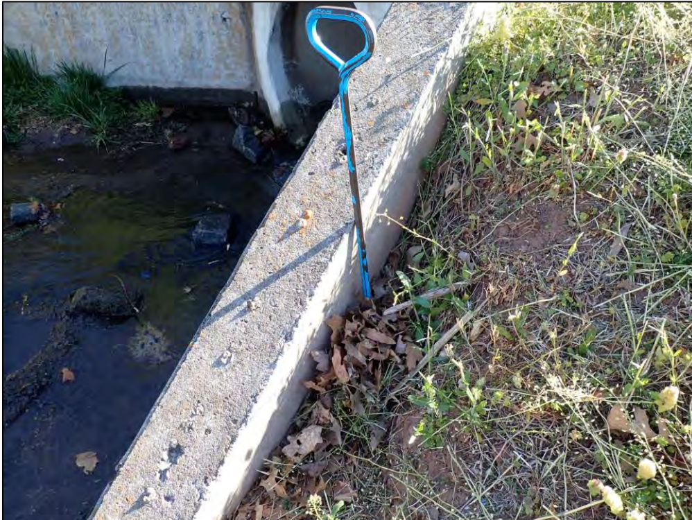
9324: Inflow Structure D5, closeup. Evidence of erosion or undermining around inlet (Routine Maintenance Needed).
