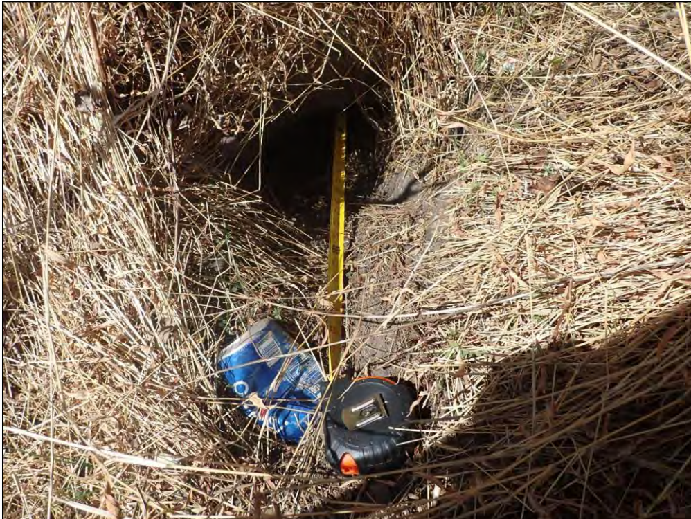
2806: Inflow 8, closeup. Evidence of nuisance animals (Routine Maintenance Needed).
