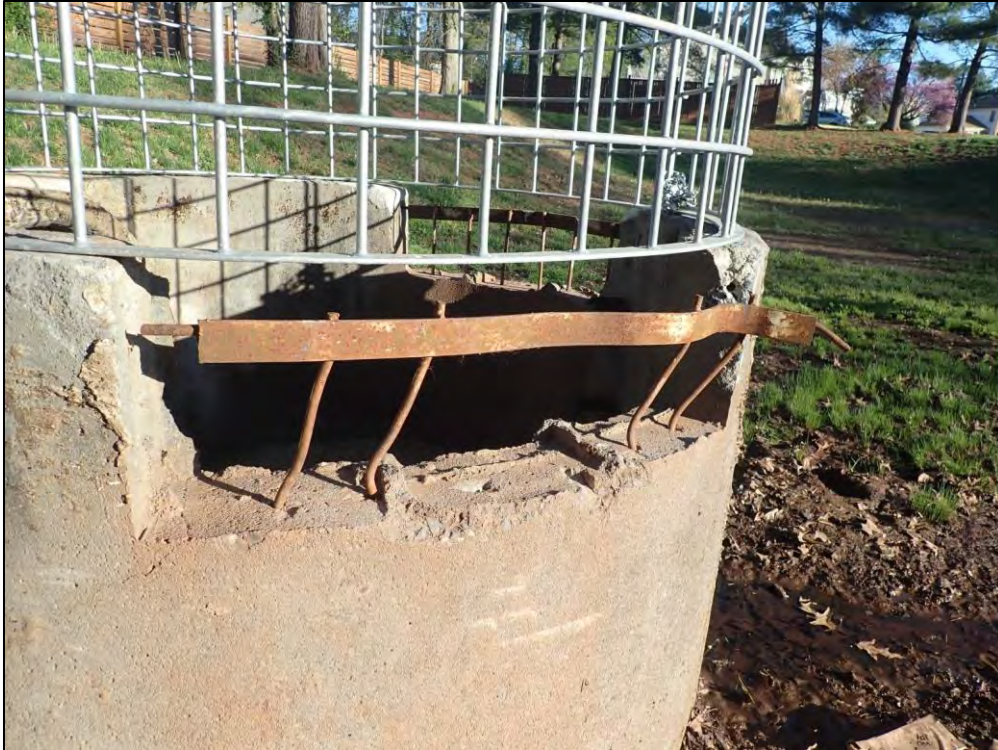
9265: Control Structure B2, Southern upper orifice close-up. Damage to trash rack. (Routine Maintenance Needed).
