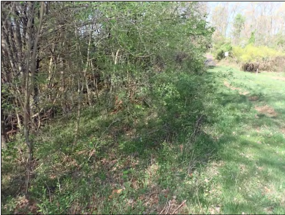
9351: Dam, Overall. Woody vegetation on the embankment (Routine Maintenance Needed).
