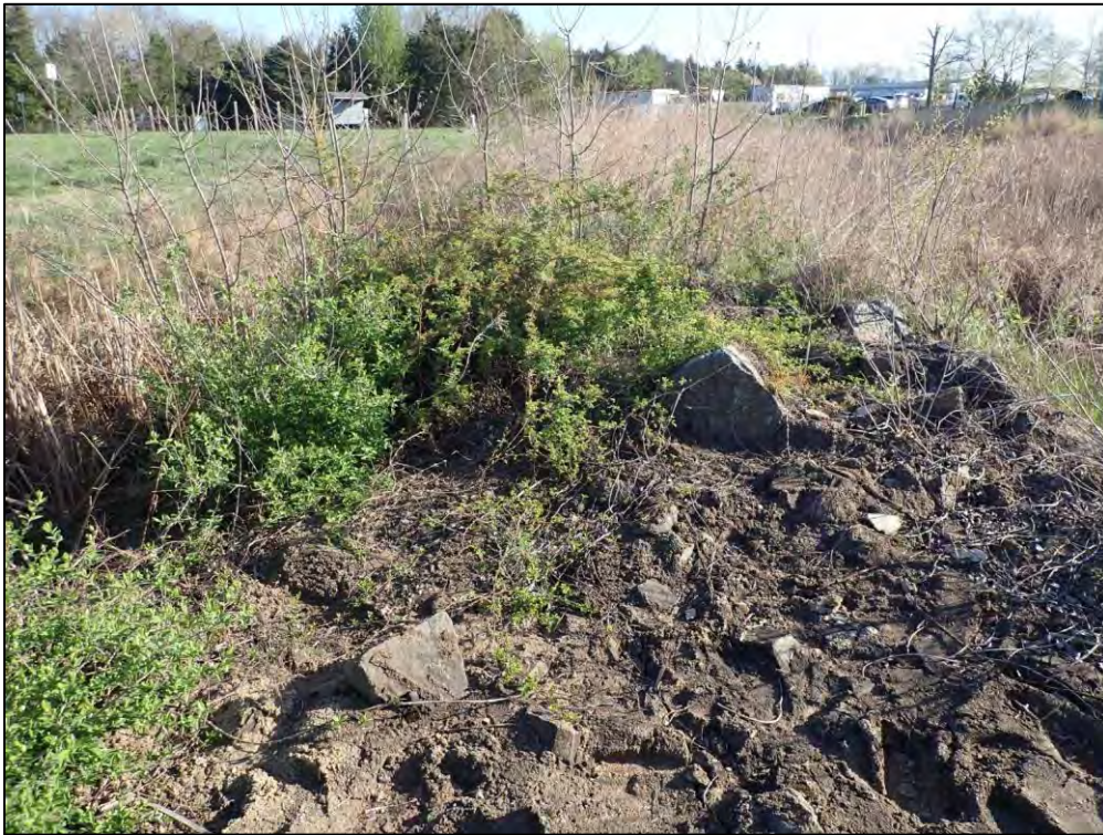
2704: Dam Overall. Woody vegetation on the embankment (Routine Maintenance Needed).
