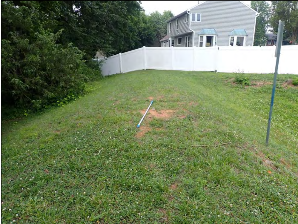
4732: Dam Overall. Sparse vegetative coverage (Monitor).
