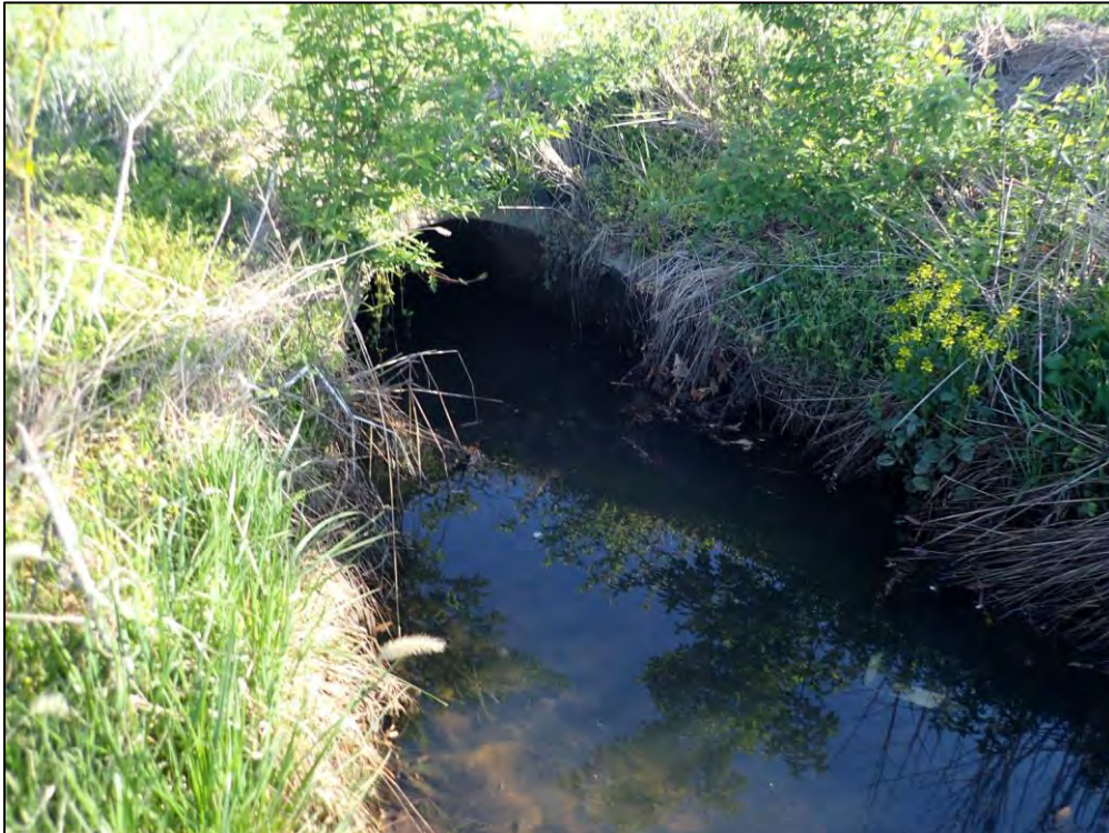
2717: Inflow Structure D9, front. Woody growth around inlet structure (Routine Maintenance Needed).
