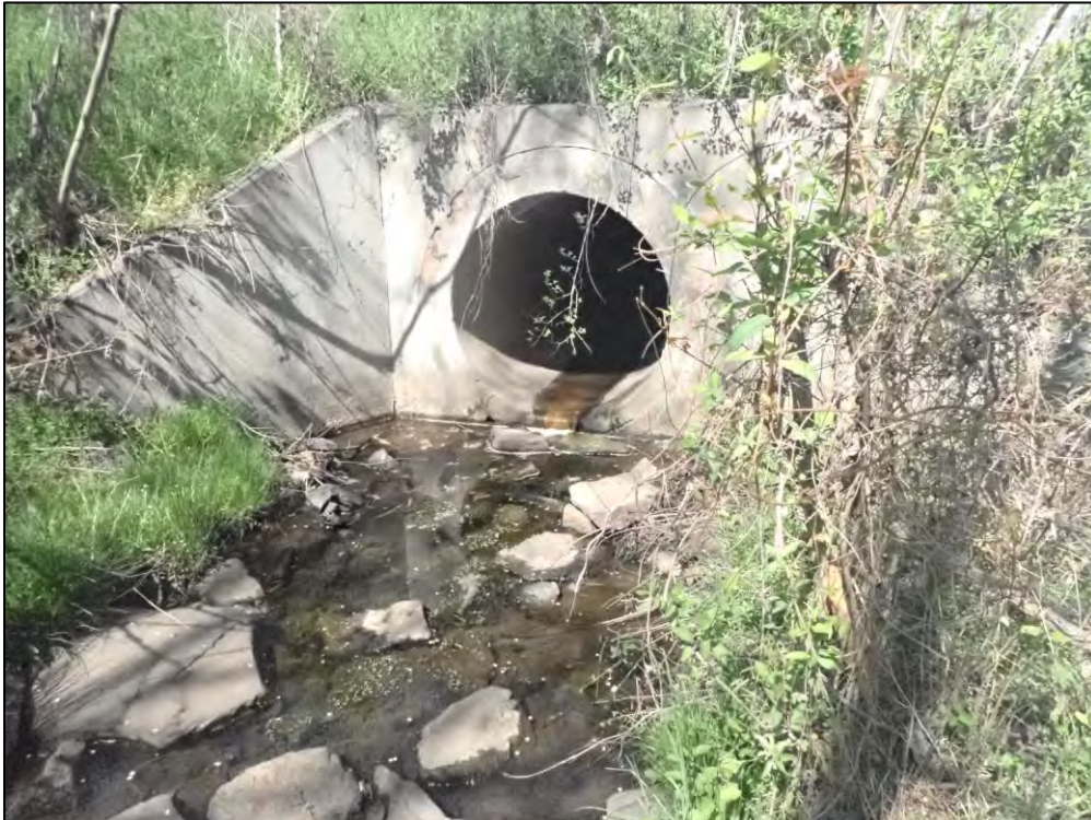
2843: Outfall Structure 4, front. Woody vegetation growing within 5' of outlet and barrel (Routine Maintenance Needed).
