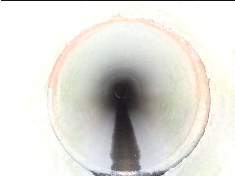
4797: Inside Inflow Structure 21. Joint misalignment and separation. (Routine Maintenance Needed).
