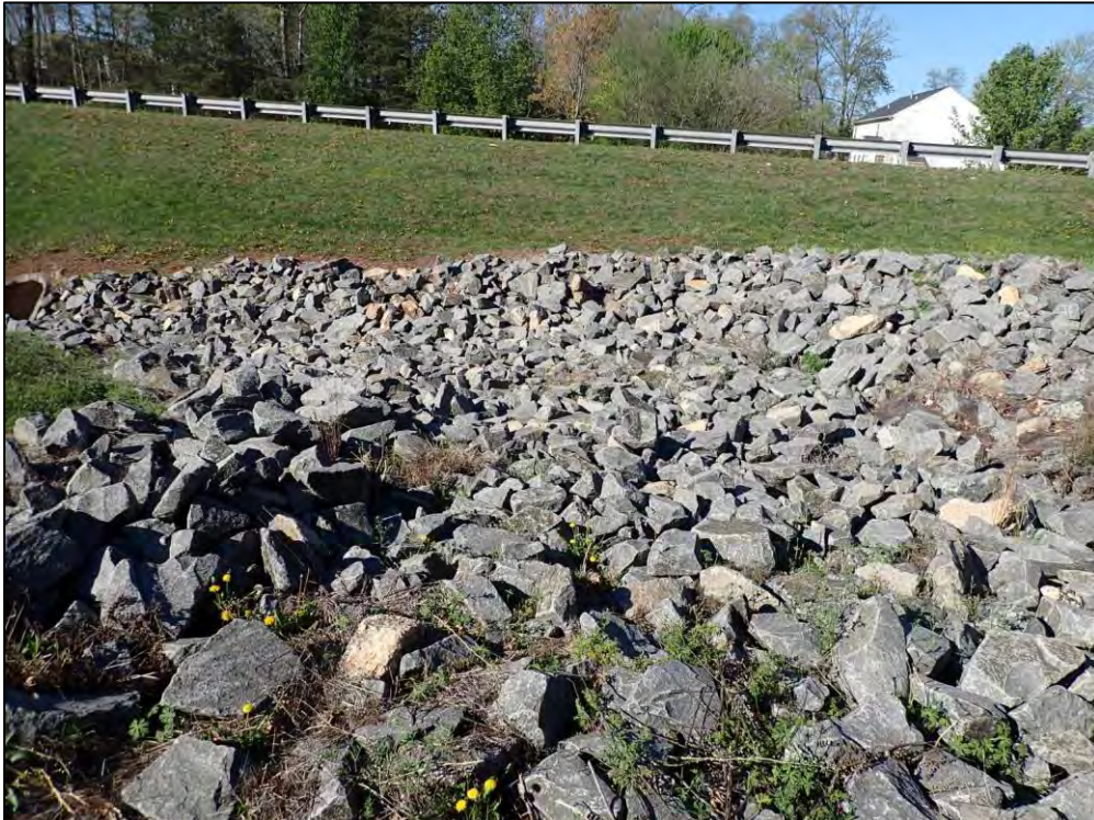
9312: Looking downstream along the Emergency Spillway. Shrubbery, low-growing vegetation, and/or vine material growing on the embankment (Monitor).
