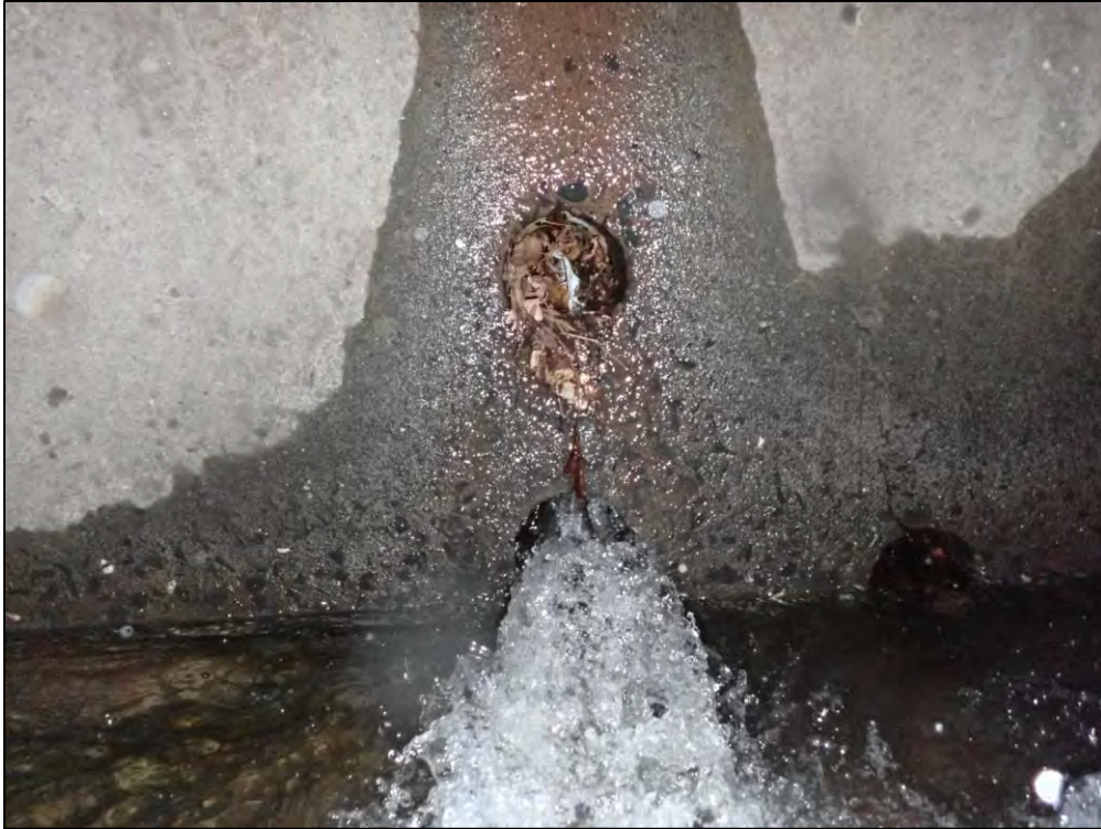
9295: Inside Control Structure D4, looking upstream toward the low-flow orifices. The low-flow orifices are blocked (Immediate Repair Needed).
