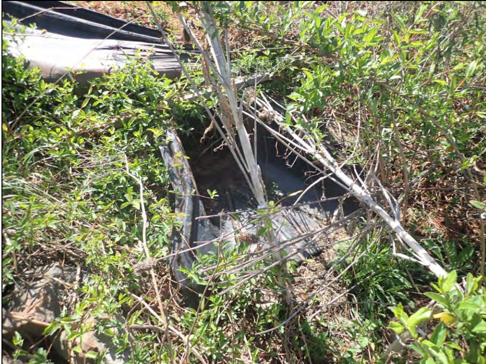
2769: Inflow 1, front. Buildup of trash, debris, and sediment (Routine Maintenance Needed).
