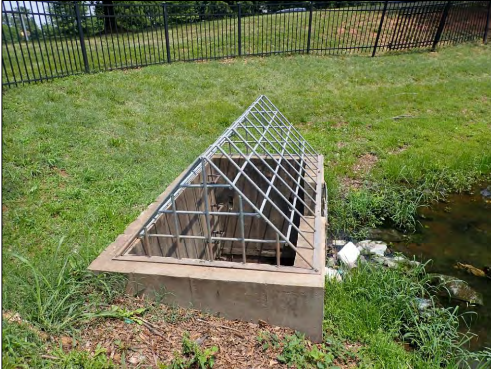
4776: Control Structure 37, top trash rack. Trash, debris, or other material in BMP device (Routine Maintenance Needed).
