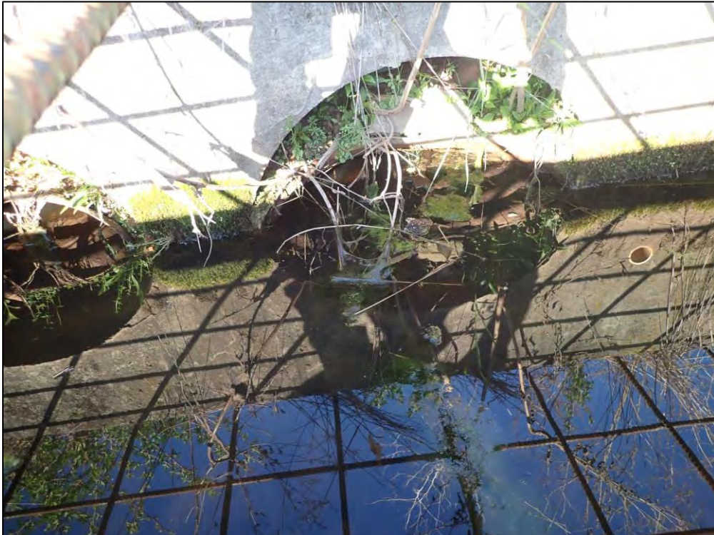
2697: Inside the Control Structure, looking downstream toward the Northern pipe. Trash, debris, or other material in the BMP device (Routine Maintenance Needed).
