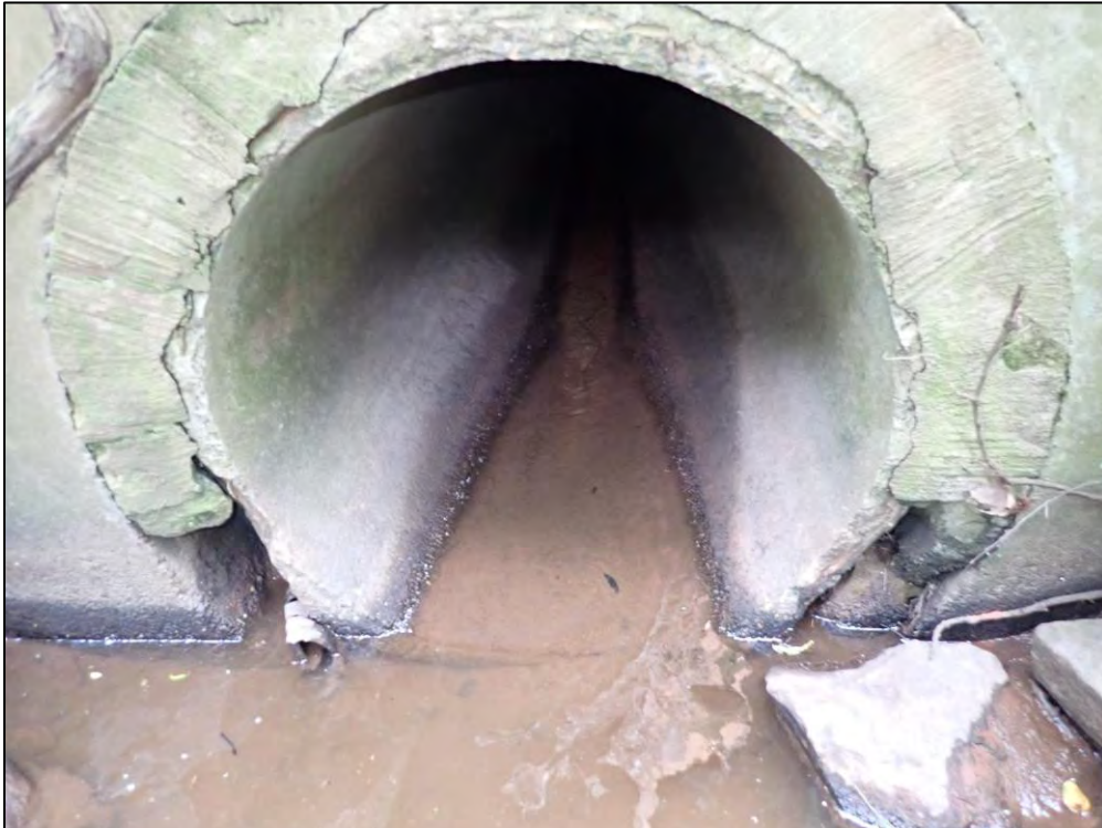
4783: Outfall Structure 36, close-up. The outfall structure is damaged, Spalling(Routine Maintenance Needed).
