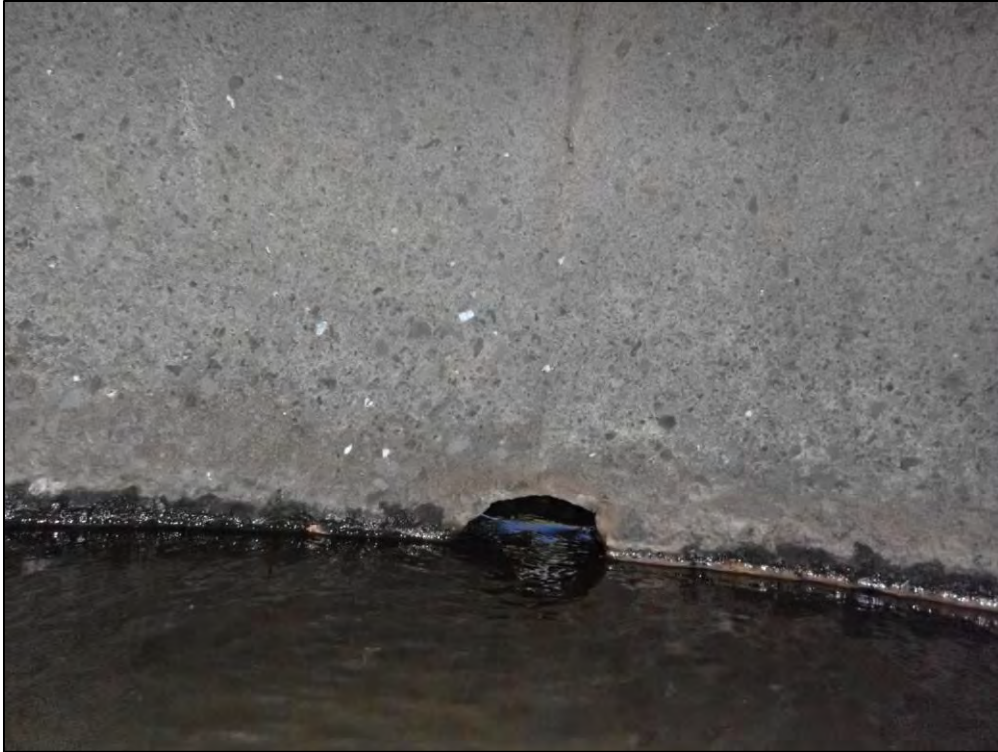
9341: Inside the Control Structure, looking upstream toward the Eastern low-flow orifice. The low-flow orifices are blocked (Immediate Repair Needed).
