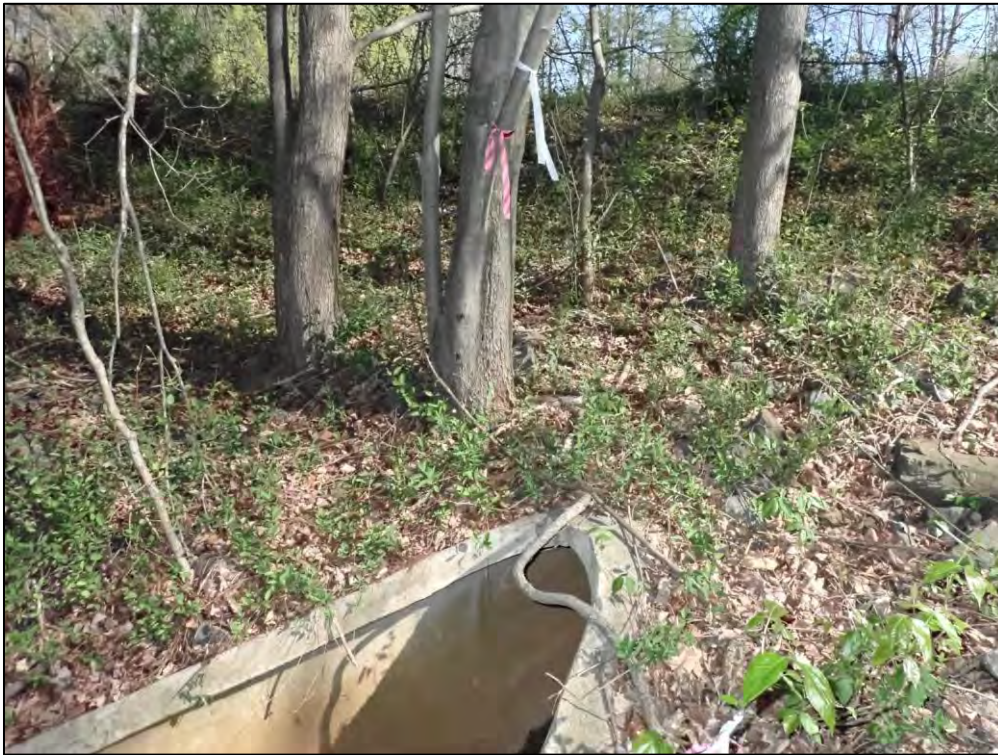
9349: Outfall, Overall. Woody vegetation growing within 5' of outlet and barrel (Routine Maintenance Needed).
