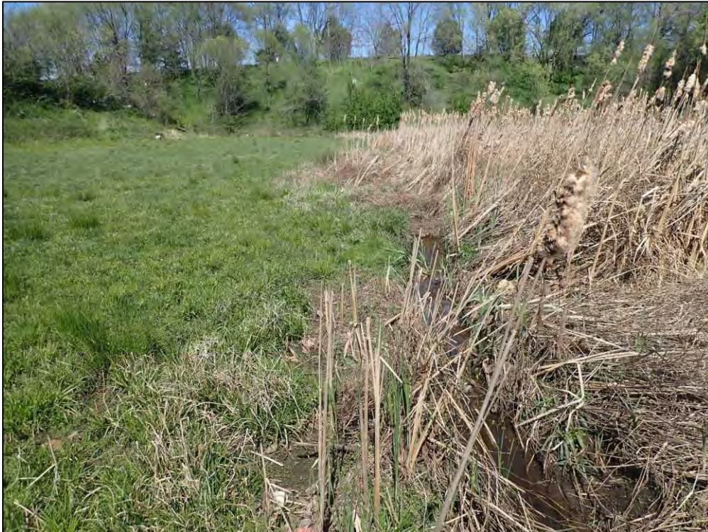
2849: Looking upstream along the Trickle Ditch toward Inflow Structure 2. Sediment observed within the trickle ditch. (Routine Maintenance Needed).
