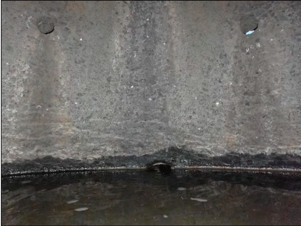
9343: Inside the Control Structure, looking upstream toward the Northeastern low-flow orifice. The low-flow orifices are blocked (Immediate Repair Needed).
