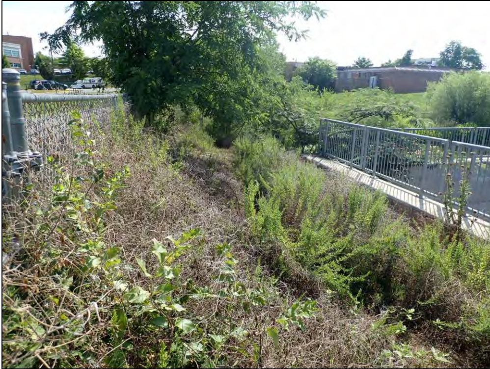
4430: Dam Overall, front slope. Shrubbery, low-growing vegetation, and/or vine material growing on the embankment (Routine Maintenance Needed).
