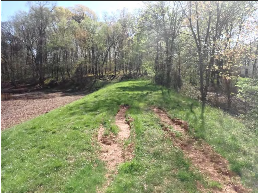
9352: Dam, Overall. Sparse vegetative coverage (Monitor).
