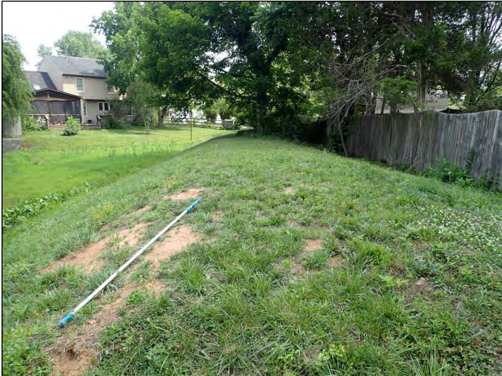
4733: Dam Overall. Sparse vegetative coverage (Monitor).
