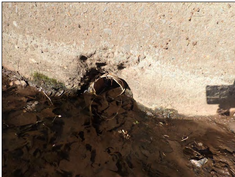
9263: Control Structure B2, low-flow orifice close-up.
