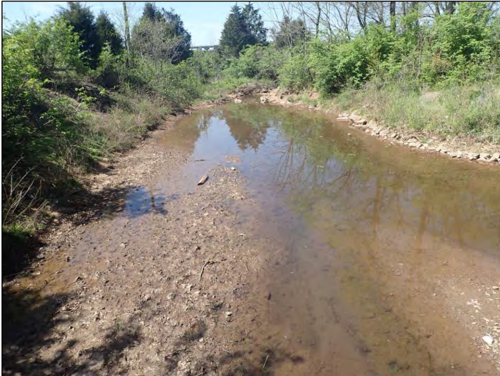
2784: From Inflow 4, looking downstream. Buildup of trash, debris, and sediment (Routine Maintenance Needed).
