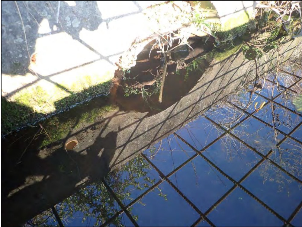
2696: Inside the Control Structure, looking downstream toward the Southern pipe. Trash, debris, or other material in the BMP device (Routine Maintenance Needed).
