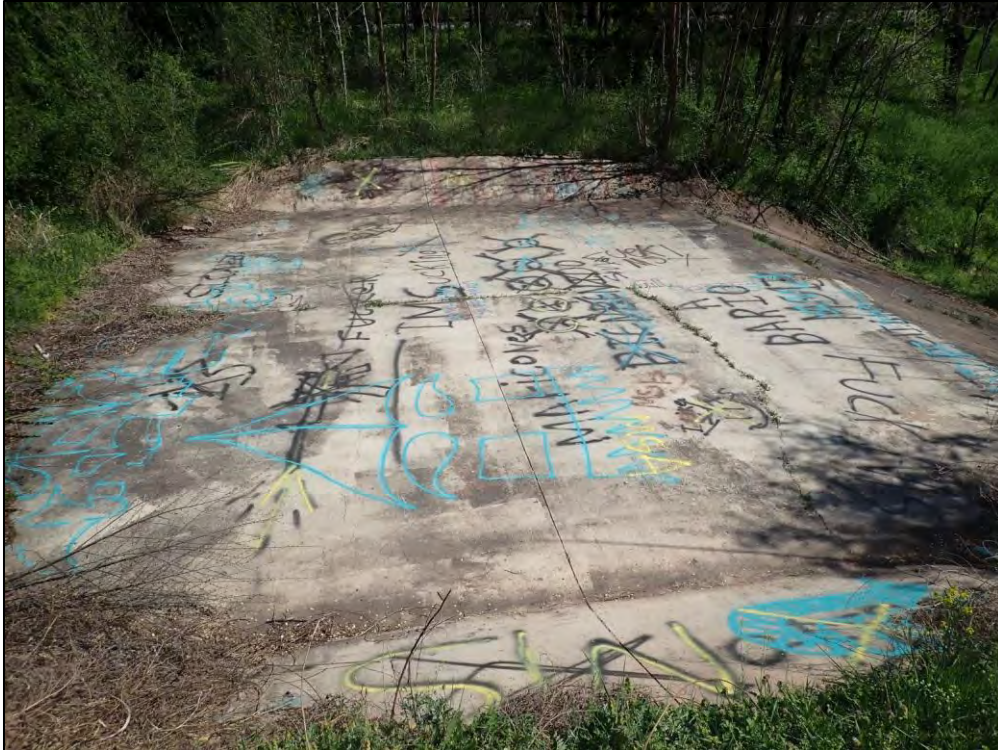
2848: Emergency Spillway, overall. Woody vegetation on the embankment (Routine Maintenance Needed).
