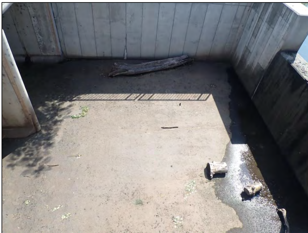
4434: Inside Control Structure 11. Trash, debris, or other material in BMP device (Monitor).
