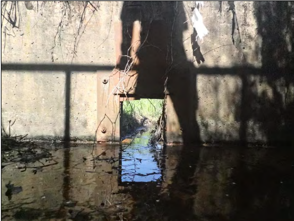
2841: Inside Control Structure 3, looking upstream toward the low-flow orifice. Orifice Plate is missing (Immediate Repair Needed).
