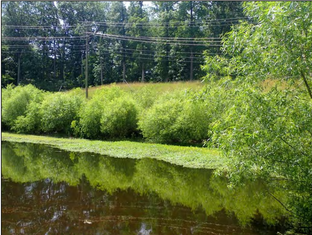
4480: Inflow Structure 6, Overall. Woody growth around inlet structure (Immediate Repair Needed).
