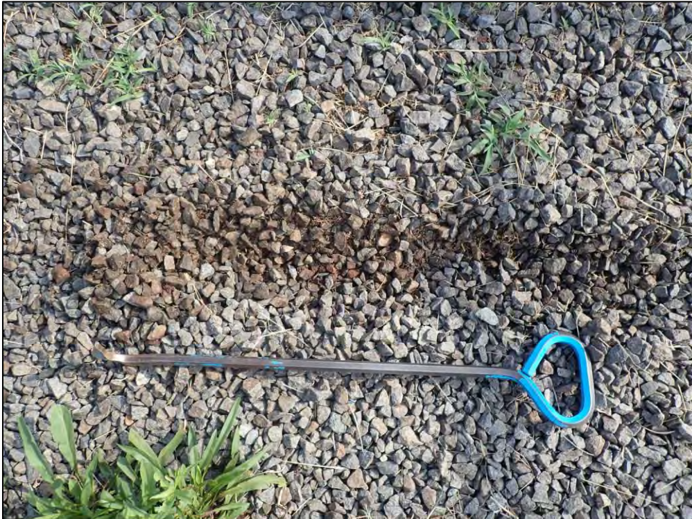
4587: Another close-up showing the Gravel Detail. Evidence of clogging (Immediate Repair Needed).
