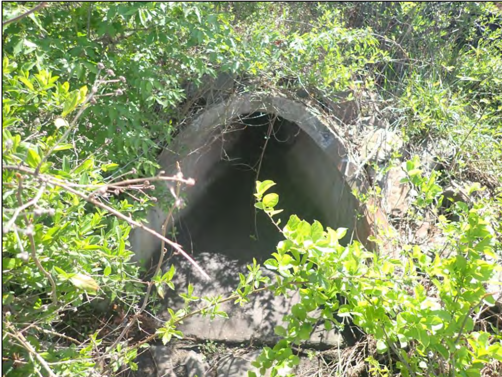
2772: Inflow 2, front. Buildup of trash, debris, and sediment (Routine Maintenance Needed).
