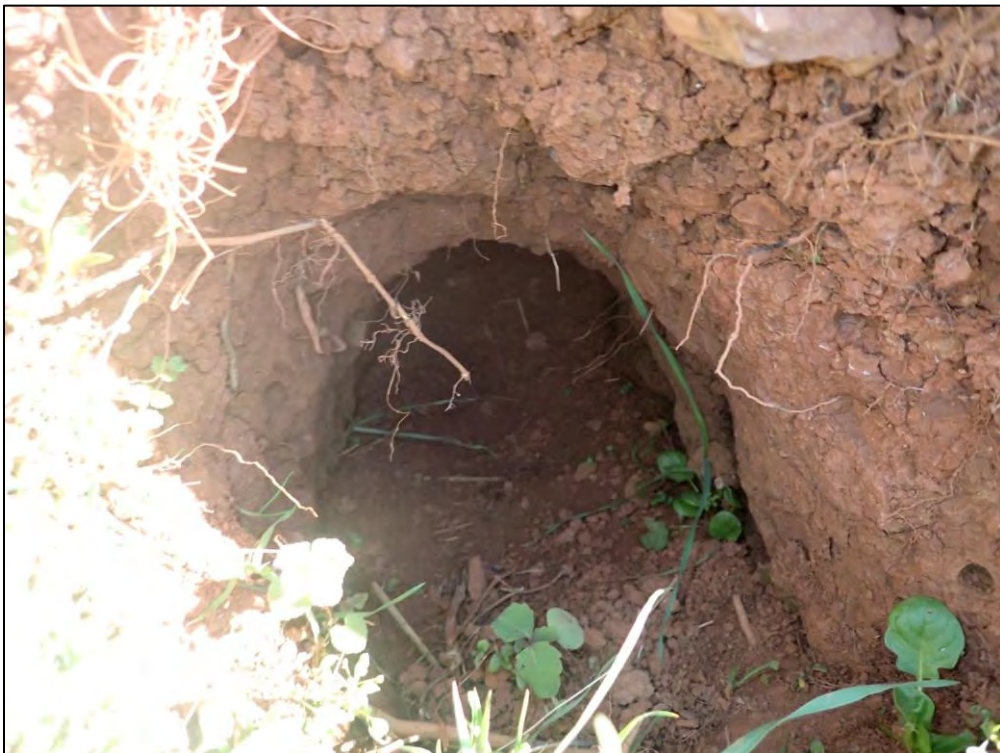
2748: Animal Hole 2, closeup. Evidence of nuisance animals (Routine Maintenance Needed).
