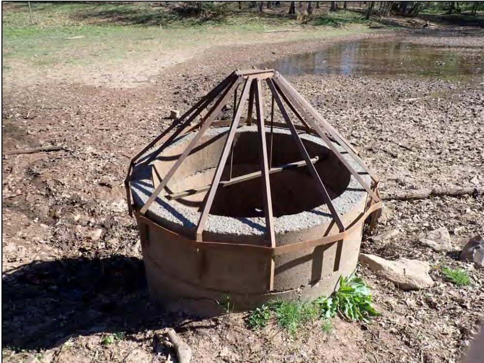
9338: Control Structure, top trash rack.
