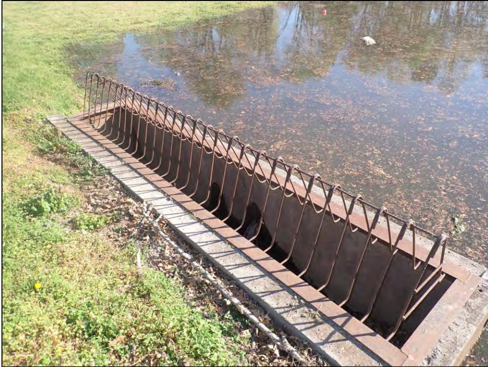
9293: Control Structure D4, top trash rack.
