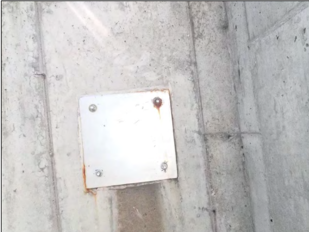
4442: Inside Control Structure 11, looking upstream toward the Dewatering Orifice. The BMP Orifice Plate device is missing (Immediate Repair Needed).
