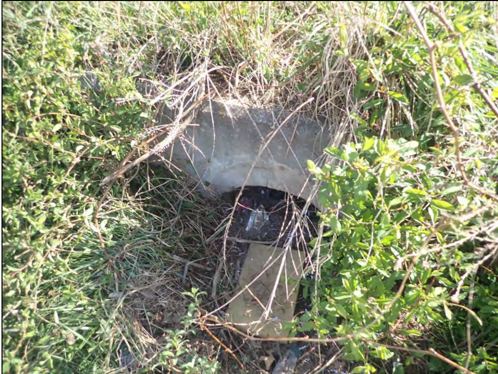
2754: Inflow 4, front. Buildup of trash, debris, and sediment (Routine Maintenance Needed). Woody growth around inlet structure, Non-woody overgrown veg. (Routine Maintenance Needed).
