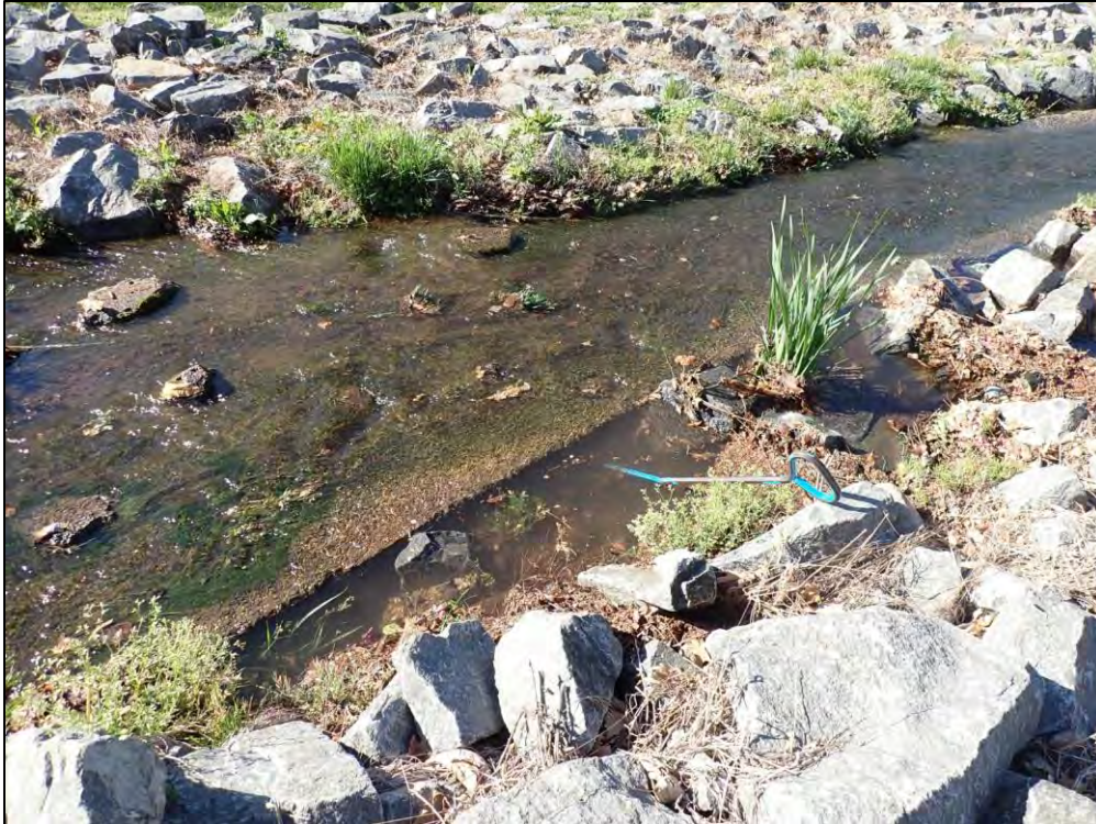
9330: Trickle Ditch, overall. Sections of the low-flow ditch are cracked or showing signs of undercutting (Routine Maintenance Needed).
