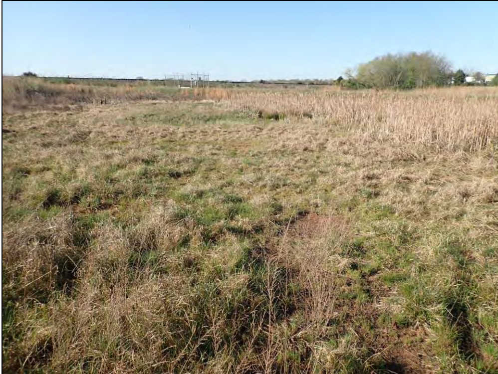
2708: Facility Overall. Overgrown vegetation was observed on the pond floor (Routine Maintenance Needed).
