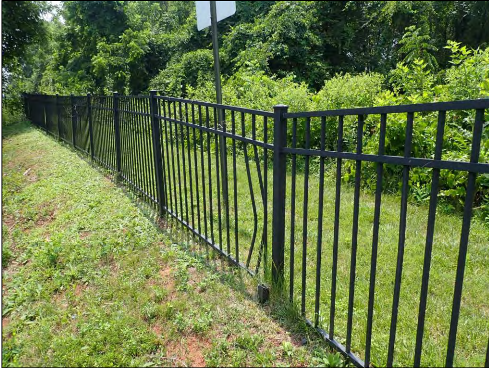
4790: Fence, Overall. Fence is damaged (Routine Maintenance Needed).
