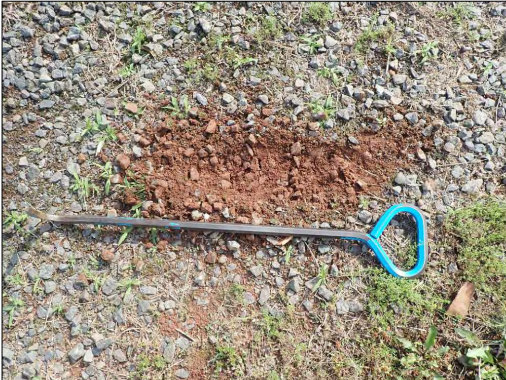
4583: Close-up showing the Gravel Detail. Evidence of clogging (Immediate Repair Needed).
