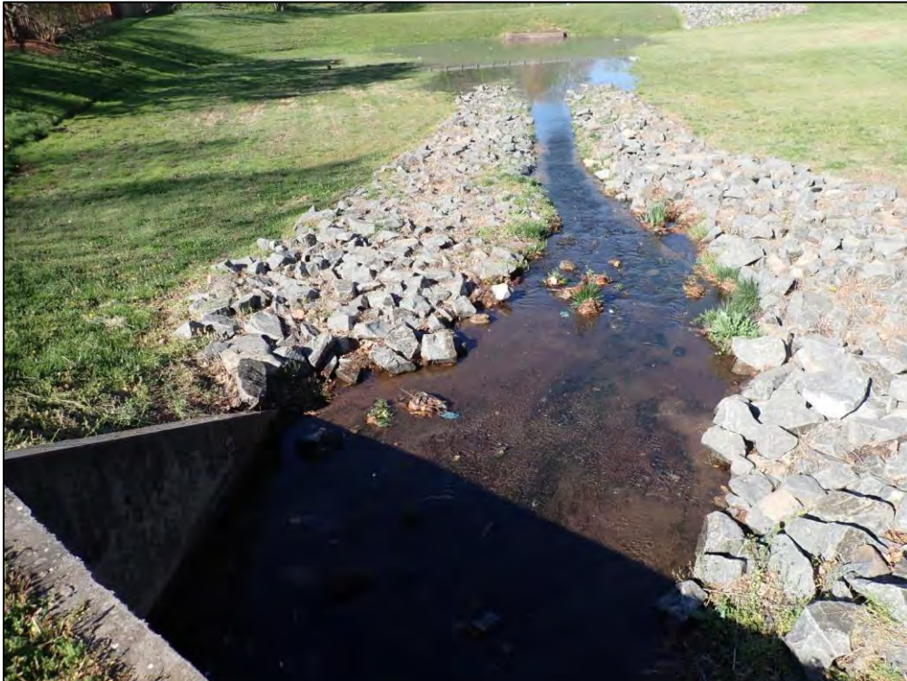
9322: From Inflow Structure D5, looking downstream. Buildup of trash, debris, and sediment (Monitor).
