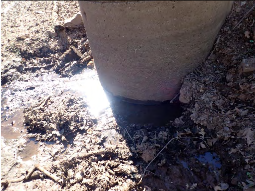
9337: Control Structure, low-flow orifice close-up. The low-flow orifices are blocked (Immediate Repair Needed).
