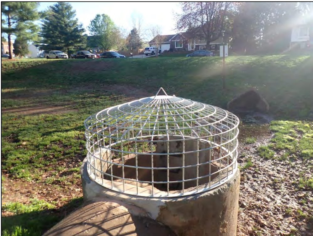
9266: Control Structure B2, top trash rack.
