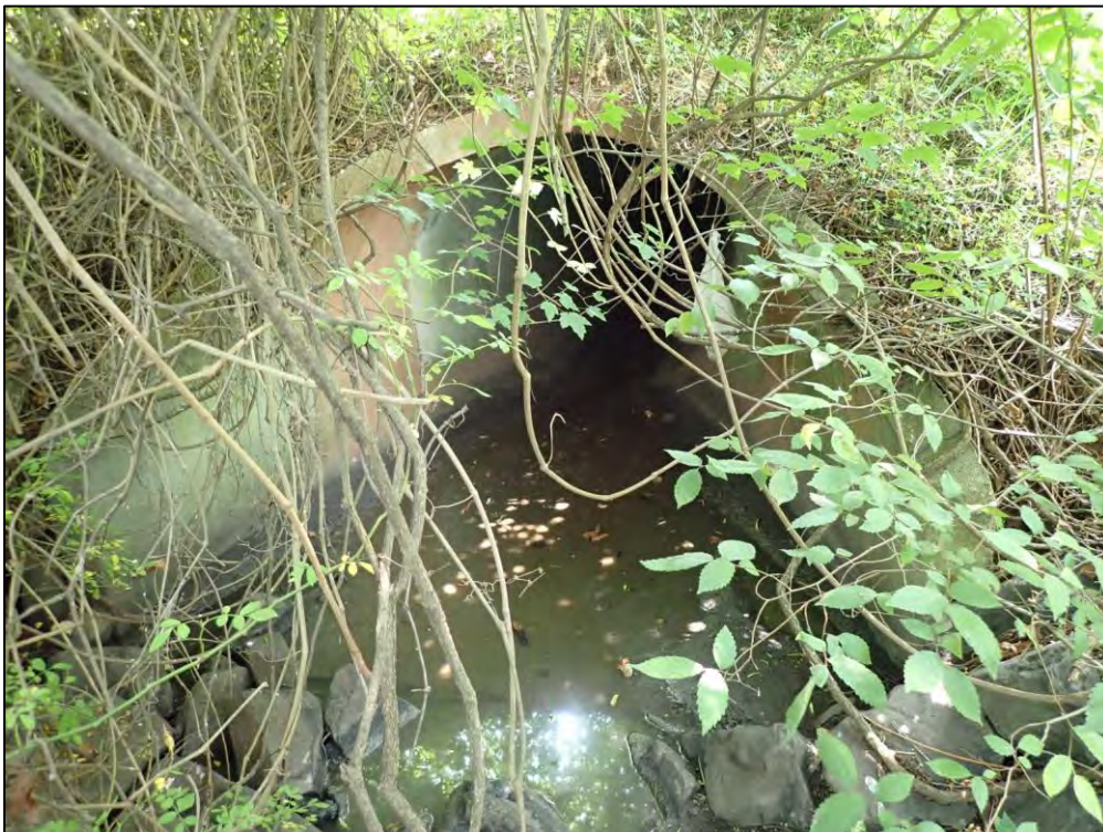
4791: Inflow Structure 1, front. Overgrown Vegetation is present (Routine Maintenance Needed).
