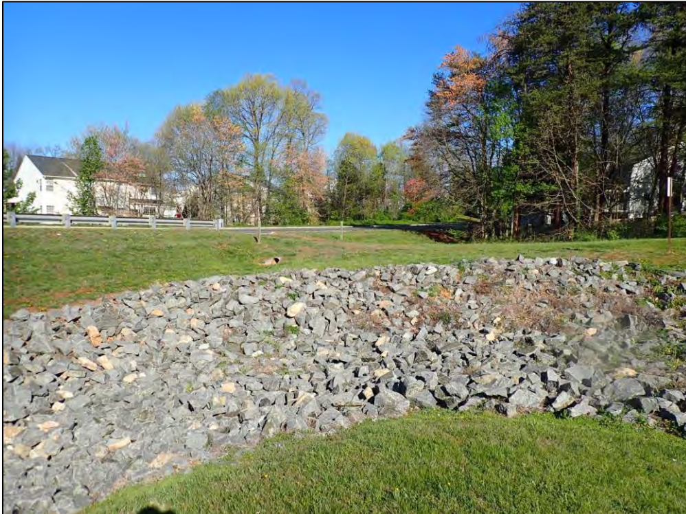
9310: Emergency Spillway, Overall. Shrubby, low-growing vegetation, and/or vine material growing on the embankment (Monitor).
