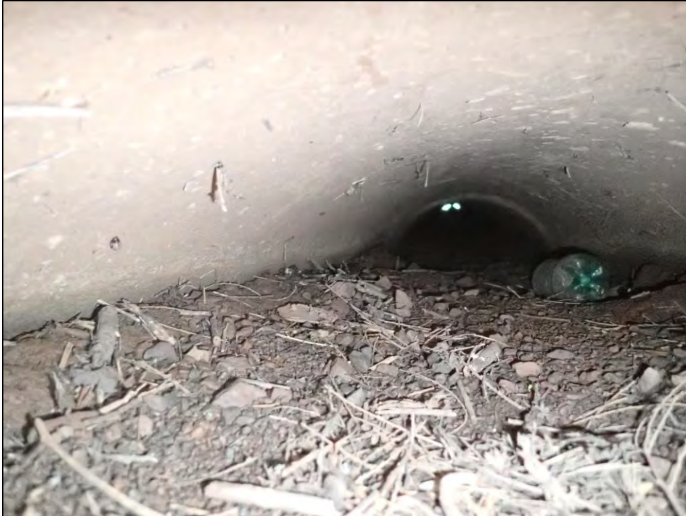
4465: Inside Inflow Structure 3A. Buildup of trash, debris, and sediment (Immediate Repair Needed).
