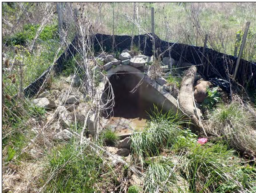
2775: Inflow 3, front. Buildup of trash, debris, and sediment (Routine Maintenance Needed).
