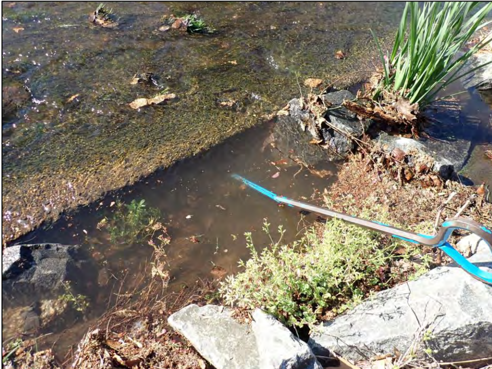
9331: Trickle Ditch, close-up. Sections of the low-flow ditch are cracked or showing signs of undercutting (Routine Maintenance Needed).
