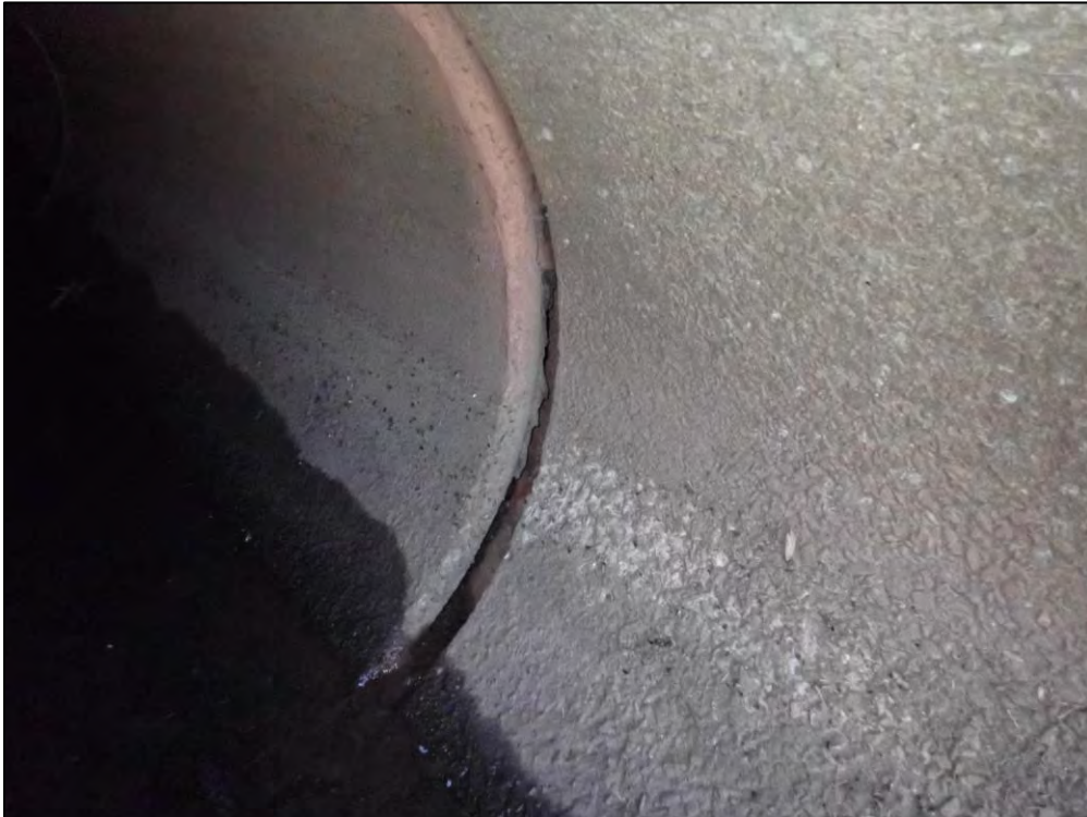
9285: Inflow Structure A1, closeup. Joint Separation (Routine Maintenance Needed).
