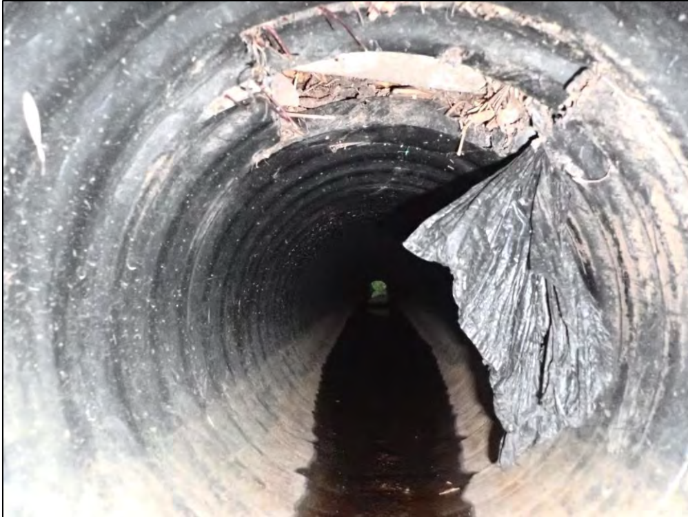
4726: Inside the Control Structure. Evidence of damaged joint (Routine Maintenance Needed).
