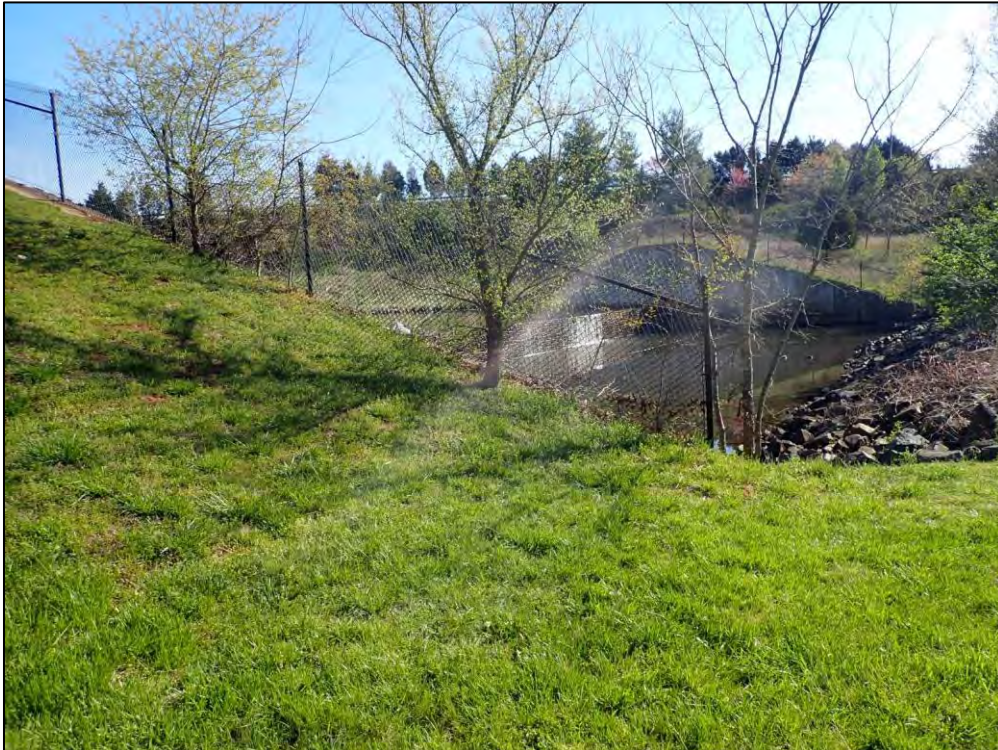
2734: Dam Overall, back slope. Woody vegetation on the embankment (Routine Maintenance Needed).
