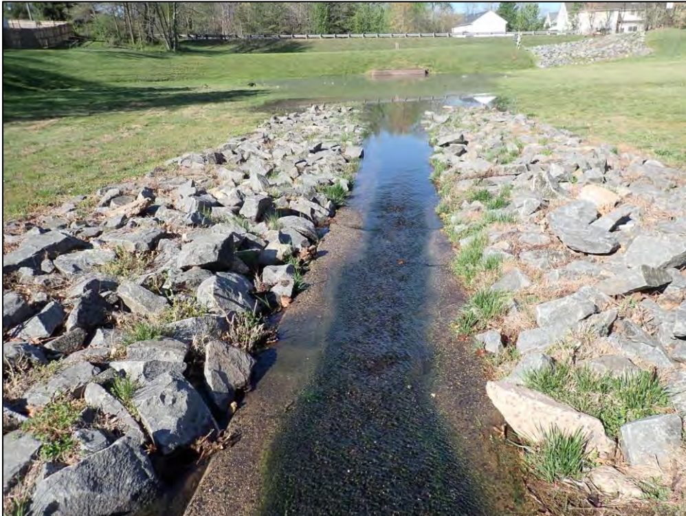
9327: Looking downstream along the Trickle Ditch. The low-flow ditch is clogged with sediment/debris (Monitor).
