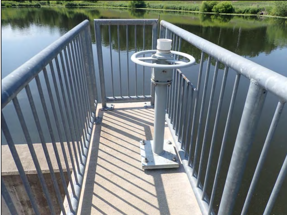
4438: Control Structure 11, Dewatering valve close-up.
