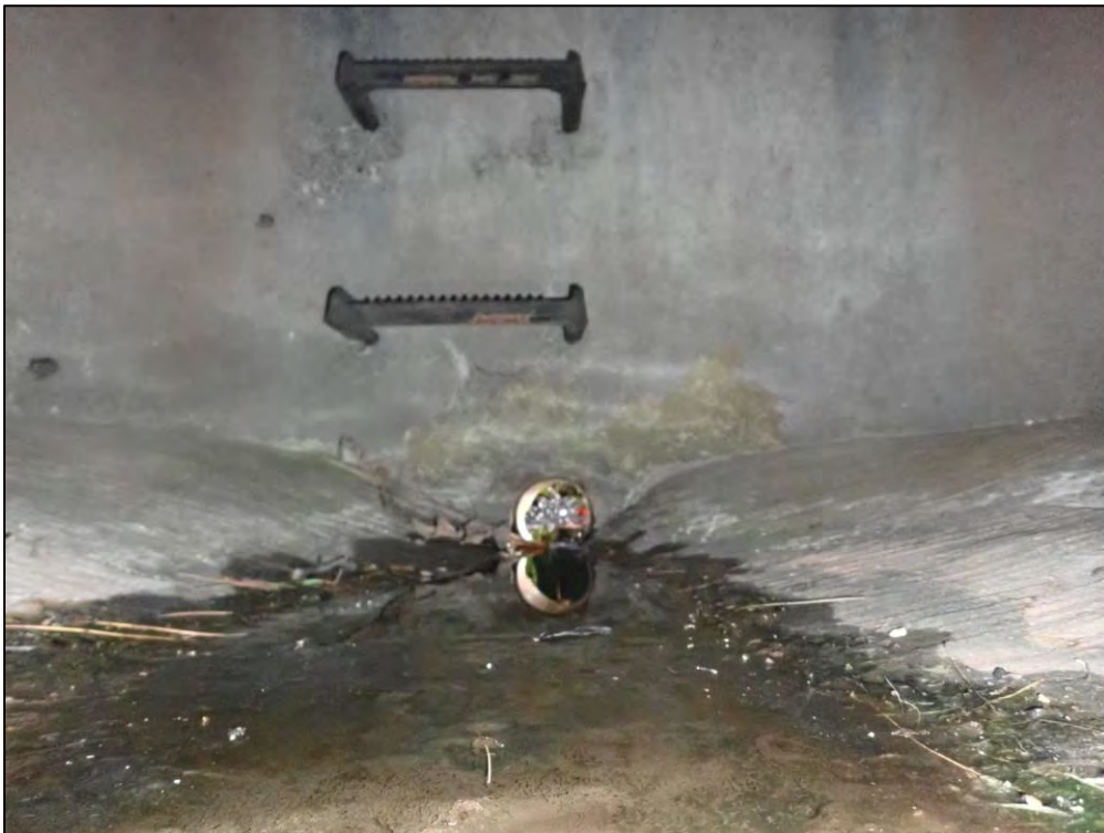
9268: Inside Control Structure B2, looking upstream toward the low-flow orifice.
