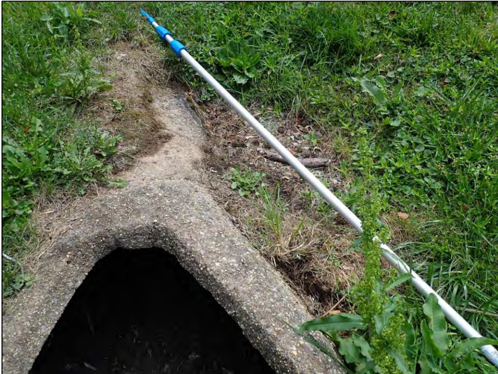
4739: Inflow Structure D1, closeup. Evidence of erosion or undermining around inlet (Routine Maintenance Needed).
