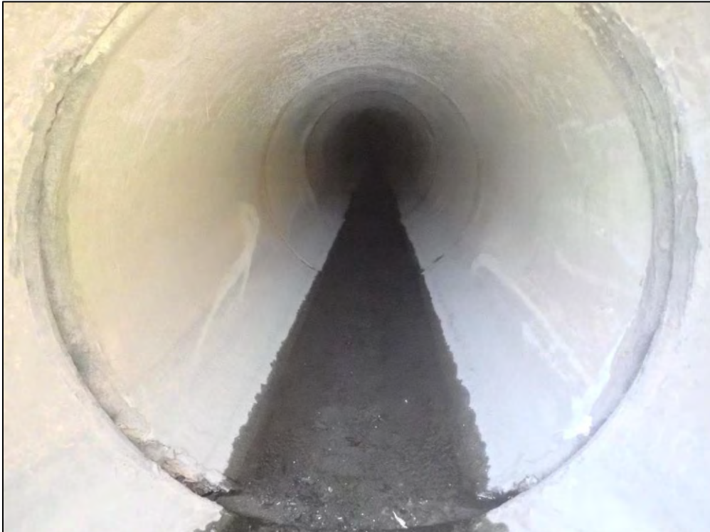
2857: Inside Inflow Structure 2. Joint separation observed (Routine Maintenance Needed).
