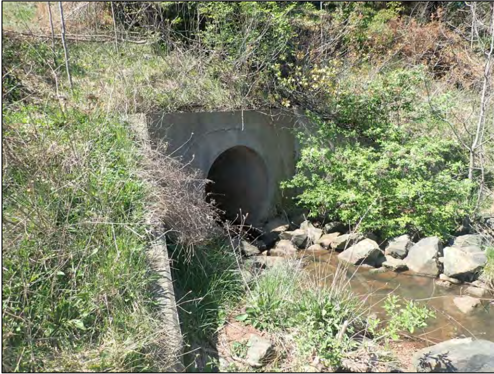
2815: Inflow 10, front. Woody growth around inlet structure (Routine Maintenance Needed).
