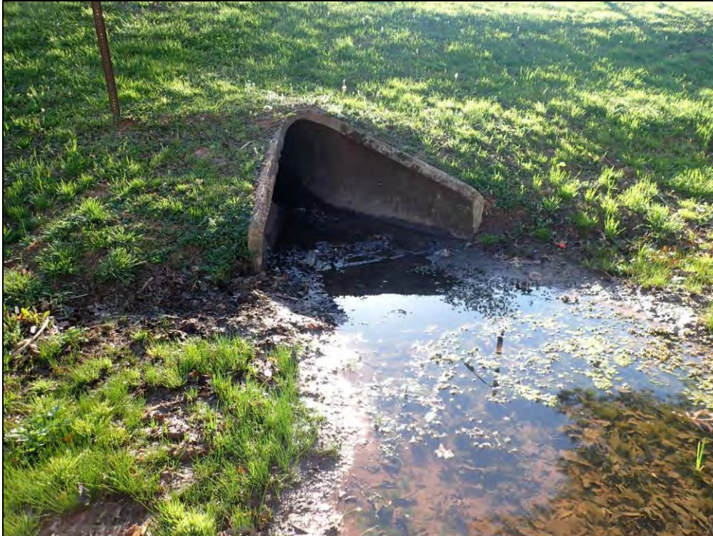
9282: Inflow Structure A1, front. Buildup of trash, debris, and sediment (Routine Maintenance Needed).
