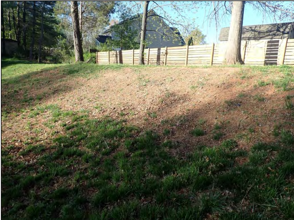
9280: Bare Spot, Overall. Sparse vegetative coverage (Routine Maintenance Needed).
