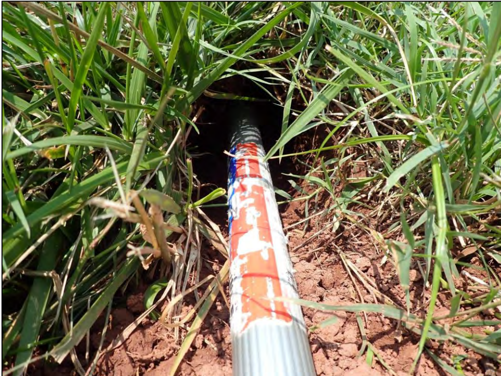
4789: Animal hole, closeup. Evidence of nuisance animals (Immediate Repair Needed).
