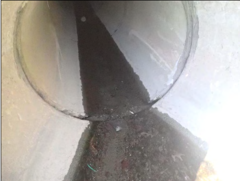
2856: Inflow Structure 2, closeup. Joint separation observed (Routine Maintenance Needed).
