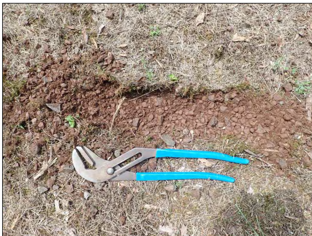
4801: Close-up showing the Gravel Detail. Evidence of clogging (Immediate Repair Needed).
