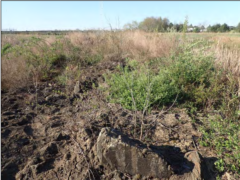
2705: Emergency Spillway, Overall. Woody vegetation on the embankment (Routine Maintenance Needed).
