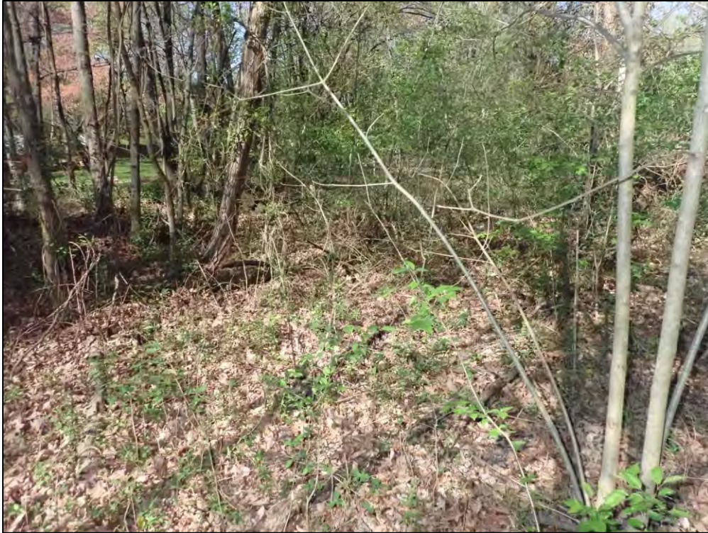
9359: Emergency Spillway, Overall. Woody vegetation on the embankment (Routine Maintenance Needed).
