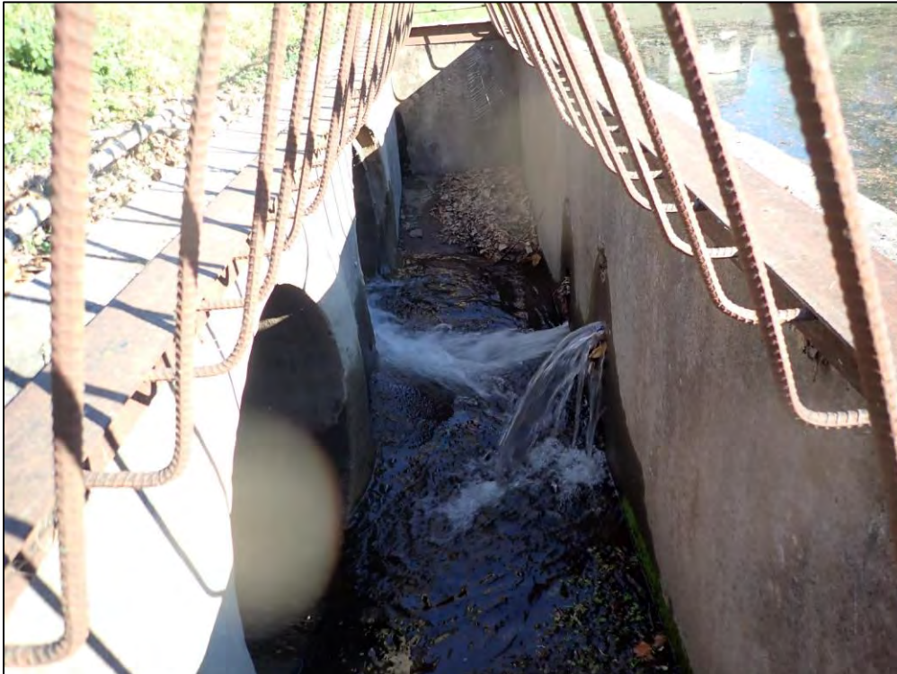
9300: Inside Control Structure D4. The low-flow orifices are blocked (Immediate Repair Needed).
