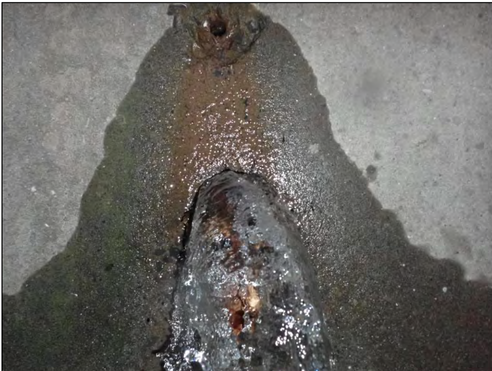
9296: Inside Control Structure D4, looking upstream toward the low-flow orifices. The low-flow orifices are blocked (Immediate Repair Needed).
