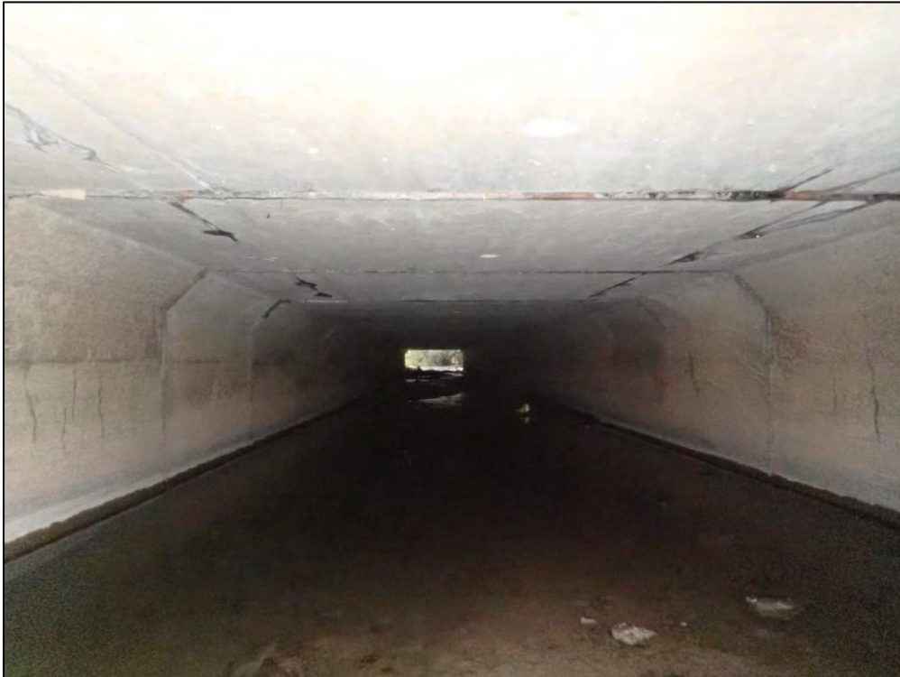
2782: Inside Inflow 4, looking along the Middle pipe. Buildup of trash, debris, and sediment (Routine Maintenance Needed).
