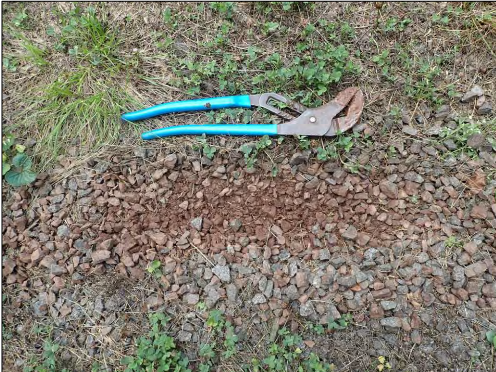
4805: Another close-up showing the Gravel detail. Evidence of clogging (Immediate Repair Needed).
