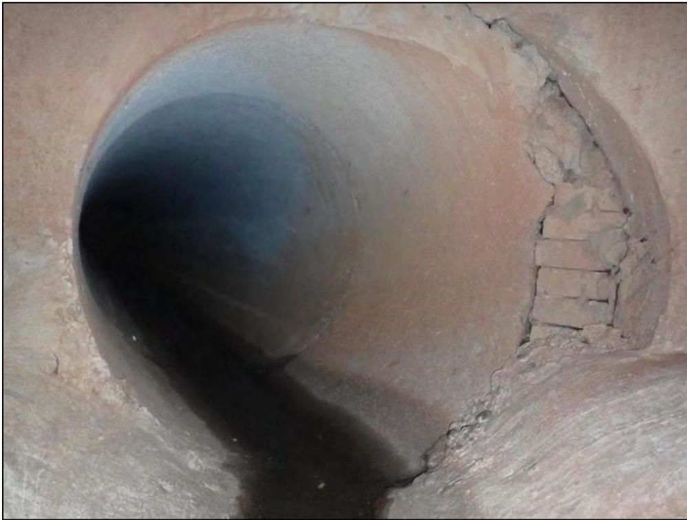
9275: Inside Outfall Structure B1, looking downstream. Spalling (Routine Maintenance Needed).
