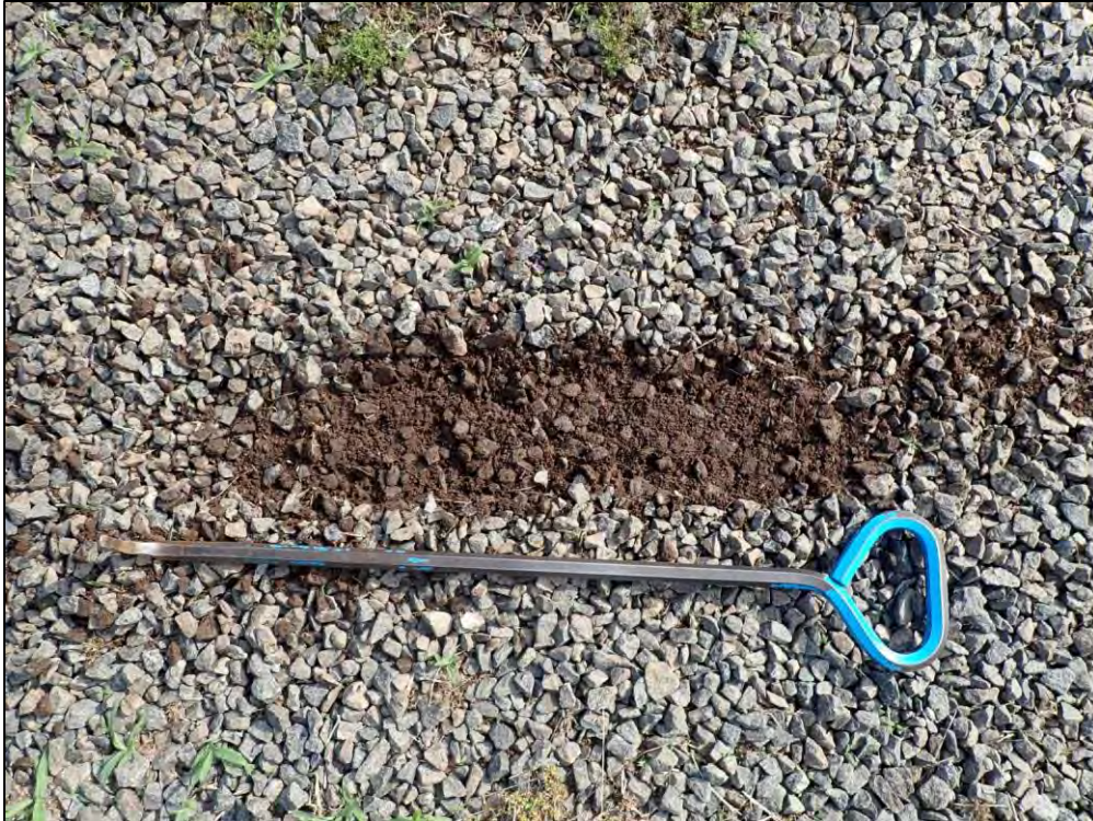
4584: Another close-up showing the Gravel Detail. Evidence of clogging (Immediate Repair Needed).
