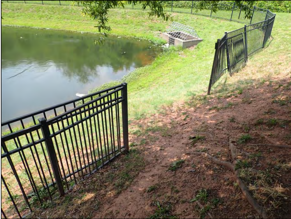
4768: Access, Overall. Fence is damaged (Routine Maintenance Needed).
