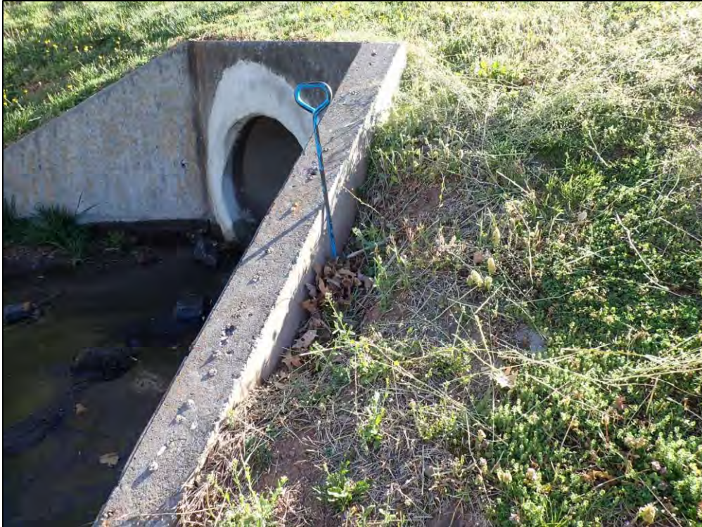
9323: Inflow Structure D5, overall. Evidence of erosion or undermining around inlet (Routine Maintenance Needed).
