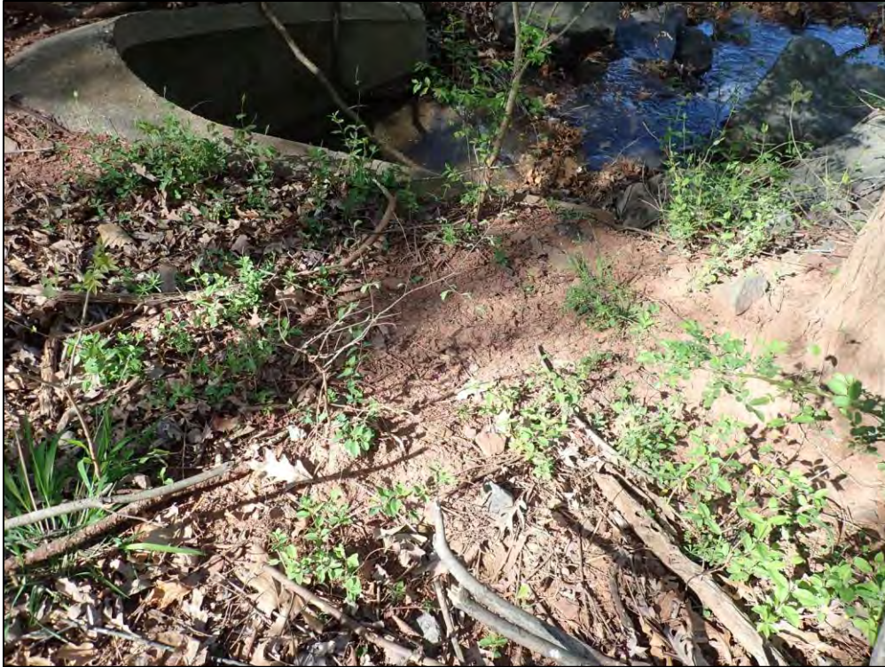
9375: Inflow Structure D1, closeup. Woody growth around the inlet structure (Routine Maintenance Needed).
