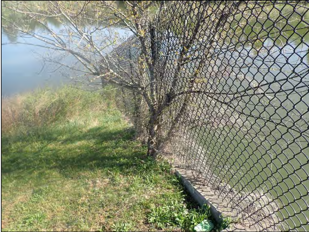
2737: Dam, closeup. Woody vegetation on the embankment (Routine Maintenance Needed).
