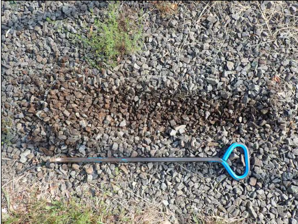
4588: Another close-up showing the Gravel Detail. Evidence of clogging (Immediate Repair Needed).
