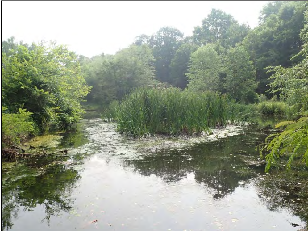
4967: Forebay Overall. Vegetation does not match the original design (Routine Maintenance Needed).
