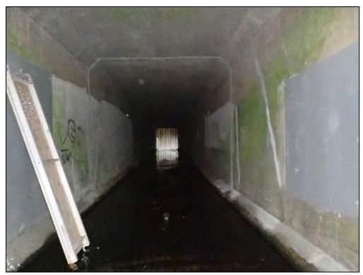
4361: Inside Control Str., looking downstream, middle pipe. Buildup of trash, debris, and sediment (Routine Maintenance Needed).
