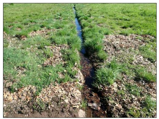
2880: Looking downstream along the Trickle Ditch toward Control Structure E-2. Low-flow ditch is clogged with sediment/debris (Routine Maintenance Needed).
