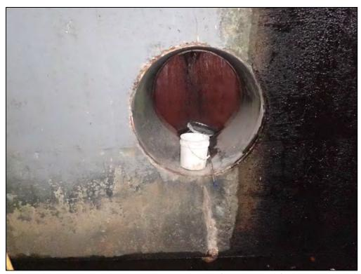
4352: Inside Control Str., looking toward dewatering valve orifice. Buildup of trash, debris, and sediment (Routine Maintenance Needed).
