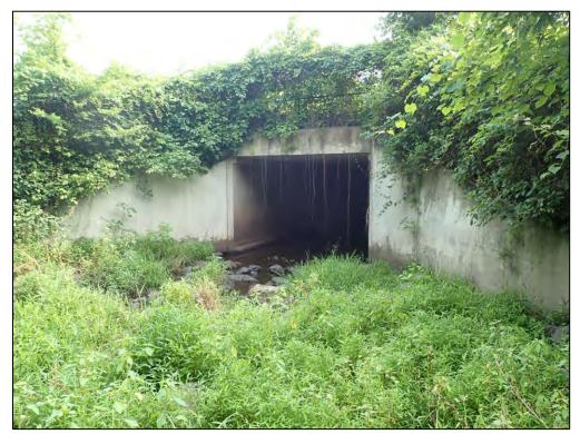
4943: Outfall Structure A, front. Woody vegetation growing within 5' of outlet and barrel (Routine Maintenance Needed).
