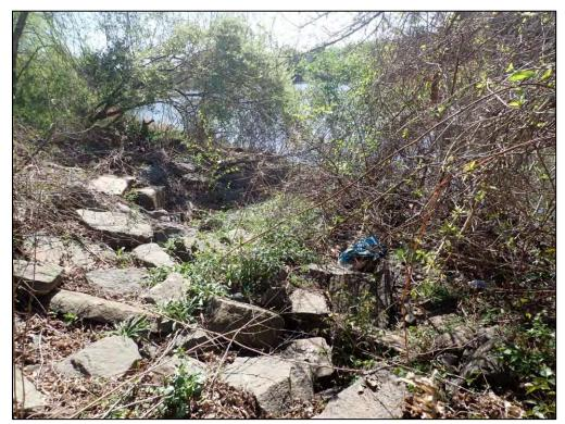
9573: From Inflow Structure EX. 19, looking downstream. Buildup of trash, debris, and sediment (Routine Maintenance Needed).
