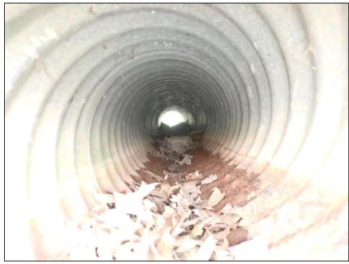
4631: Inside Inflow 1. Buildup of trash, debris, and sediment (Routine Maintenance Needed).
