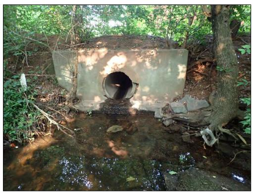
4900: Inflow Structure EX. EW-1, front. Woody growth around inlet structure (Routine Maintenance Needed).
