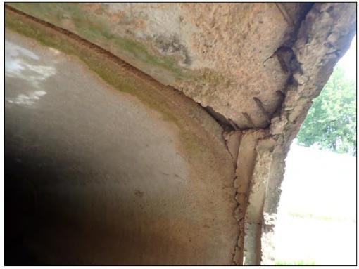
4690: Inflow Structure 1, closeup of the Middle Northern pipe. Damage to inlet pipe or structure, Spalling (Routine Maintenance Needed).
