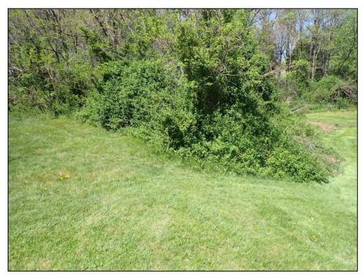
9429: Dam Overall. Woody vegetation on the embankment (Routine Maintenance Needed).
