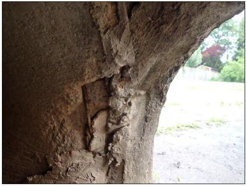
4686: Inflow Structure 1, closeup of the Middle Southern pipe. Damage to inlet pipe or structure, Spalling (Routine Maintenance Needed).
