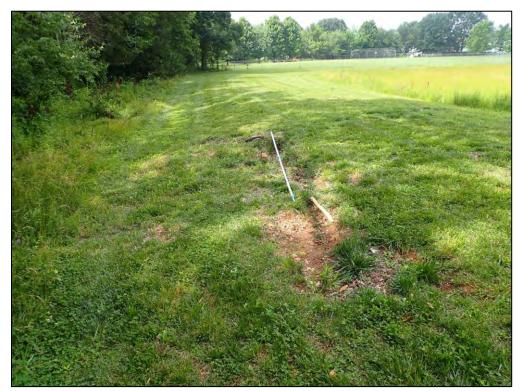
4720: Dam Overall. Signs of erosion, settlement, piping, or slope slippage (Routine Maintenance Needed).
