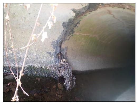
2884: Inflow 4, closeup. Woody growth around inlet structure (Routine Maintenance Needed).
