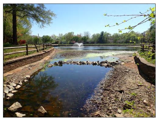
9502: Facility overall. Silt and sedimentation buildup (Routine Maintenance Needed).
