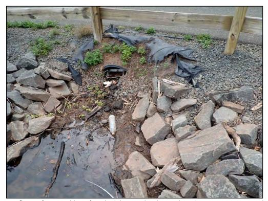
4384: Inflow 3, front. Buildup of trash, debris, and sediment (Routine Maintenance Needed).
