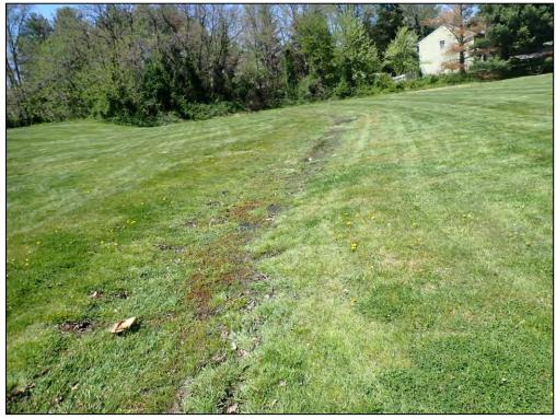
9443: Looking downstream along the Trickle Ditch toward Control Structure 1A. Low-flow ditch is clogged with sediment/debris (Routine Maintenance Needed).
