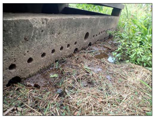
4610: Control Structure 21, low-flow orifices close-up. Sediment, debris, and vegetation accumulation. (Routine Maintenance Needed).
