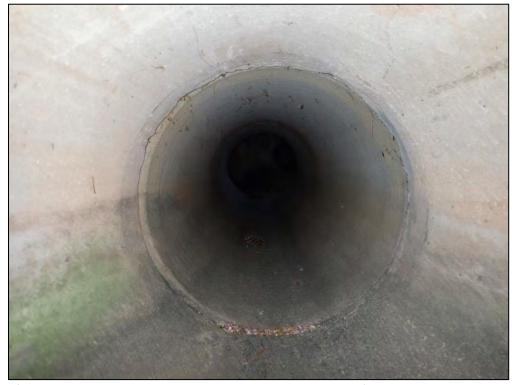
9594: Inflow 4. Damage to inlet pipe or structure, Joint separation (Routine Maintenance Needed).
