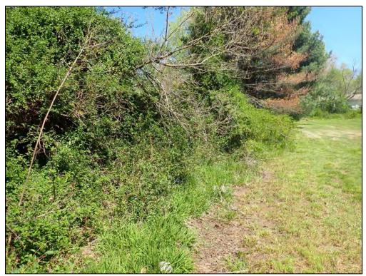
9434: Dam Overall. Woody vegetation on the embankment (Routine Maintenance Needed).
