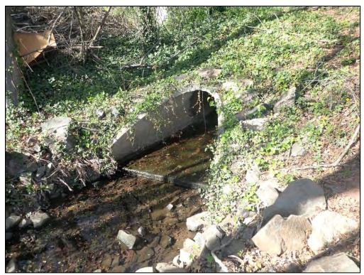
2881: Inflow 4, front. Woody growth around inlet structure (Routine Maintenance Needed).
