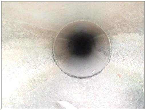
4670: Inside Inflow 9. Damage to inlet pipe or structure, Joint separation (Routine Maintenance Needed).
