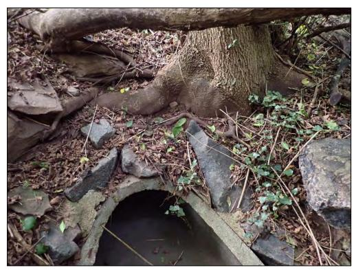
4908: Inflow Structure E-3, closeup. Woody growth around inlet structure (Routine Maintenance Needed).
