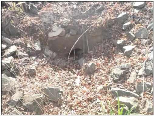
2885: Inflow E-3, front. Buildup of trash, debris, and sediment (Routine Maintenance Needed).
