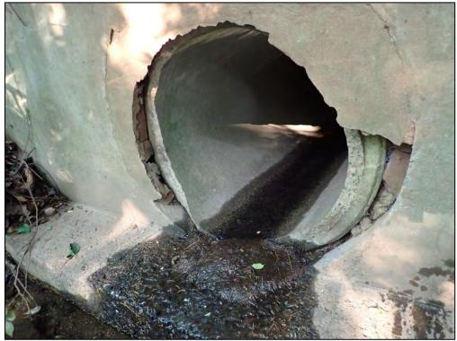
4901: Inflow Structure EX. EW-1, closeup. Damage to inlet pipe or structure, Spalling (Routine Maintenance Needed).
