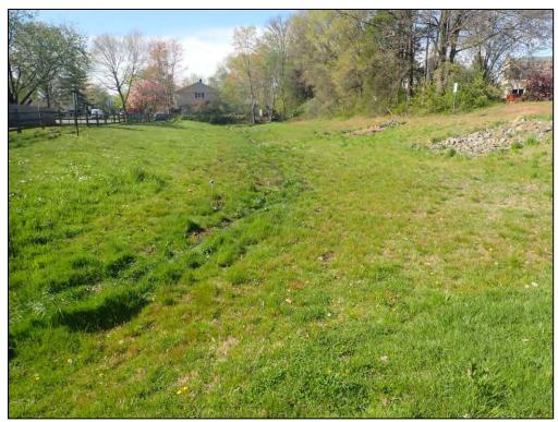
2867: Facility Overall. Low-flow ditch is clogged with sediment/debris (Routine Maintenance Needed).
