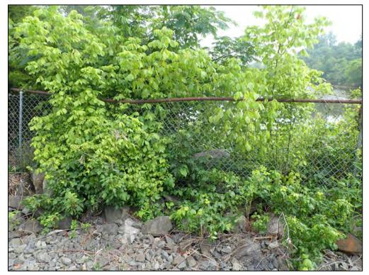
4857: From Emergency Spillway, looking upstream. Shrubbery, low growing vegetation, and/or vine material growing on embankment (Routine Maintenance Needed).
