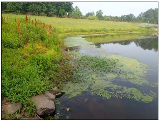
4956: Impoundment area, overall. The ponding area shows signs of poor health (i.e. nutrient overload, excess aquatic vegetation, or turbidity) (Monitor).
