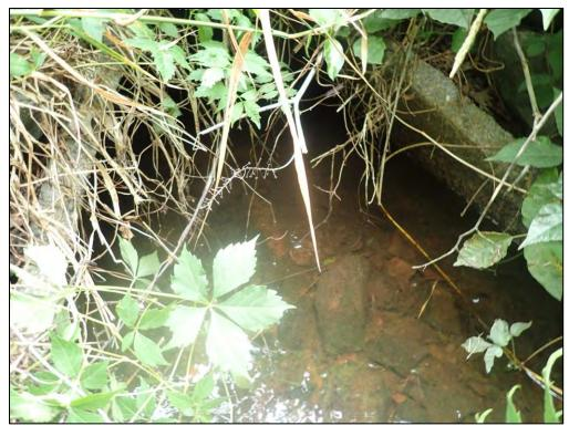
4715: Outfall Structure 22, closeup. Overgrown vegetation adjacent to the outfall (Routine Maintenance Needed).
