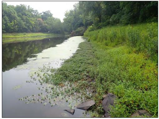
4955: Impoundment area, overall. The ponding area shows signs of poor health (i.e. nutrient overload, excess aquatic vegetation, or turbidity) (Monitor).
