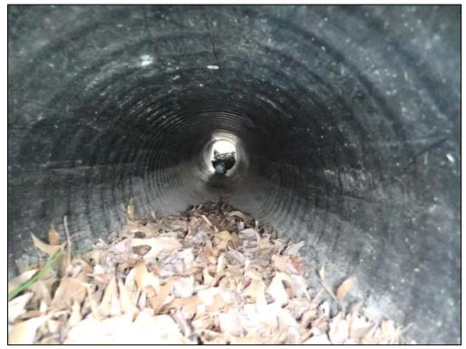
4640: Inside Inflow 3. Buildup of trash, debris, and sediment (Routine Maintenance Needed).
