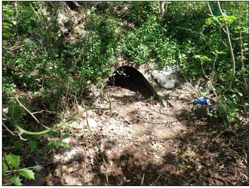
9439: Inflow Structure 11, front. Buildup of trash, debris, and sediment (Routine Maintenance Needed).
