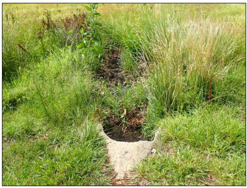
4665: From Inflow 8, looking downstream. Buildup of trash, debris, and sediment (Routine Maintenance Needed).
