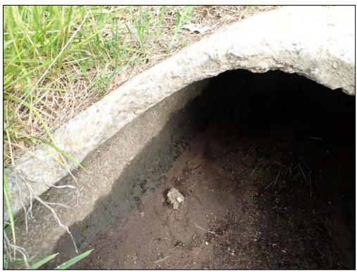
4663: Inflow 8, closeup. Damage to inlet pipe or structure, Spalling (Routine Maintenance Needed).
