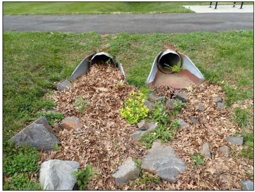
4633: Inflow 2, front. Buildup of trash, debris, and sediment (Routine Maintenance Needed).
