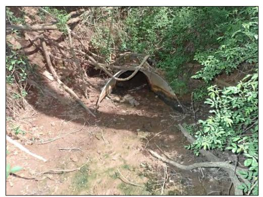
9430: Outfall Structure 1B, front. Buildup of trash, debris, and sediment around the outfall or in the channel (Routine Maintenance Needed).
