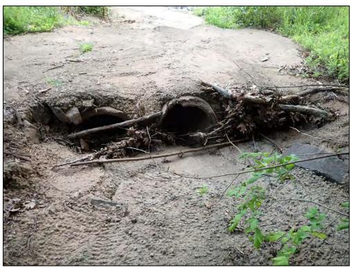
4954: Inflow 2, overall. Buildup of trash, debris, and sediment (Routine Maintenance Needed).
