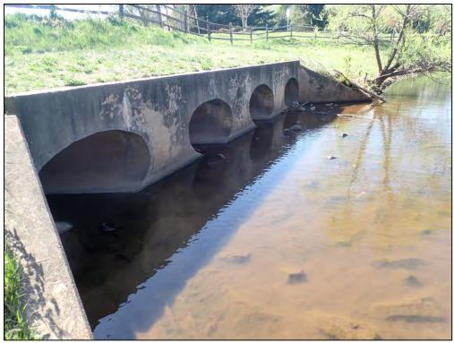
9603: Control Structure 1, front. Woody vegetation on the embankment (Routine Maintenance Needed).
