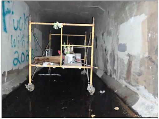
4360: Inside Control Str., looking downstream, North pipe. Buildup of trash, debris, and sediment (Routine Maintenance Needed).
