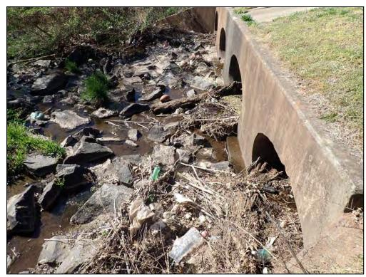
9617: Outfall Structure 2, front. Buildup of trash, debris, and sediment around the outfall or in the channel (Routine Maintenance Needed).
