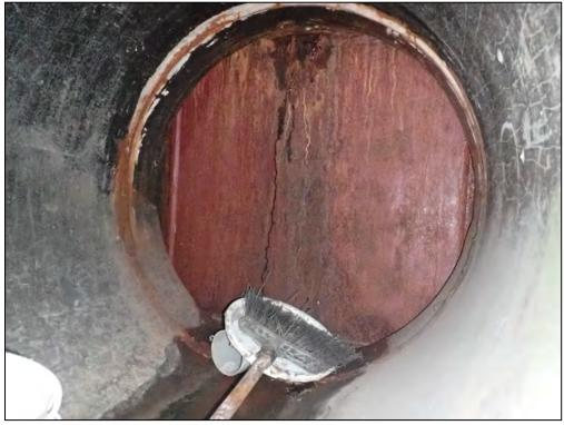
4355: Inside Control Str., closeup of dewatering valve orifice. Buildup of trash, debris, and sediment (Routine Maintenance Needed).
