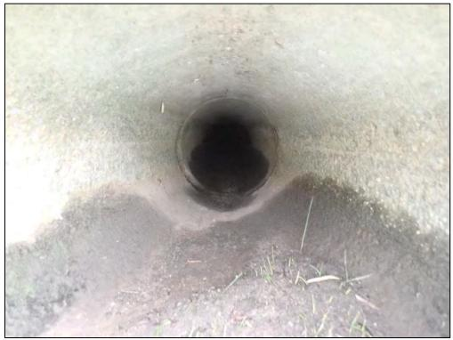
4664: Inside Inflow 8. Damage to inlet pipe or structure, Joint separation (Routine Maintenance Needed).
