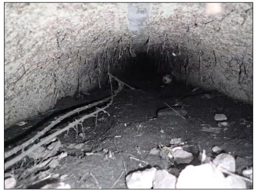
4891: Inside Inflow 1. Buildup of trash, debris, and sediment (Immediate Repair Needed).
