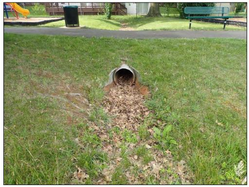
4630: Inflow 1, front. Buildup of trash, debris, and sediment (Routine Maintenance Needed).
