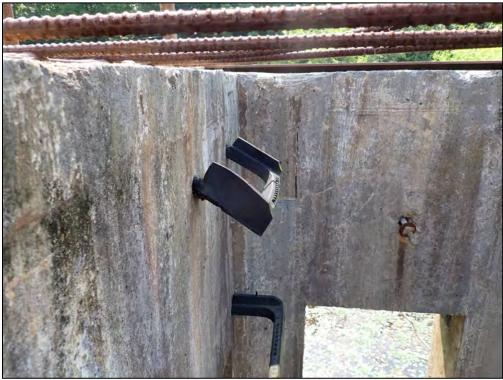
4839: Inside Control Str., closeup. BMP device is deteriorated, misaligned, and/or damaged (Immediate Repair Needed)
