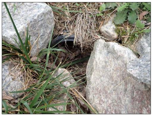
4645: Inflow 4, closeup. Buildup of trash, debris, and sediment (Routine Maintenance Needed).
