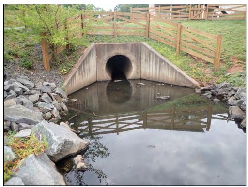
4391: Inflow 4, front. Woody growth around inlet structure (Routine Maintenance Needed).
