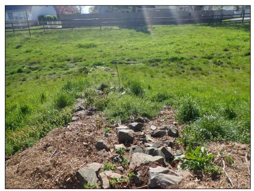
2874: From Inflow 2, looking downstream. Buildup of trash, debris, and sediment (Routine Maintenance Needed).
