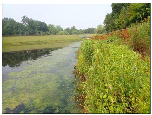
4922: Impoundment area, Overall. The ponding area shows signs of poor health (i.e. nutrient overload, excess aquatic vegetation, or turbidity) (Monitor).
