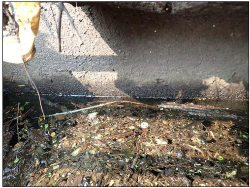
4927: Control Structure B, inside the trash rack. Trash, debris, or other material in BMP device (Routine Maintenance Needed).
