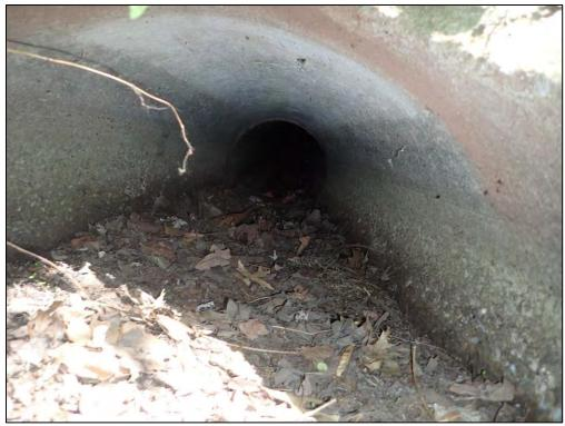
9440: Inside Inflow Structure 11. Joint Misalignment (Routine Maintenance Needed)
