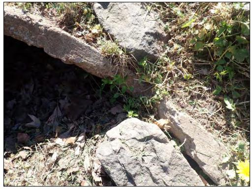
9437: Inflow 1, closeup. Damage to inlet pipe or structure (Routine Maintenance Needed).
