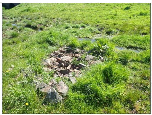
2877: From Inflow 3, looking downstream. Buildup of trash, debris, and sediment (Routine Maintenance Needed).
