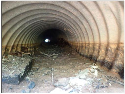
9431: Outfall Structure 1B, inside. Buildup of trash, debris, and sediment around the outfall or in the channel (Routine Maintenance Needed).
