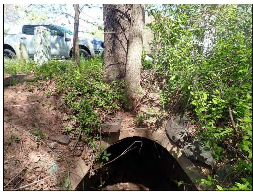
9448: Inflow 3, closeup. Woody growth around inlet structure (Routine Maintenance Needed).
