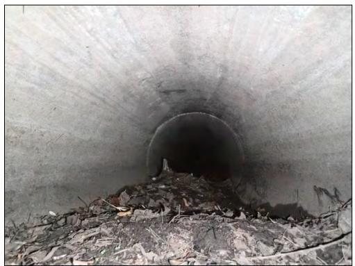
4380: Inside Inflow 2. Buildup of trash, debris, and sediment (Routine Maintenance Needed).
