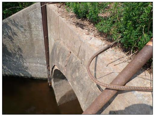
4828: Inflow 2, closeup. Damage to inlet pipe or structure, Spalling (Routine Maintenance Needed).
