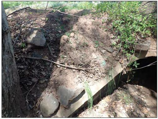
9447: Inflow 3, closeup. Evidence of erosion or undermining around the inlet (Routine Maintenance Needed).
