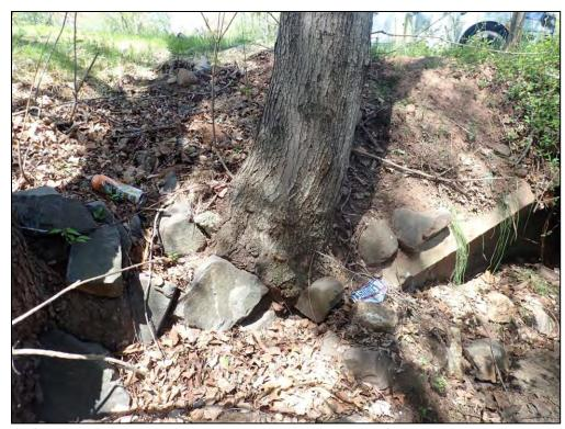
9450: Inflow 3, closeup. Woody growth around inlet structure (Routine Maintenance Needed).
