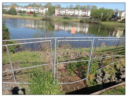
9602: From Inflow 5, looking downstream. Buildup of trash, debris, and sediment (Routine Maintenance Needed).
