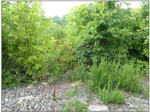
4859: From Emergency Spillway, looking downstream. Shrubbery, low growing vegetation, and/or vine material growing on embankment (Routine Maintenance Needed).
