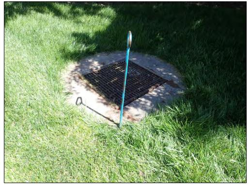
9411: Outfall Structure 54, overall. Signs of erosion around outfall or channel (Routine Maintenance Needed).
