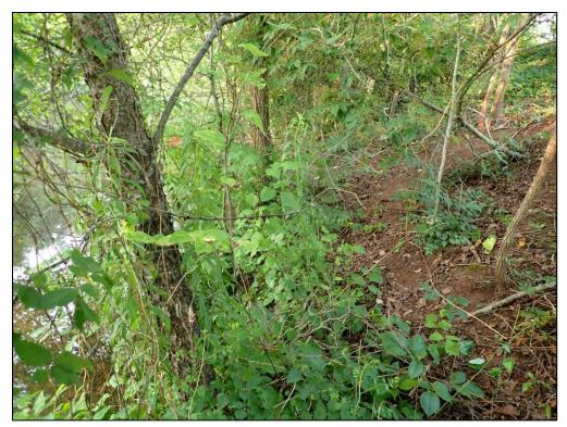
4896: Inflow Structure EX. ES-1, Overall. Woody growth around inlet structure (Routine Maintenance Needed).
