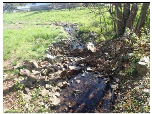
2883: From Inflow 4, looking downstream. Buildup of trash, debris, and sediment (Monitor).
