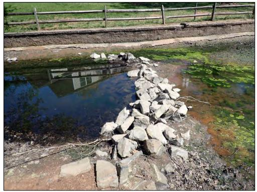
9505: Check Dam, closeup. Buildup of trash or debris (Routine Maintenance Needed).
