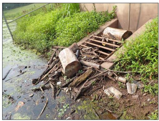
4926: Control Structure B, trash rack close-up. Trash, debris, or other material in BMP device (Routine Maintenance Needed).
