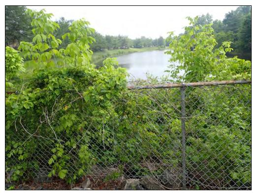
4856: From Emergency Spillway, looking upstream. Shrubbery, low growing vegetation, and/or vine material growing on embankment (Routine Maintenance Needed).
