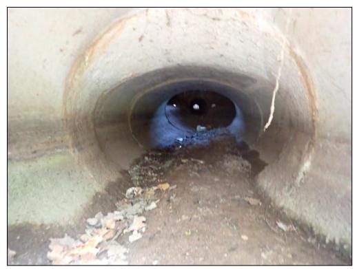
9446: Inside Inflow 3. Buildup of trash, debris, and sediment (Routine Maintenance Needed).
