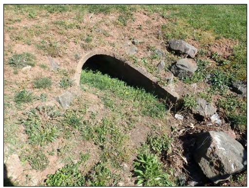
9631: Inflow Structure 9, front. Buildup of trash, debris, and sediment (Immediate Repair Needed).
