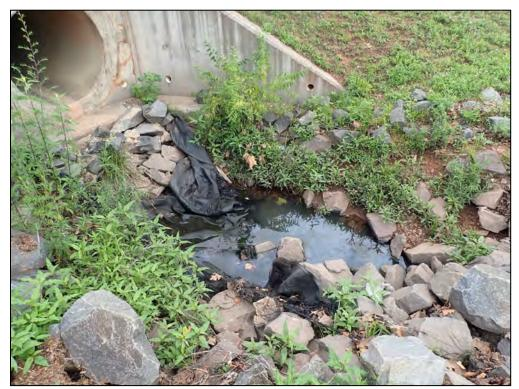
4420: Inflow 9, closeup. Evidence of erosion or undermining around inlet (Routine Maintenance Needed).
