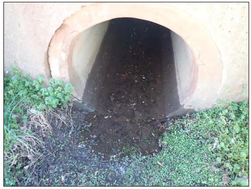
9600: Inflow 5, closeup. Damage to inlet pipe or structure (Monitor).
