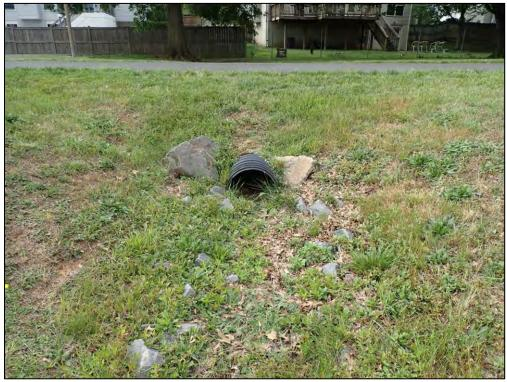
4639: Inflow 3, front. Buildup of trash, debris, and sediment (Routine Maintenance Needed).
