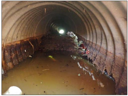
9421: Control Structure 1A, inside. Trash, debris, or other material in BMP device (Immediate Repair Needed). Extreme Invert Erosion Observed (Immediate Repair Needed).
