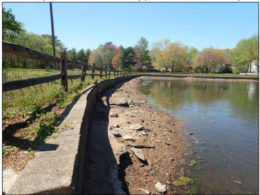
9484: Impoundment area, Sediment 2 overall. Buildup of trash and debris (Routine Maintenance Needed). Silt and sedimentation buildup (Routine Maintenance Needed).
