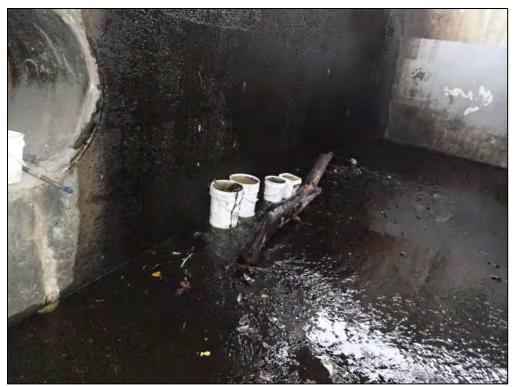
4357: Inside Control Str., Buildup of trash, debris, and sediment (Routine Maintenance Needed).
