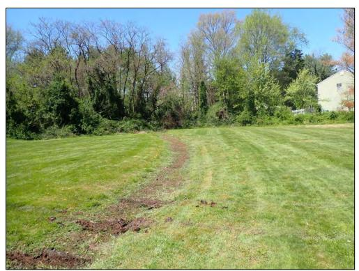
9444: Looking downstream along the Trickle Ditch toward Control Structure 1A. Low-flow ditch is clogged with sediment/debris (Routine Maintenance Needed).
