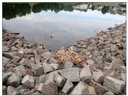
4381: From Inflow 2, looking downstream. Buildup of trash, debris, and sediment (Routine Maintenance Needed).
