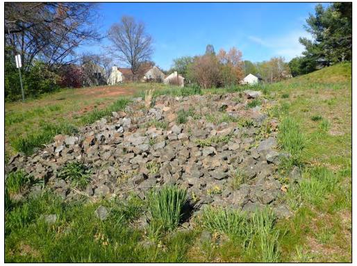
2868: Looking upstream along Inflow 1. Buildup of trash, debris, and sediment (Routine Maintenance Needed).
