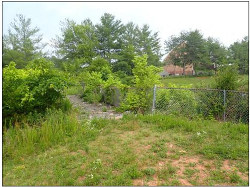
4855: Emergency Spillway, overall. Shrubbery, low growing vegetation, and/or vine material growing on embankment (Routine Maintenance Needed).
