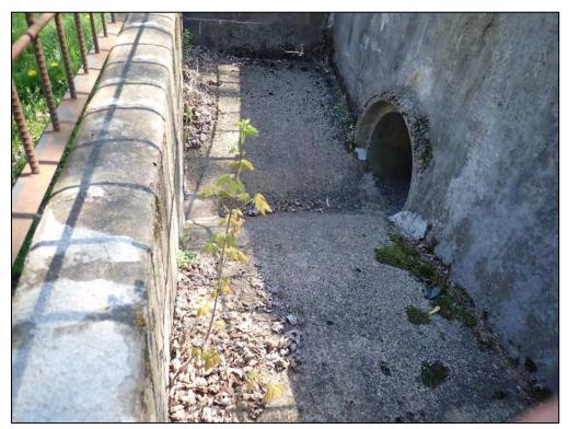
9391: Inside Control Structure 16. Trash, debris, or other material in BMP device (Routine Maintenance Needed).
