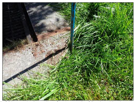
9412: Outfall Structure 54, closeup. Signs of erosion around outfall or channel (Routine Maintenance Needed).
