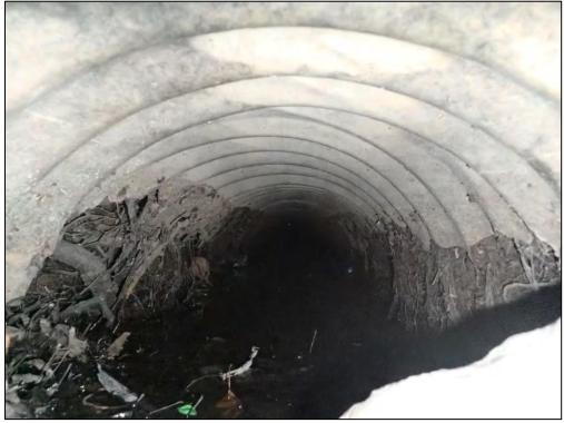
2886: Inside Inflow E-3. Damage to inlet pipe or structure (Immediate Repair Needed).
