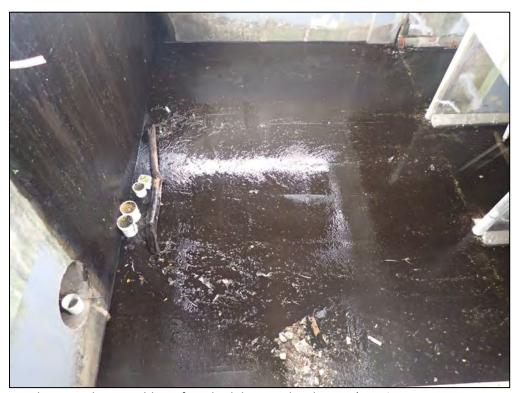
4358: Inside Control Str., Buildup of trash, debris, and sediment (Routine Maintenance Needed).
