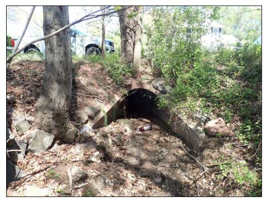
9445: Inflow 3, front. Woody growth around inlet structure (Routine Maintenance Needed). Buildup of trash, debris, and sediment (Routine Maintenance Needed).
