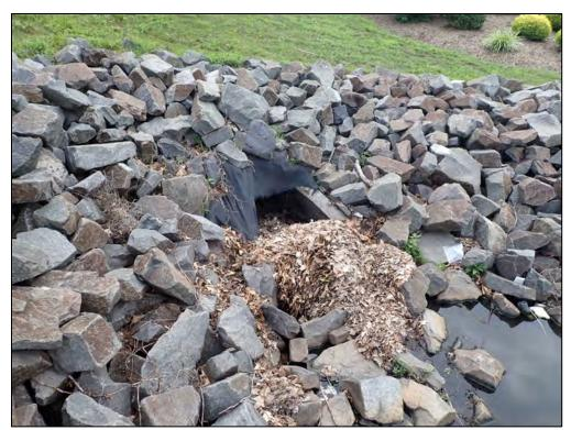
4379: Inflow 2, front. Buildup of trash, debris, and sediment (Routine Maintenance Needed).
