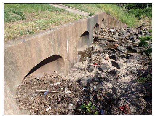
9612: Outfall Structure 2, front. Buildup of trash, debris, and sediment around the outfall or in the channel (Routine Maintenance Needed).
