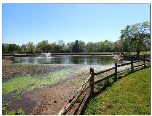
9507: Facility overall. Silt and sedimentation buildup (Routine Maintenance Needed).
