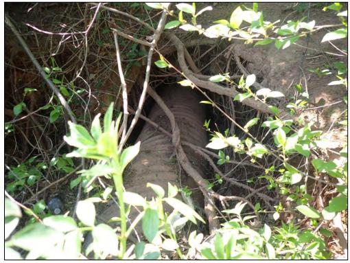
9423: Control Structure 1A, closeup. Signs of erosion, settlement, piping, or slope slippage (Immediate Repair Needed).
