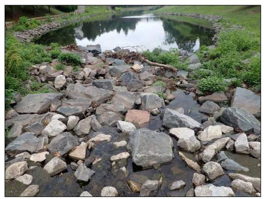
4396: From Inflow 5, looking downstream. Buildup of trash, debris, and sediment (Routine Maintenance Needed).
