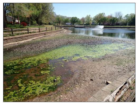
9508: Impoundment area, Sediment 3 overall. Silt and sedimentation buildup (Routine Maintenance Needed).
