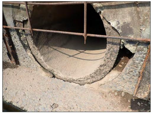
4875: Inflow 6, closeup. Damage to inlet pipe or structure (Routine Maintenance Needed).
