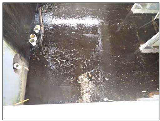
4359: Inside Control Str., Buildup of trash, debris, and sediment (Routine Maintenance Needed).
